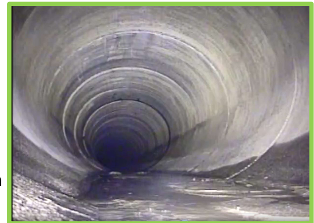
Figure 1 Plant 3 Outfall Storm Main Inspection Summary
