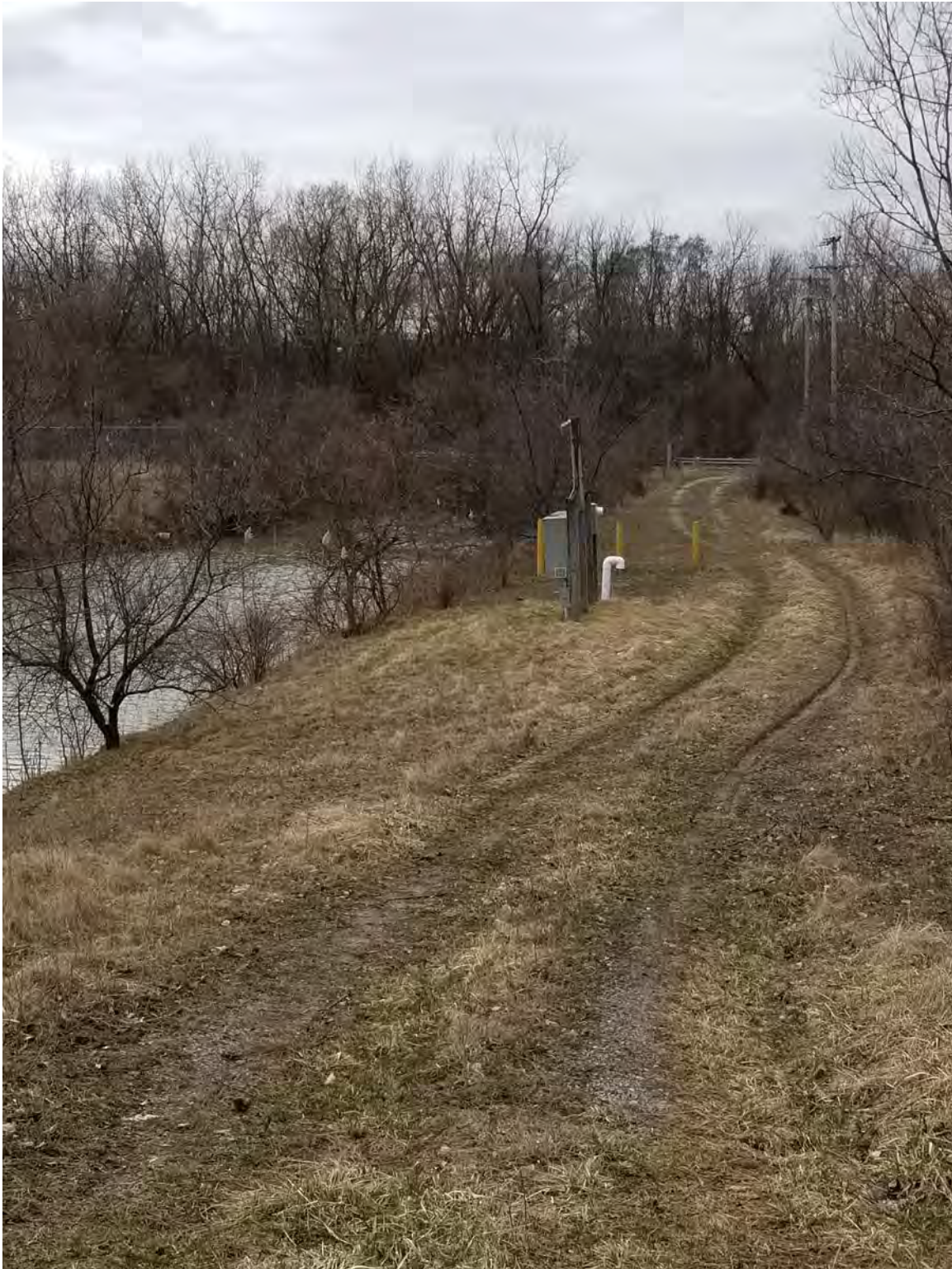
Photo 1 – View of Gauge Drain and electrical panel for pump station for Crow Island Landfill , west towards the Saginaw River 04-11-2019
