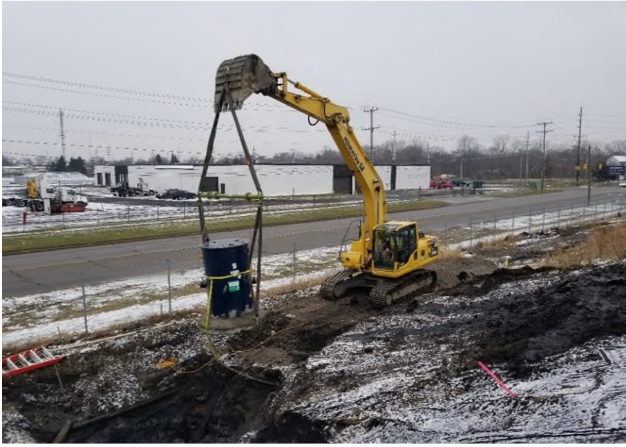
11/30/18 - Sump structure placed in excavation level and at grade.
