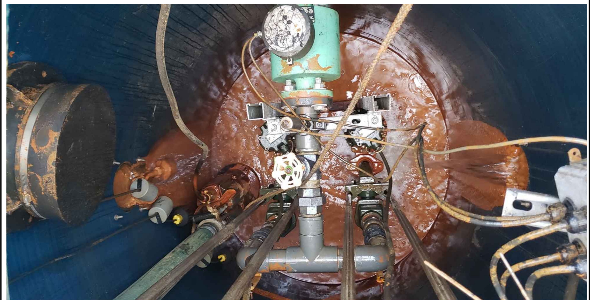
1/16/19 - Inside of Dewatering sump.
