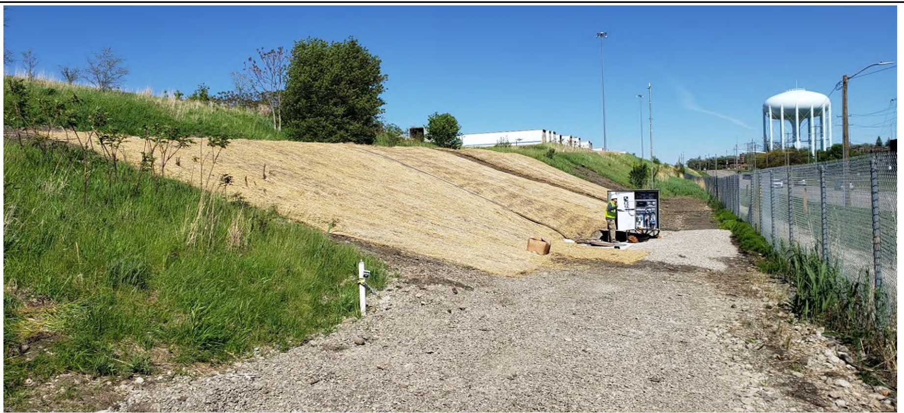
05/23/19 - Injection panel with straw mat cover down.
