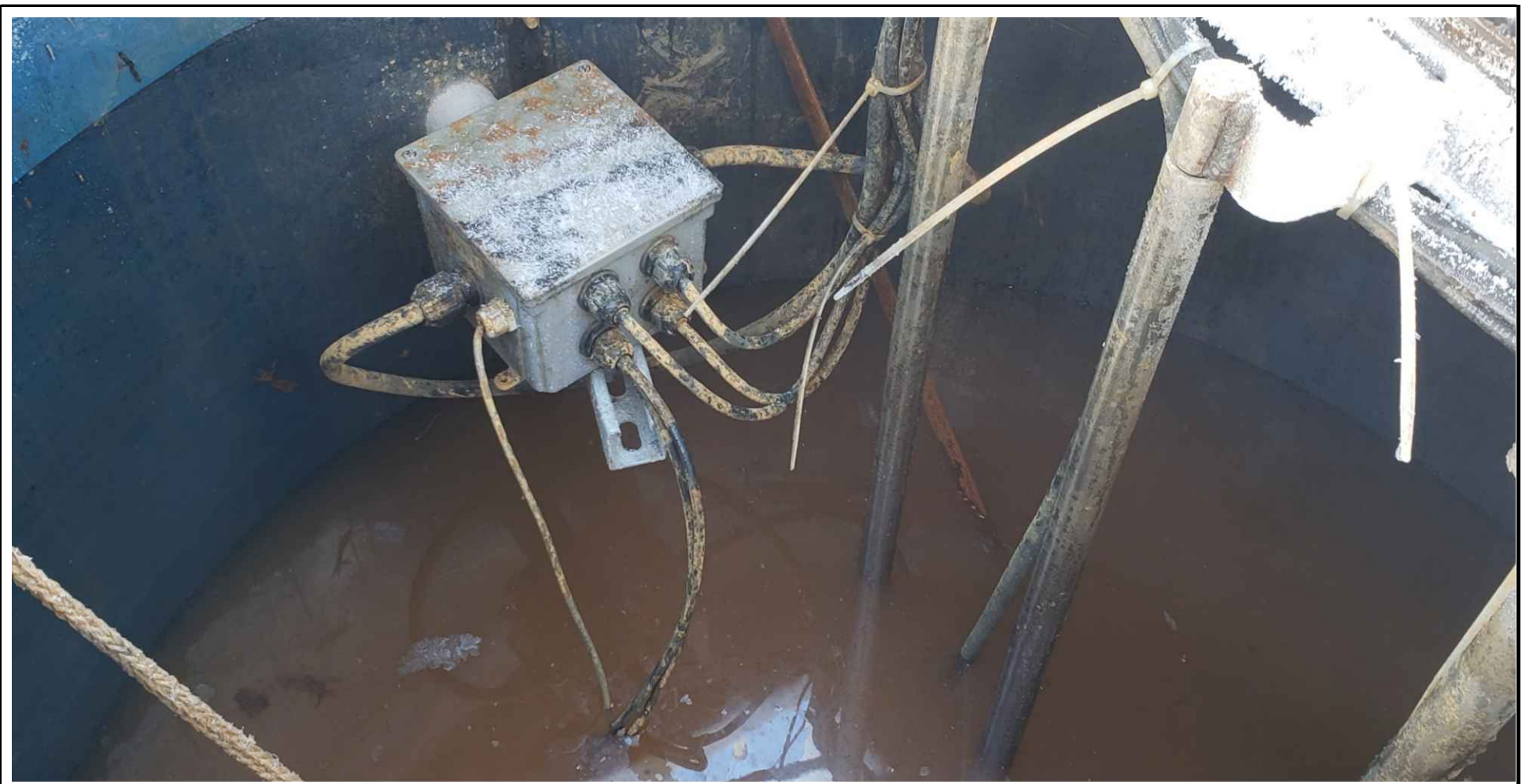
1/21/19 - Sump filled with water.
