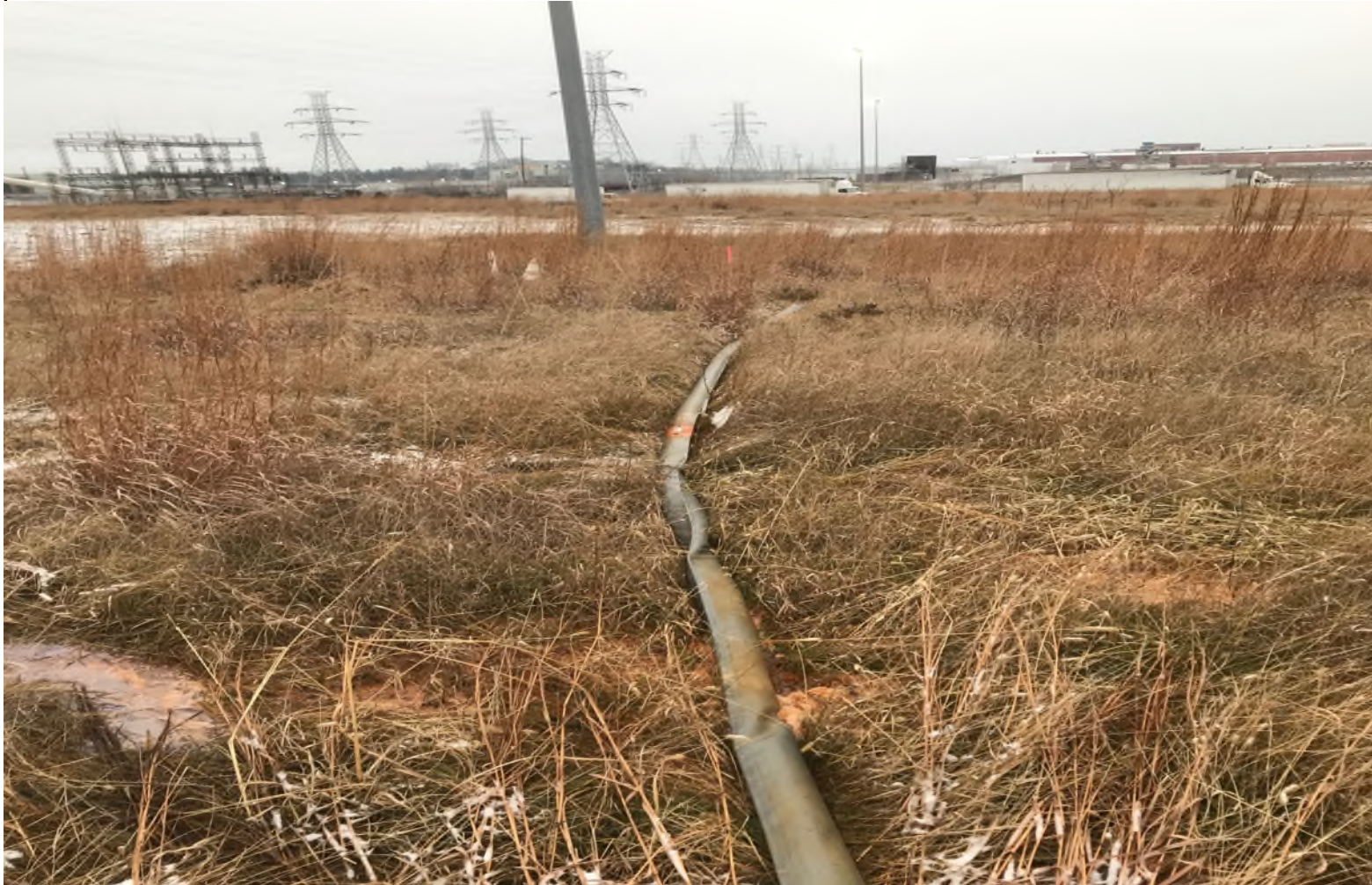
12/26/18 - Photo of dewatering pump discharge location in USPS west field.
