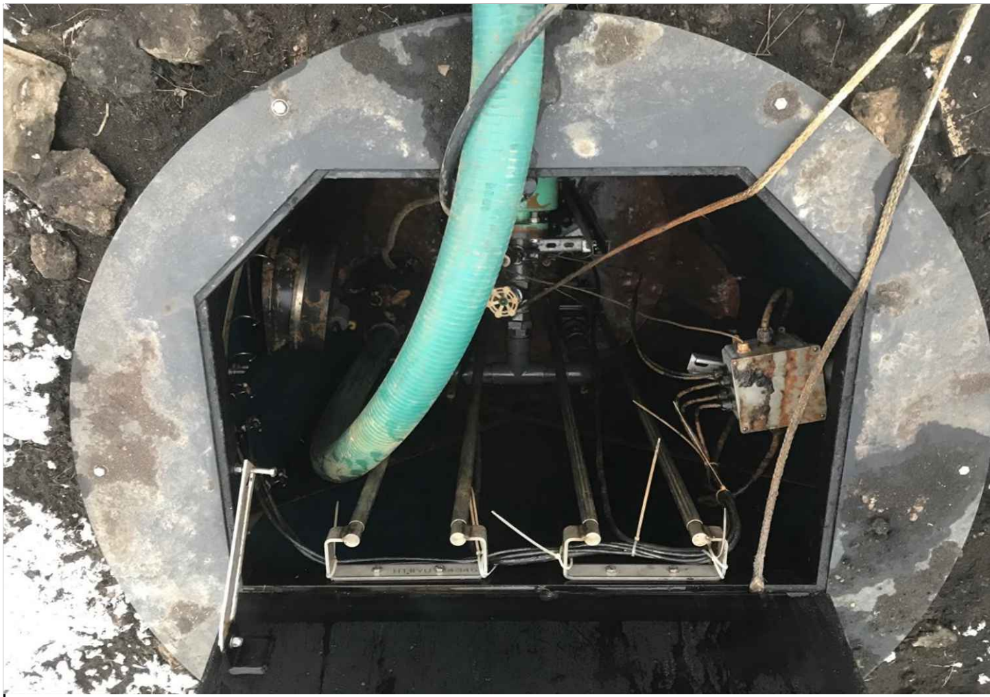
12/26/18 - Inside of Dewatering sump.
