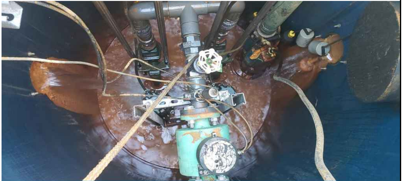
1/4/19 - Inside of Dewatering sump.
