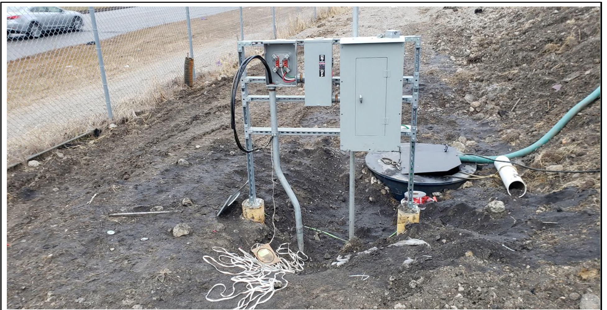
1/16/19 - Wire pulled to meter from pole.
