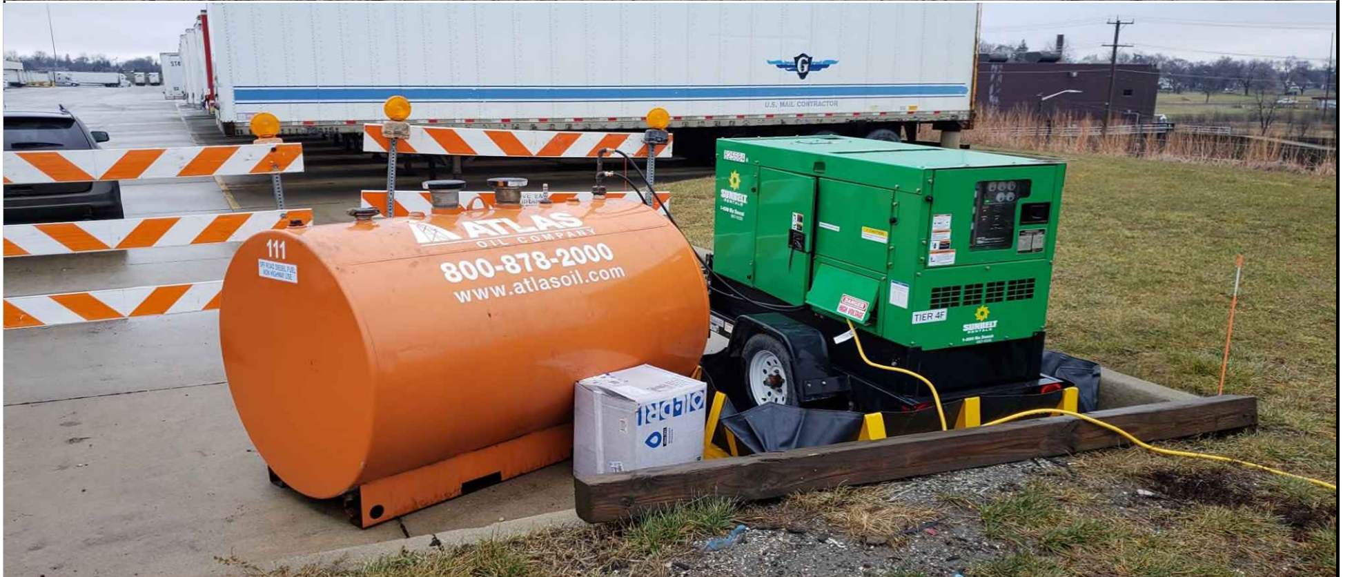
12/21/18 - Photo of dewatering pump generator and fuel tank.
