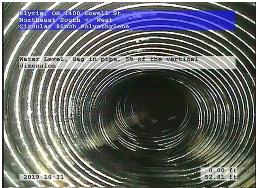
Northeast South-West_bdfccd14-7ccc-4f71-950a-f52a4c11683f_20191031_113611_977.jpg, 00:04:59, 52.81ft Water Level, Sag in pipe, 5% of the vertical dimension
