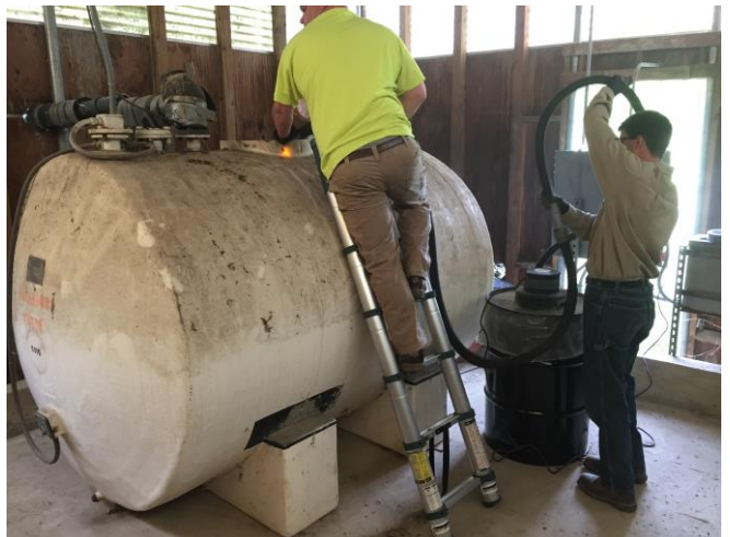
Photo #4: EMS removes liquids from AST
