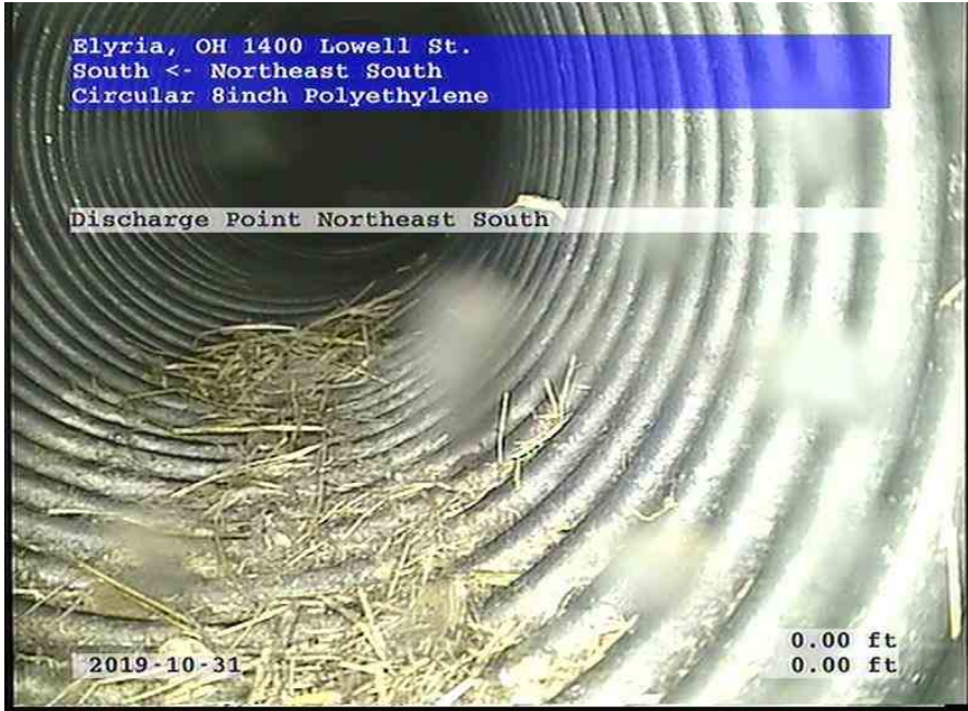
South-Northeast South_406ce8ba-2203-49f8-8e1b-991e7a9781ac_20191031_095500_247.jpg, 00:00:00, 0.00ft Discharge Point
