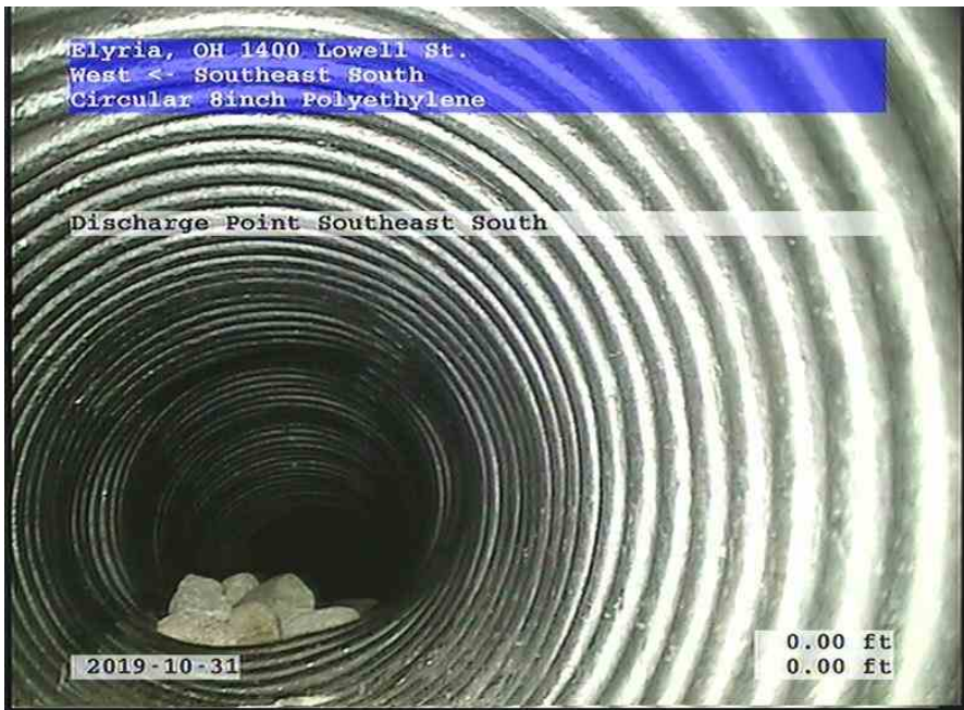
West-Southeast South_48dce329-3f1d-46e8-8c1b-5b46760ac551_20191031_105906_665.jpg, 00:00:00, 0.00ft Discharge Point
