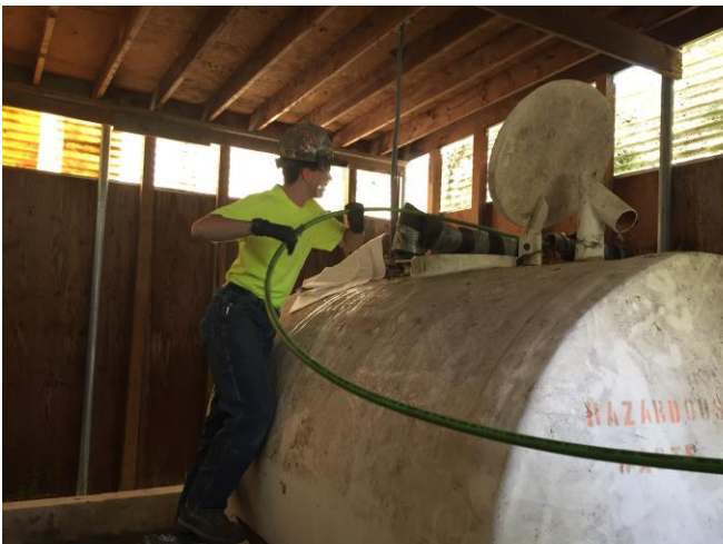
Photo #5: EMS Power washing interior of AST
