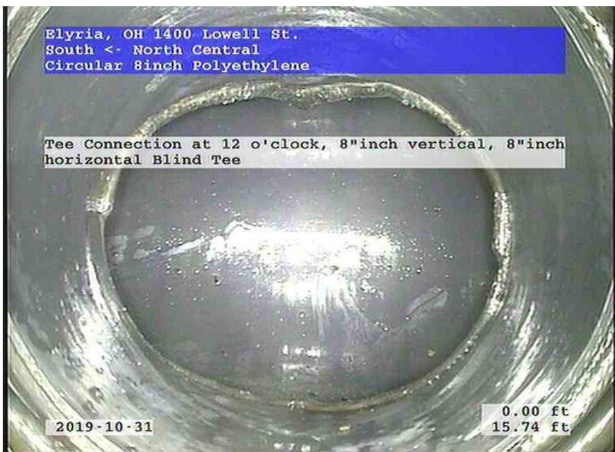
South-North Central_06741066-205a-465b-8f09-2f74ef4eb135_20191031_153315_767.jpg, 00:00:50, 15.74ft Tee Connection at 12 o'clock, 8"inch vertical, 8"inch horizontal
