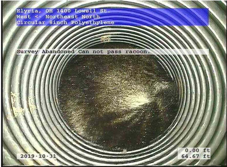
West-Northeast North_019c96a4-564a-49cf-ab16-098a7b071397_20191031_093956_600.jpg, 00:07:00, 64.67ft Survey Abandoned
