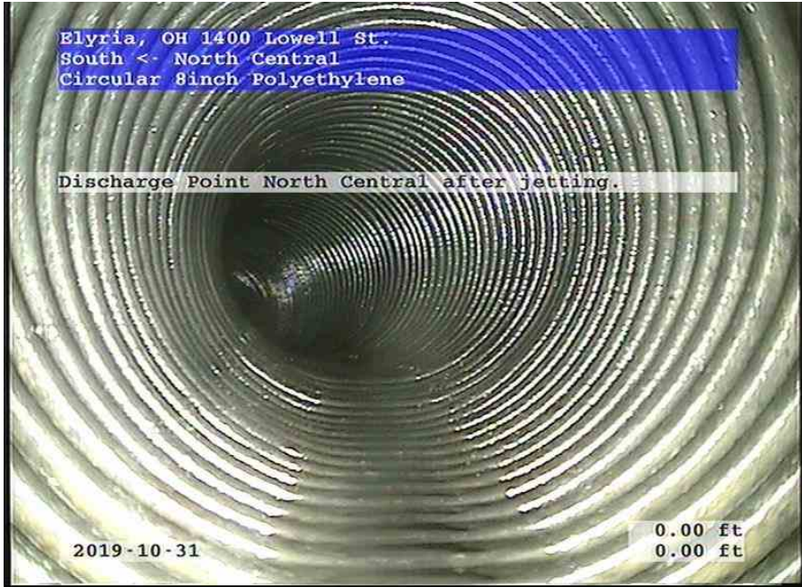
South-North Central_8dc7d76d-a76e-466f-a145-517f92d6a92d_20191031_153154_760.jpg, 00:00:00, 0.00ft Discharge Point
