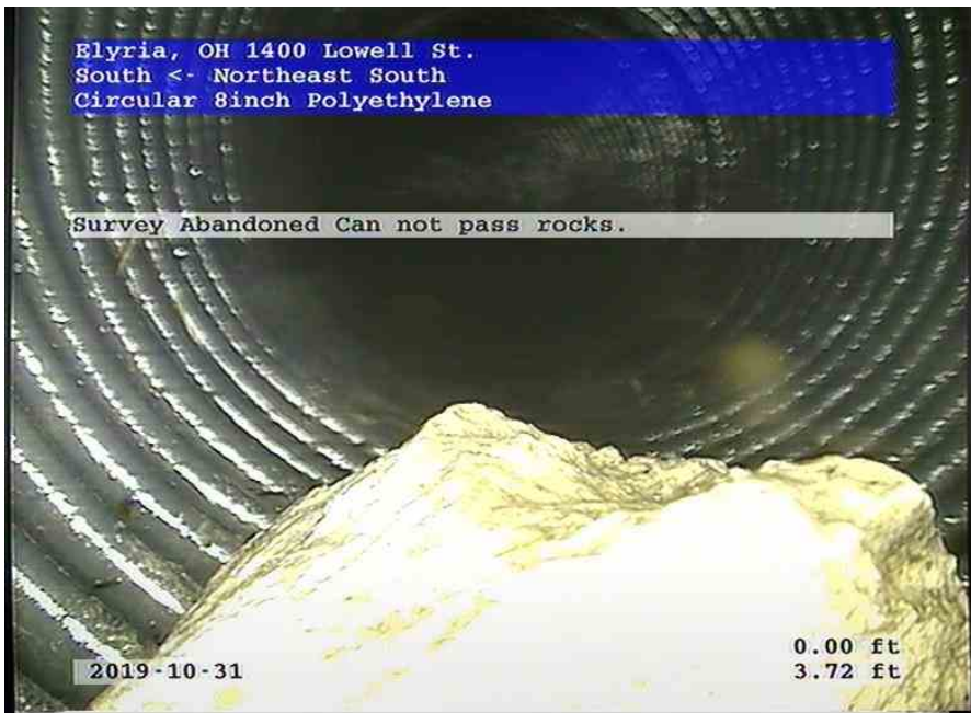
South-Northeast South_de225c83-cf7a-408c-8adc-360815883731_20191031_102206_004.jpg, 00:00:54, 3.72ft Survey Abandoned
