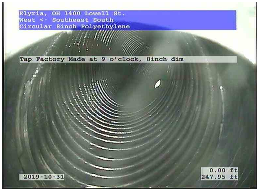
West-Southeast South_49aff70b-8ae0-48a3-94c9-8be63afd766d_20191031_141221_220.jpg, 00:10:19, 247.95ft Tap Factory Made at 9 o'clock, 8inch dim
