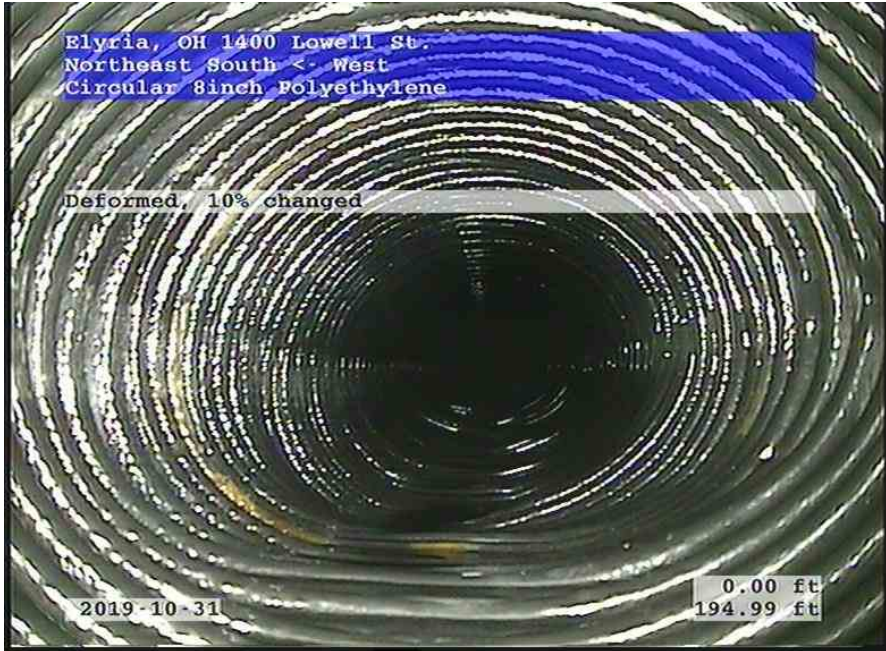
Northeast South-West_b9c4ef06-2f18-43e8-8cd0-aba396c9e2c9_20191031_120419_104.jpg, 00:12:18, 194.99ft Deformed, 10% changed
