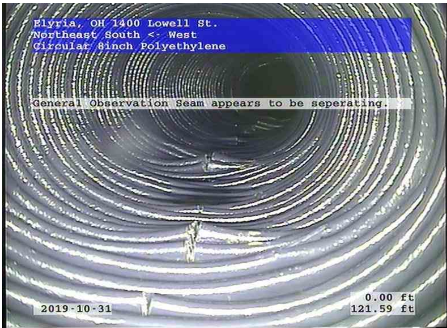
Northeast South-West_805729f6-6de5-4d77-813e-1ce6491aae7e_20191031_120054_791.jpg, 00:09:26, 121.59ft General Observation
