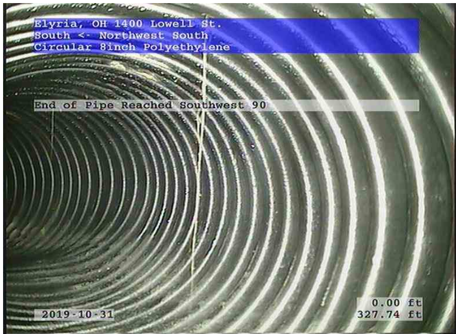
South-Northwest South_e19ea4a1-15b1-40a0-857b-e148e82df634_20191031_163821_498.jpg, 00:07:15, 327.74ft End of Pipe
