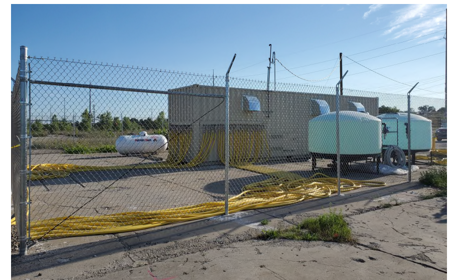
Plant 2 Biosparging Unit and Nutrient Injection Tanks
