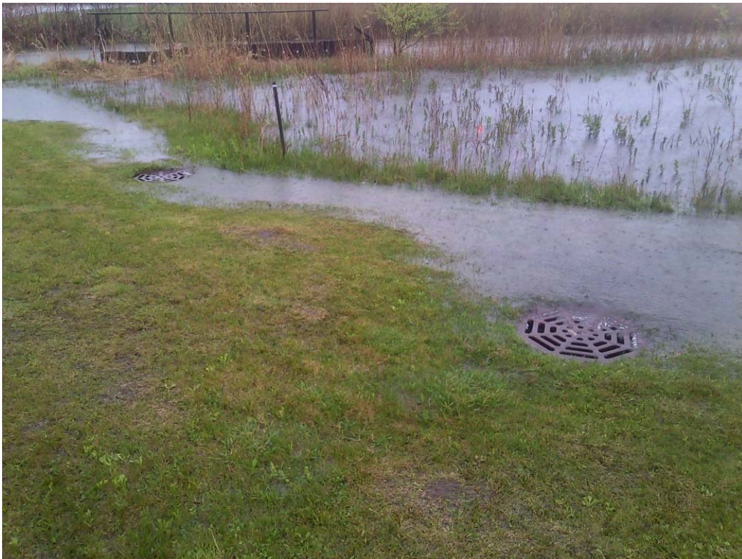
PHOTO 8: NORTH DITCH – OUTFALL 22 DISCHARGE LOCATIONS (5/2014)
