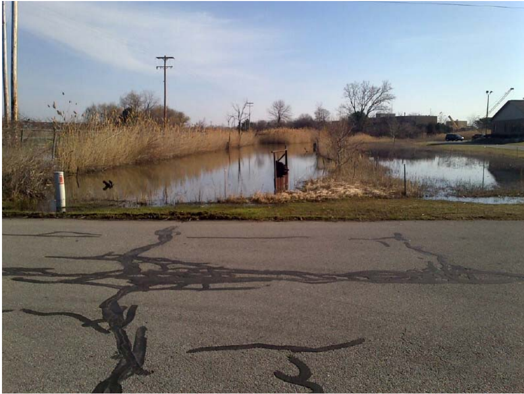
PHOTO 1: NORTH DITCH - LOOKING NORTHEAST FROM DRIVEWAY (4/2013)
