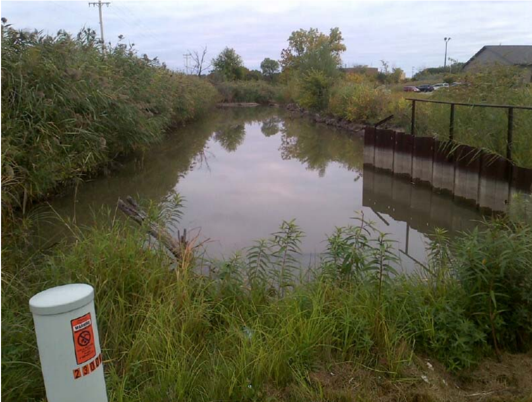
PHOTO 7: NORTH DITCH - LOOKING NORTHEAST FROM DRIVEWAY (9/2013)
