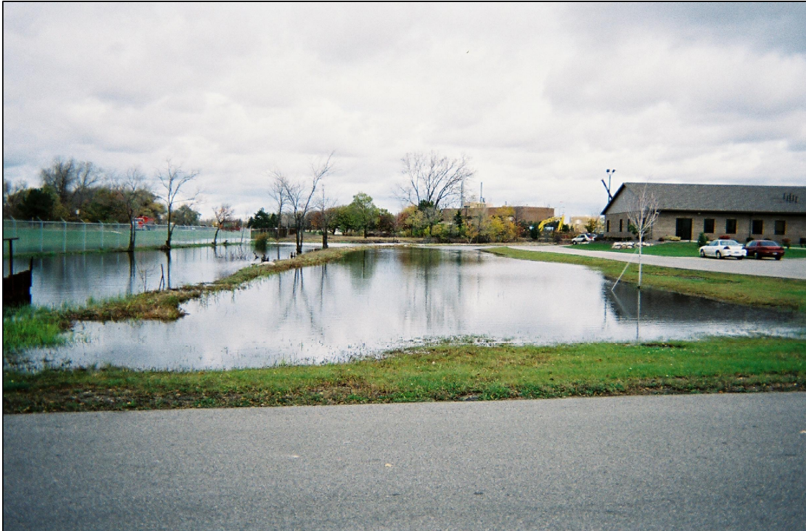
NORTH DITCH AFTER RAINFALL EVENT - FALL 2006. PHOTOGRAPH TAKEN FROM THE DRIVEWAY INTO THE SUPPLIER PARK OFF OF VETERANS MEMORIAL PARKWAY LOOKING TO THE NORTHEAST.
