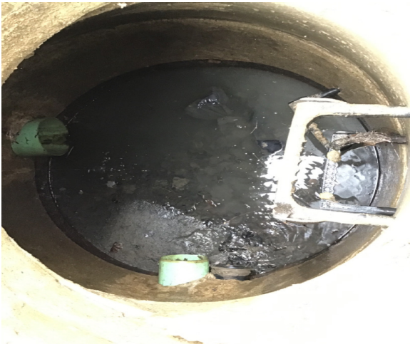
P2-MH-12 after pumping out. Facing north.
