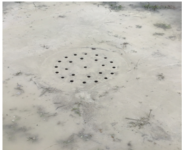
P2-MH-14 filled with flowable fill.
