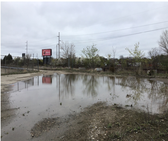
Ponded area between P2-MH-14 and bridge. Facing northeast.
