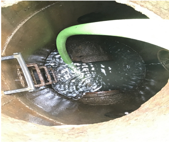
P2-MH-14 after pumping out. Facing north.
