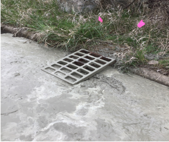
P2-MH-12 filled with concrete.
