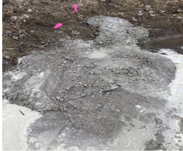
P2-MH-13 filled with concrete.
