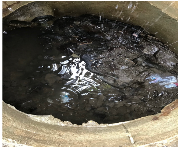
P2-MH-13 after pumping out. Facing north.
