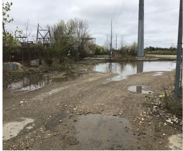
Ponded area between bridge and P2-MH-14. Taken from bridge facing south.
