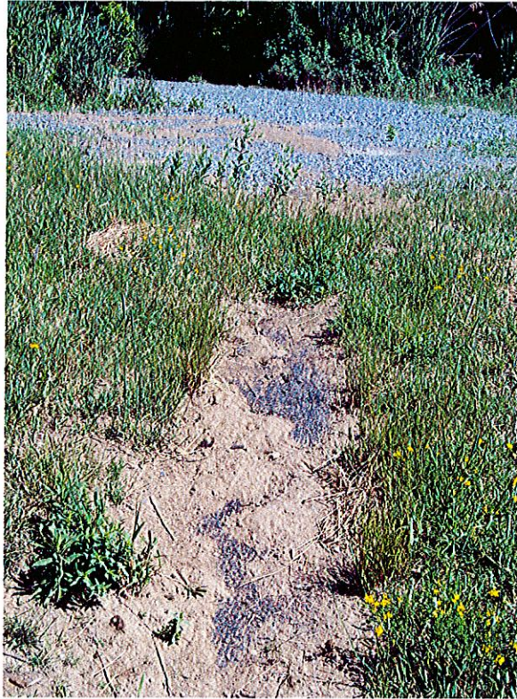
Photograph 7: View of eroded topsoil with visible erosion control fabric.
