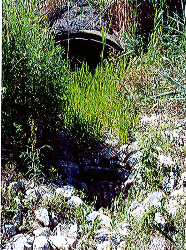
Photograph 1: View of CB-5/Outfall 004 spillway.
