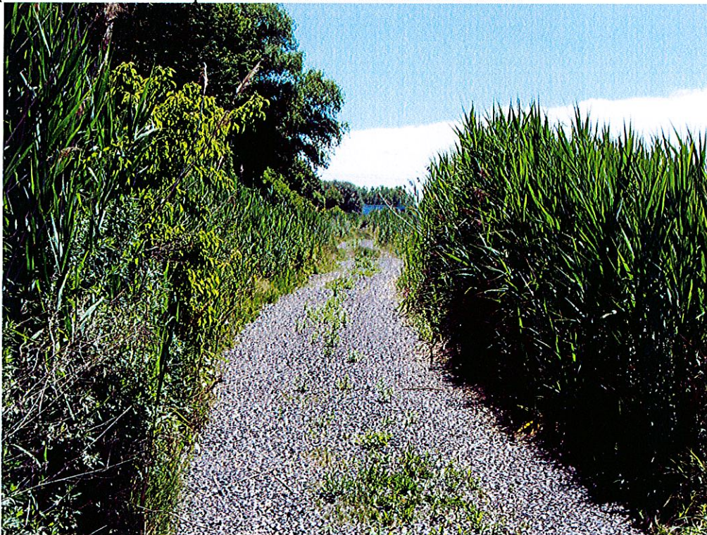
Photograph 8: View looking east from CB-3 outlet at repaired access road.
