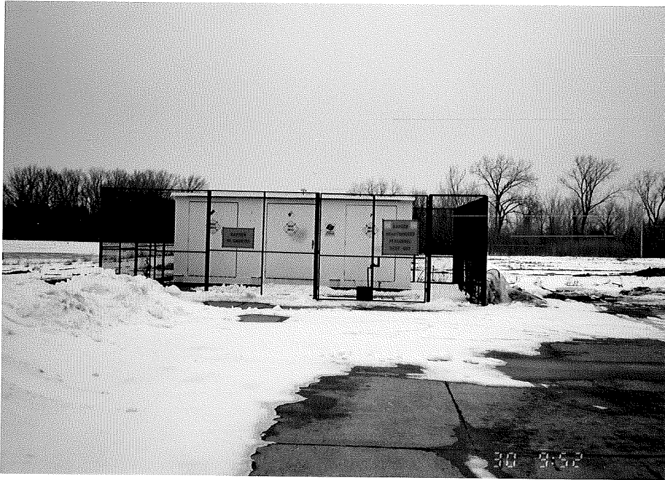
Photograph No. 3 Orientation: North Description: This photograph shows the HWSA shed.
