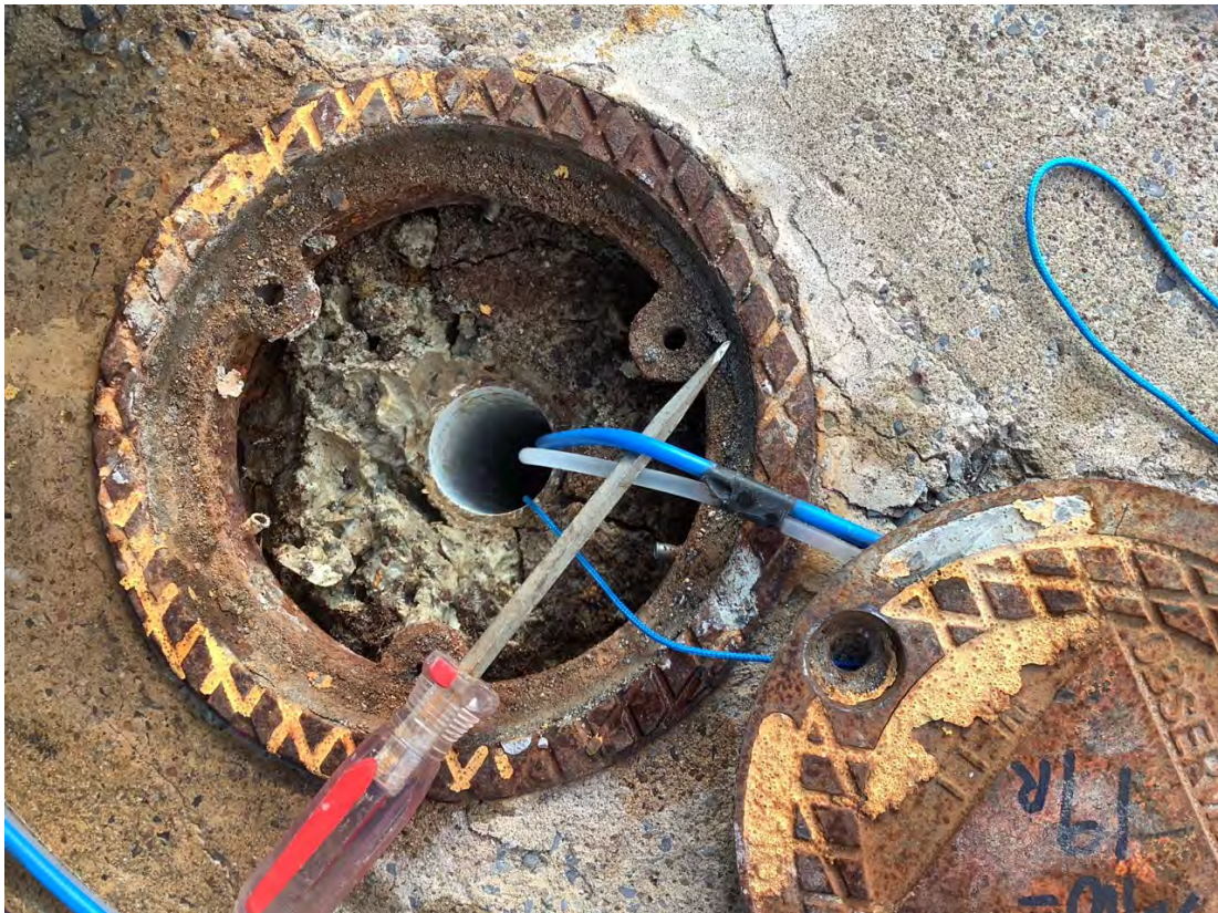
Photo 3: Grease/sludge around well casing
