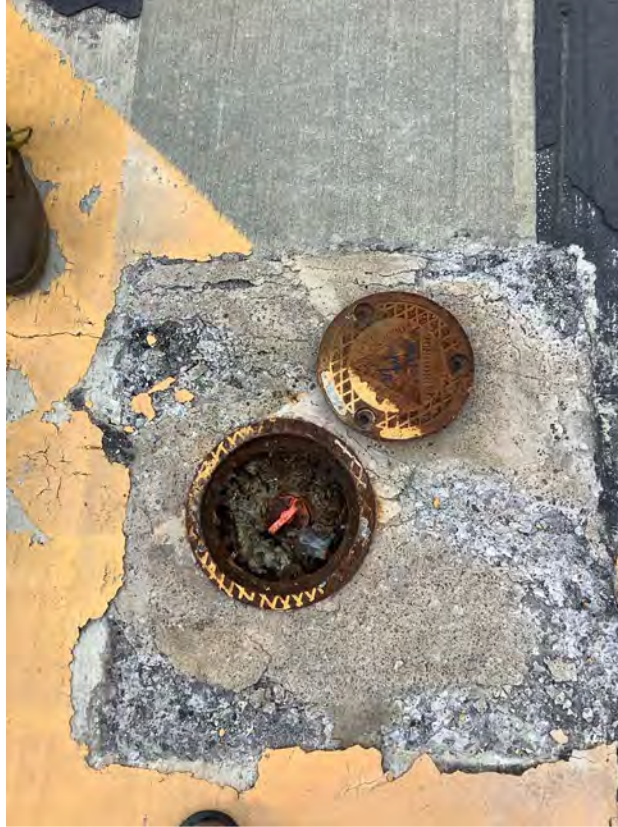
Photo 3: Grease/sludge around well casing
