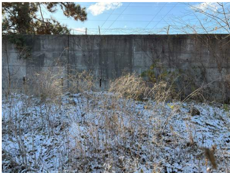
PP02, Facing South
