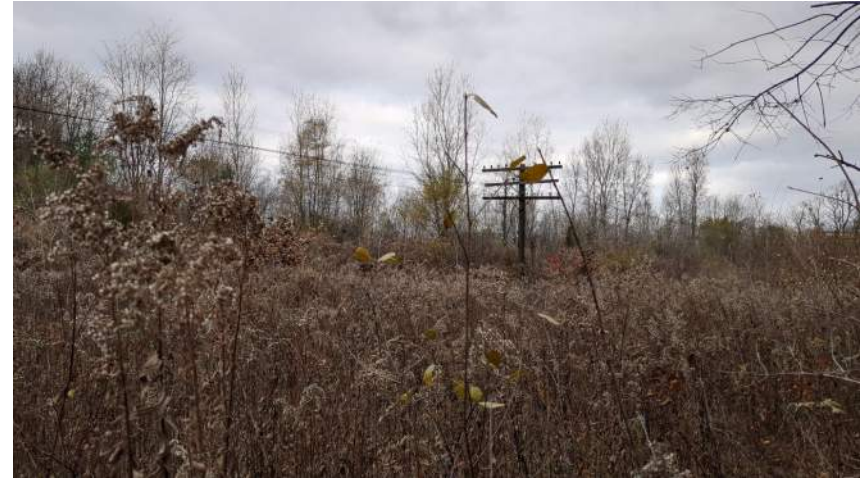
PP06, Facing West
