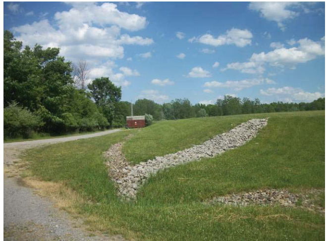
Photo 4: Former RCRA Landfill looking east.
