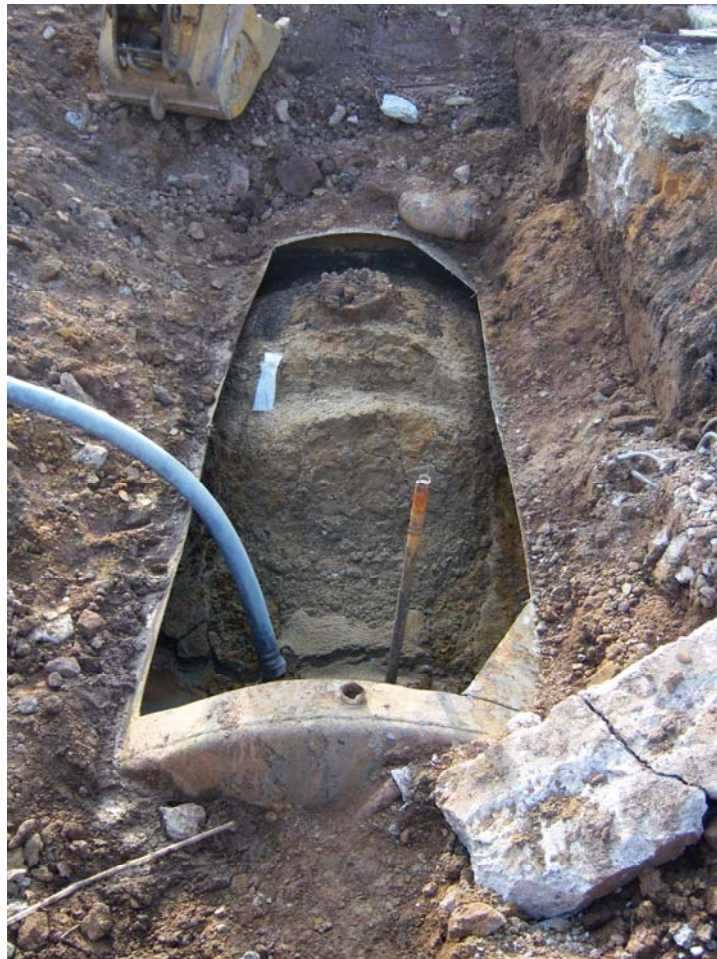
10,000 gallon UST Opened
