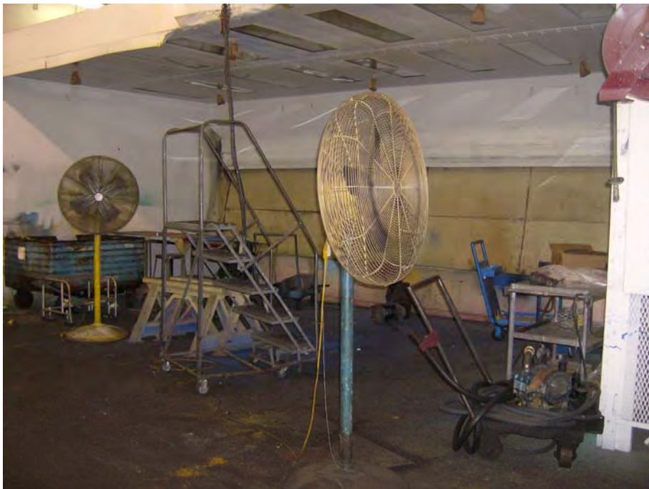
Photo 6: Maintenance paint booth
