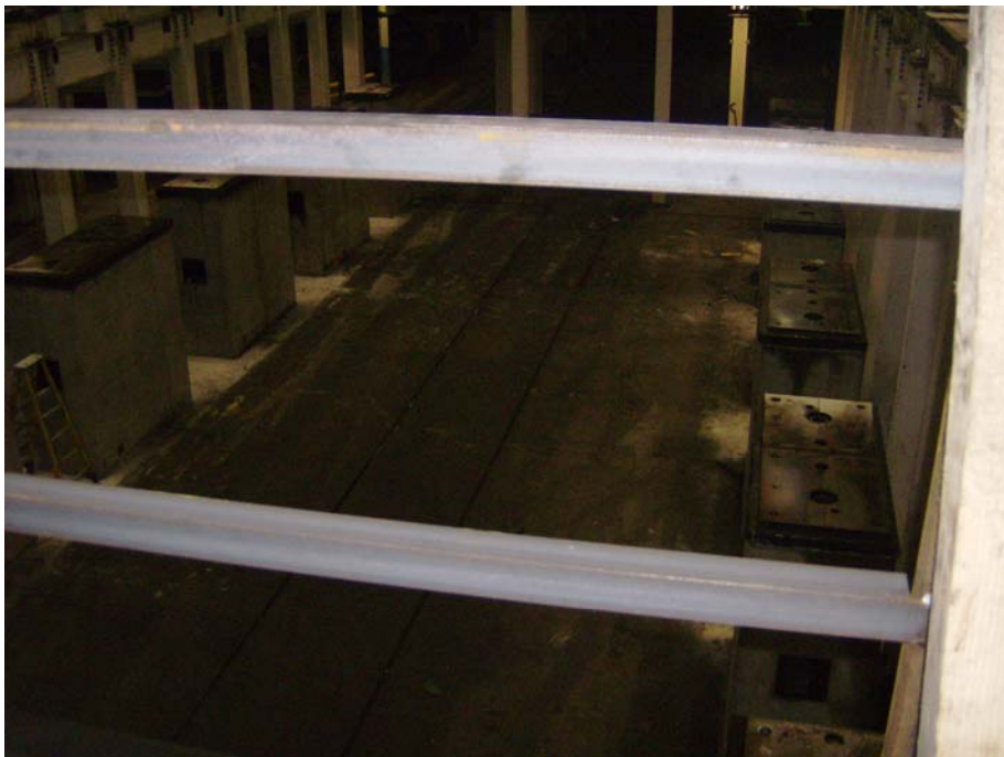
Photo 18: Former press pit (from first floor looking in basement)
