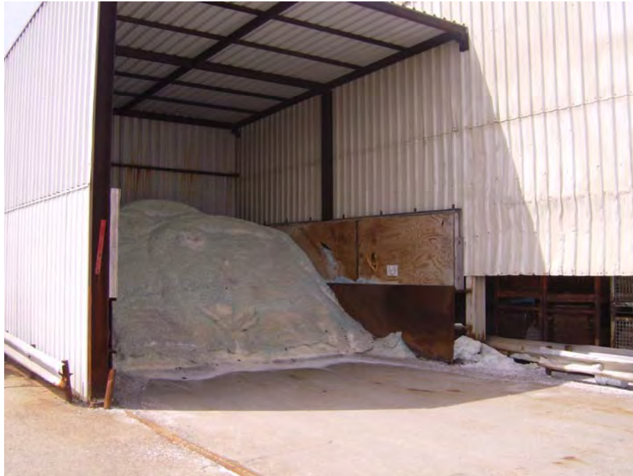
Photo 50: Salt storage area
