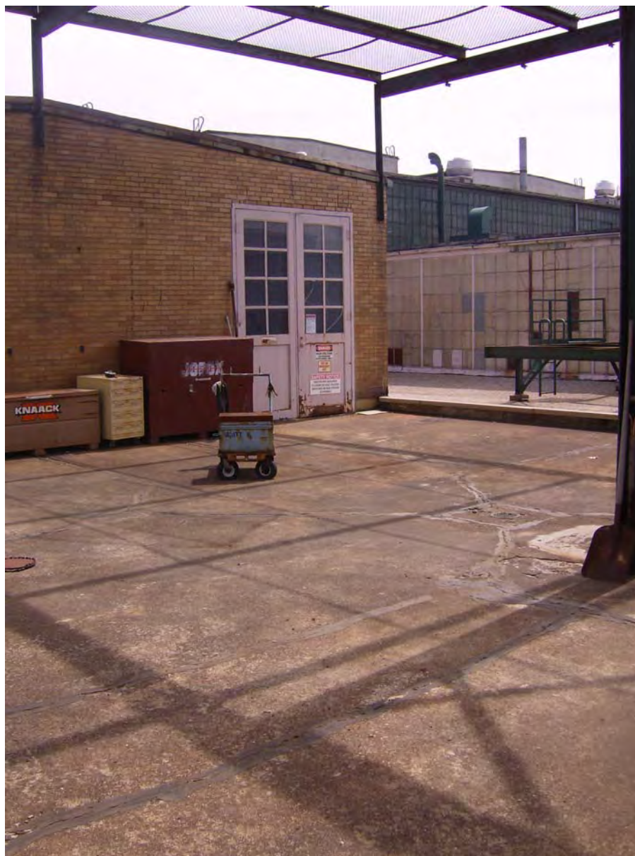
Photo 49: Potential exterior substation on roof
