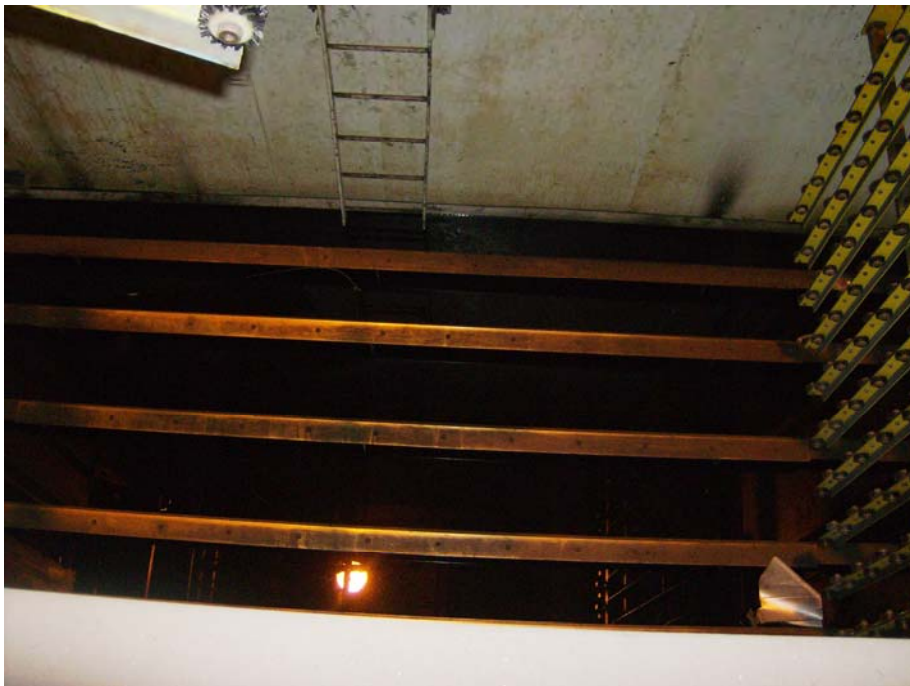
Photo 30: Oil in press pit
