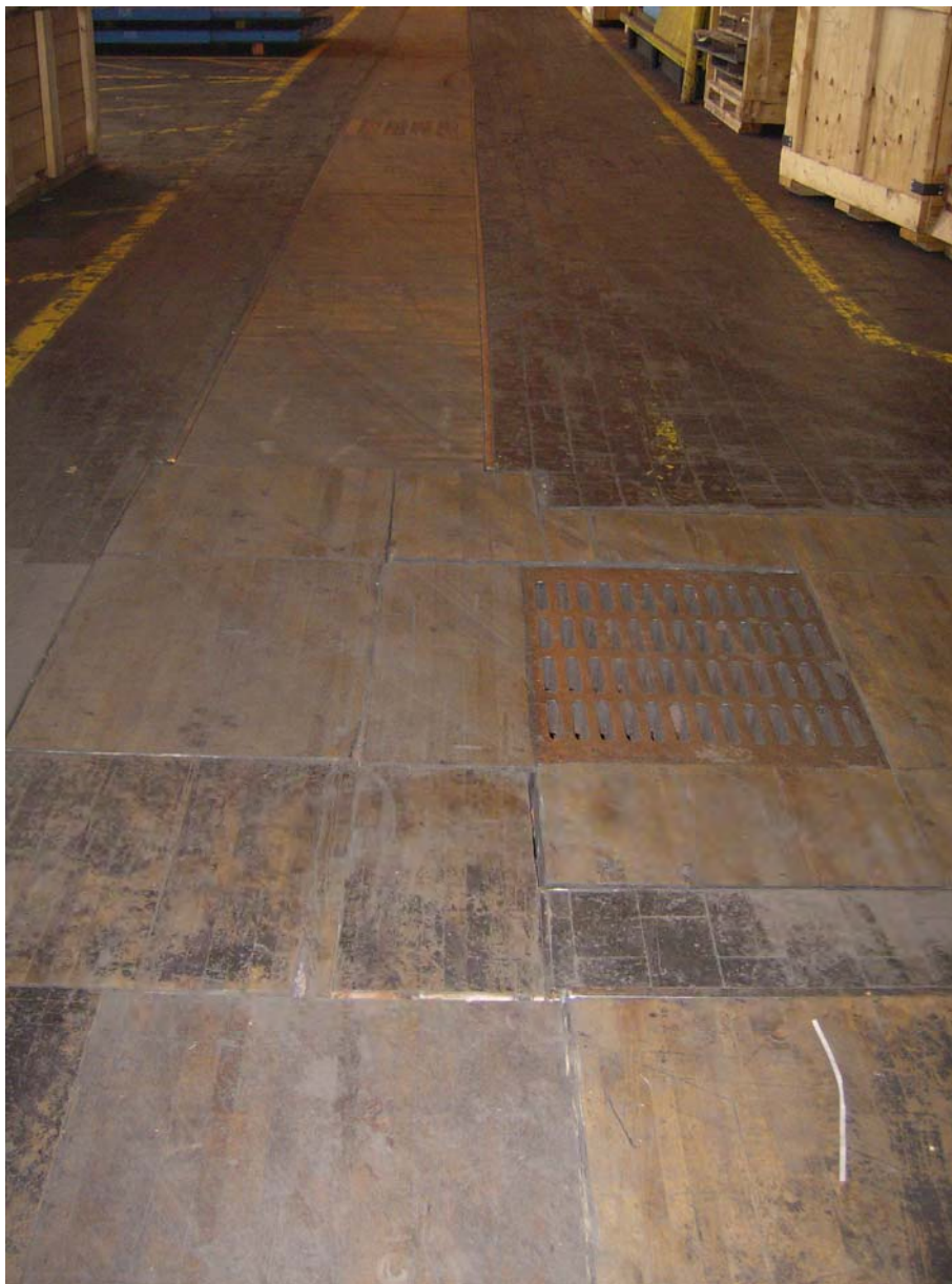
Photo 41: Grinding swarf trench in TDO
