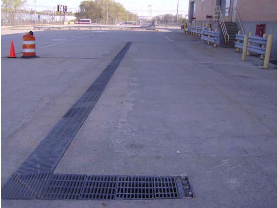
Photo 1: Containment trench in Oil Stores bulk unload area
