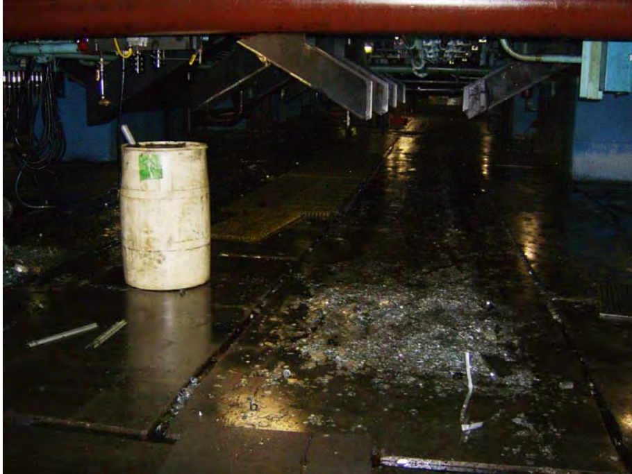
Photo 19: Scrap collection area in basement of Main Manufacturing Building
