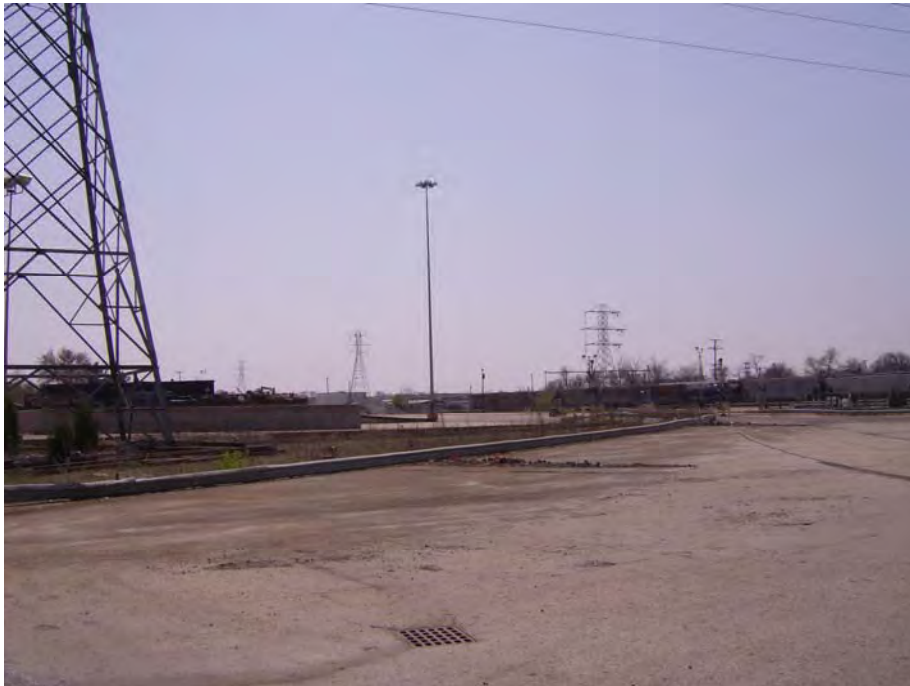
Photo 26: Southern portion of Site
