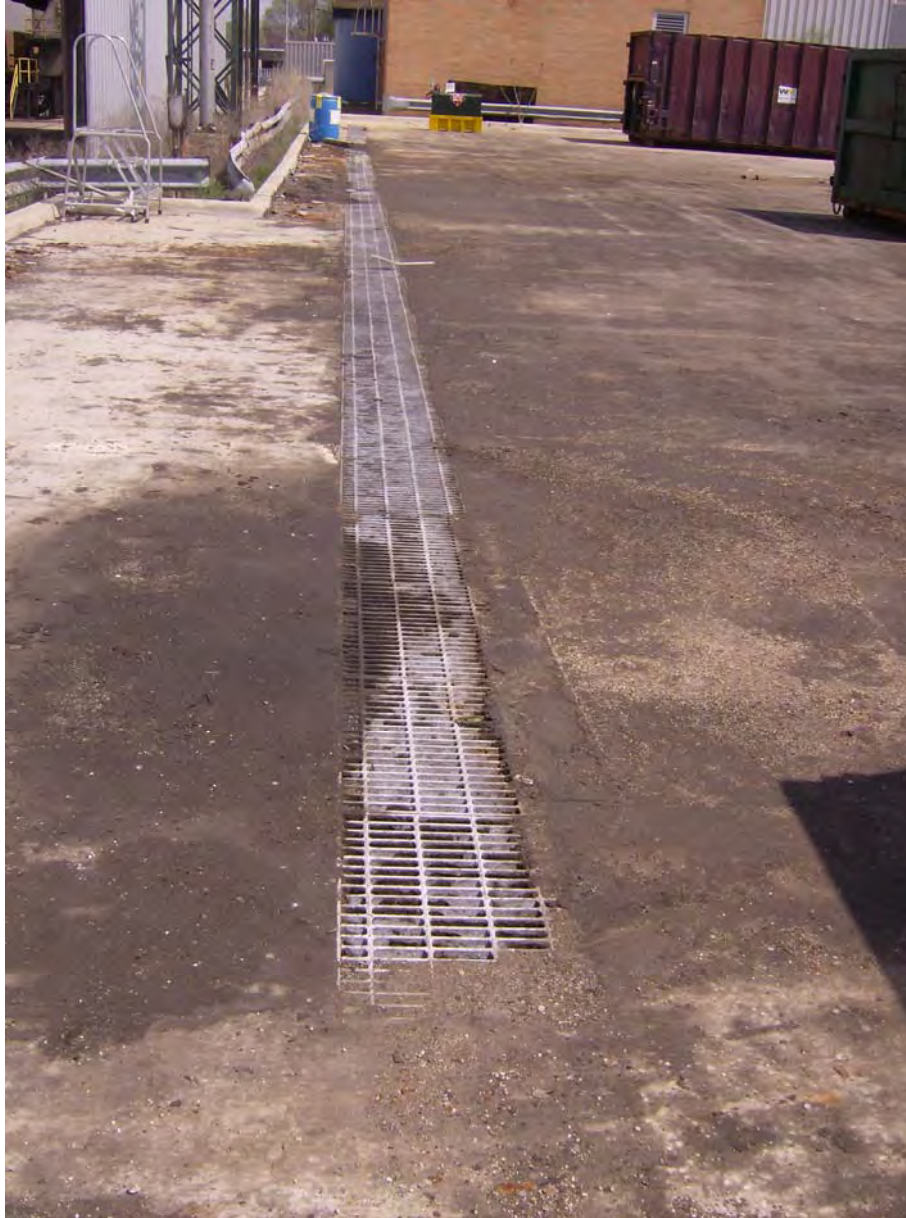
Photo 38: Trench in containment pad
