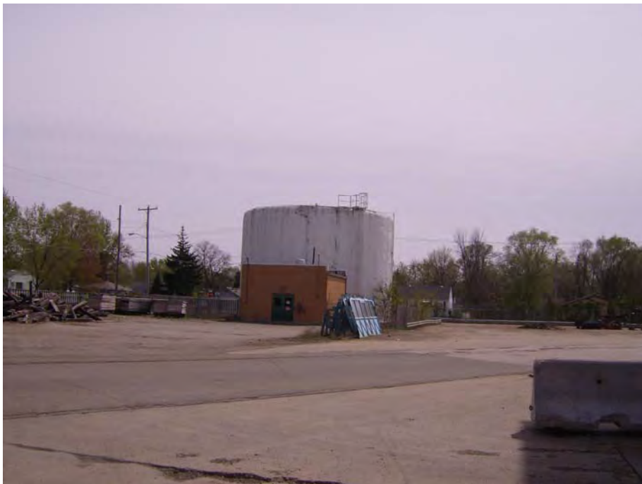
Photo 55: South Pump House
