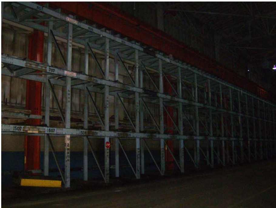
Photo 8: Former steel coil storage area
