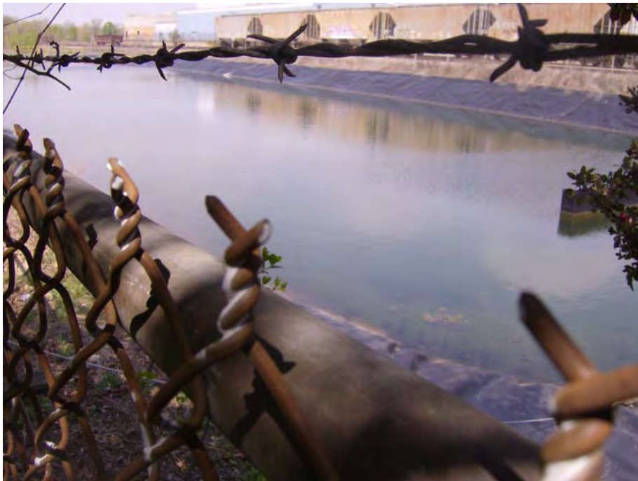
Photo 2: Stormwater retention pond
