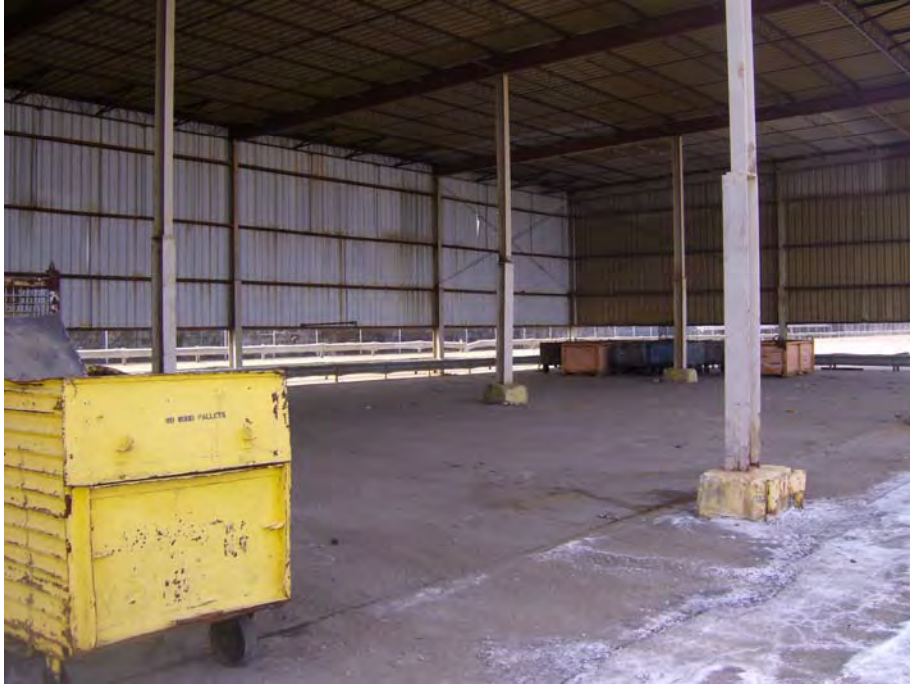
Photo 52: Metal storage shed
