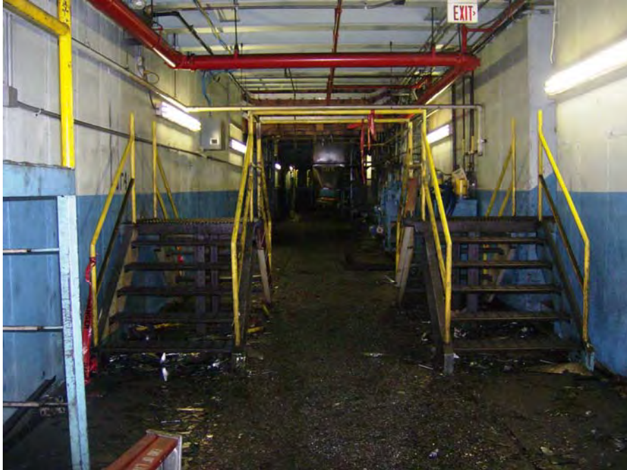
Photo 21: Basement tunnel under blanking presses
