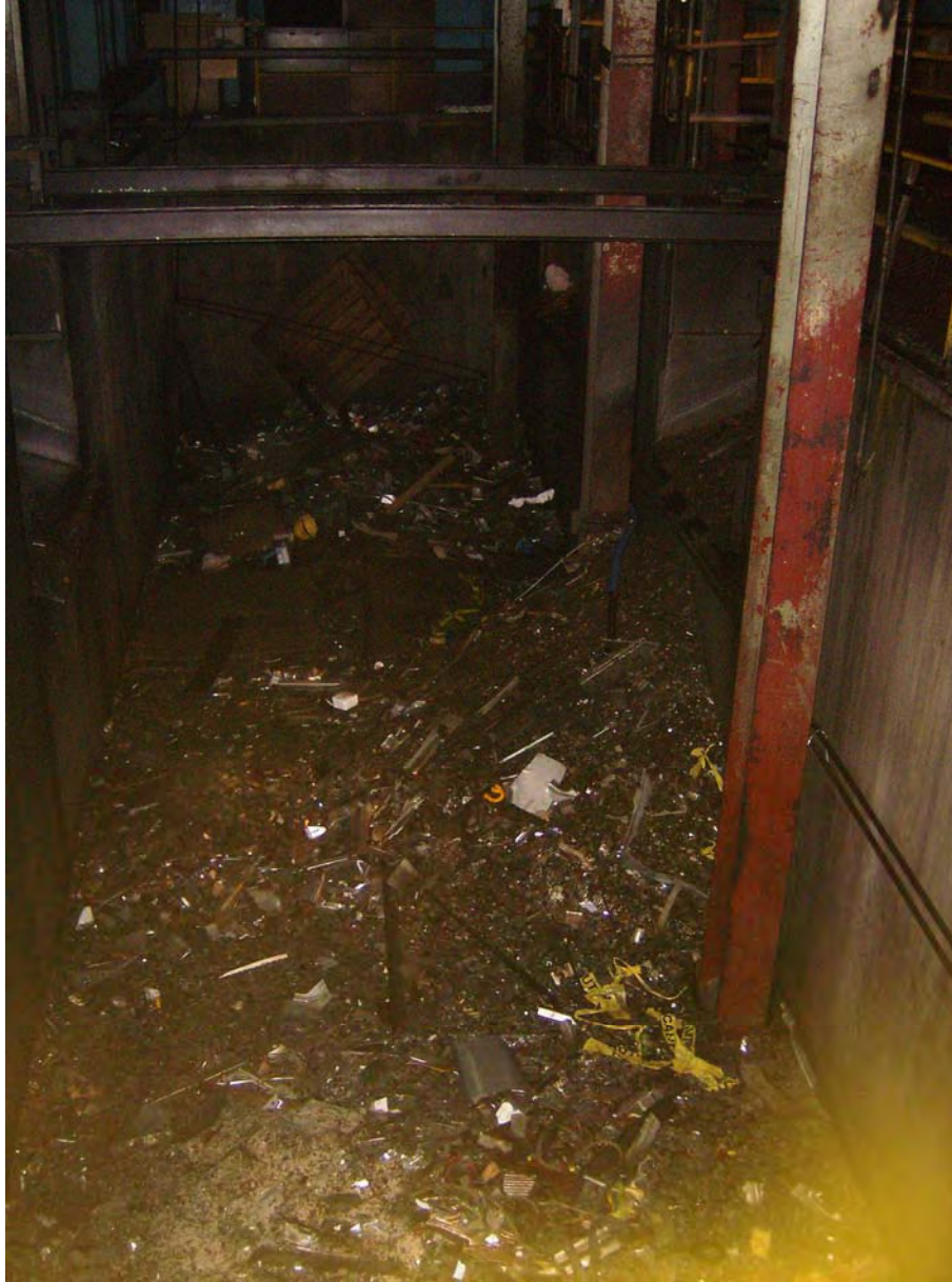
Photo 46: Oily scrap in Baler House pit
