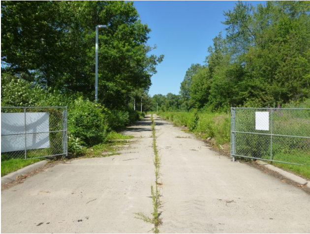
Photo #1: View of access road at entry facing west
