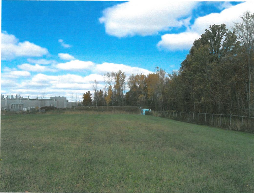
Minerals 009 – view of Minerals Processing Soil Cap from south end looking north. Date: 10/12/10. Time: 1:05 pm
