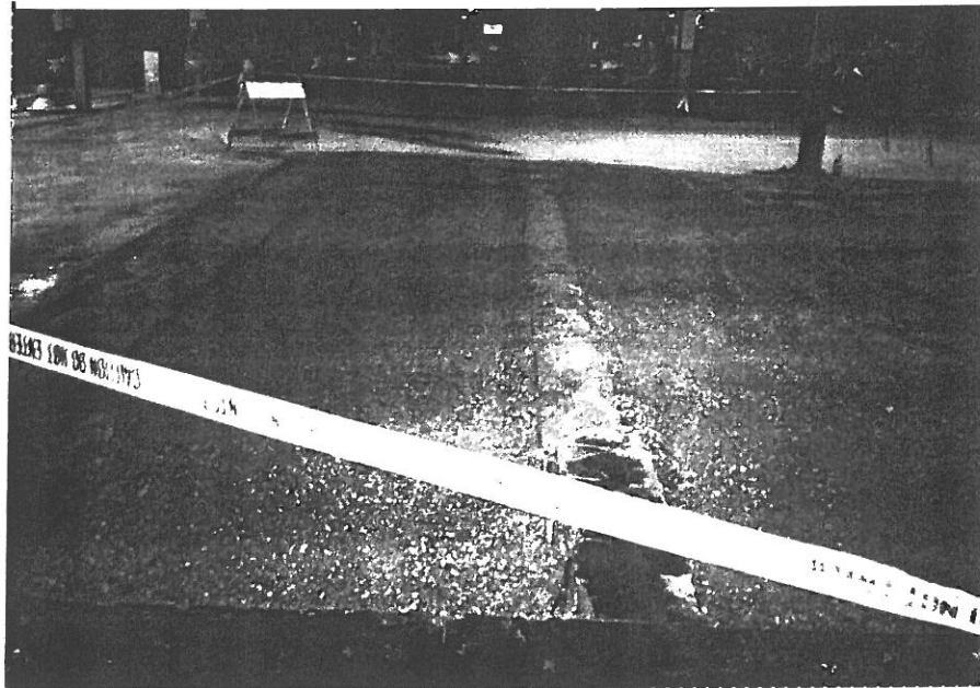
PHOTO 14 - ESP BACKFILLED WITH CRUSHED ROCK
