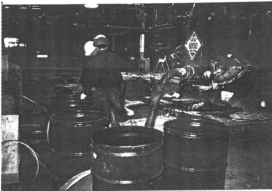
PHOTO 6 - LIQUID REMOVED FROM TANK BEING TRANSFERRED TO 55-GALLON DRUMS
