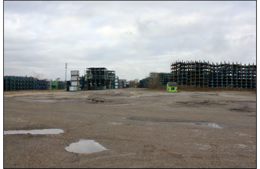
Photo 18: Southeast project area, looking west over racking.
