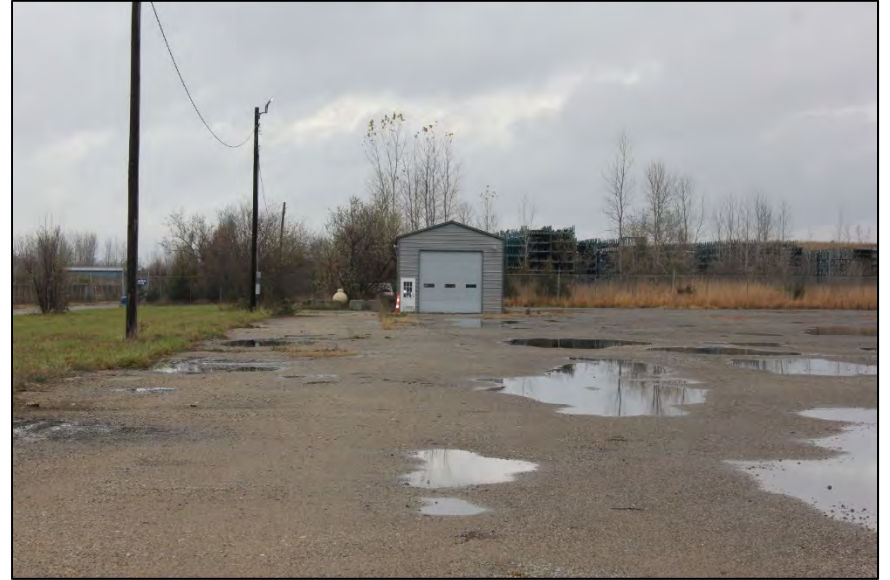
Photo 14: Maintenance/storage building, looking north.
