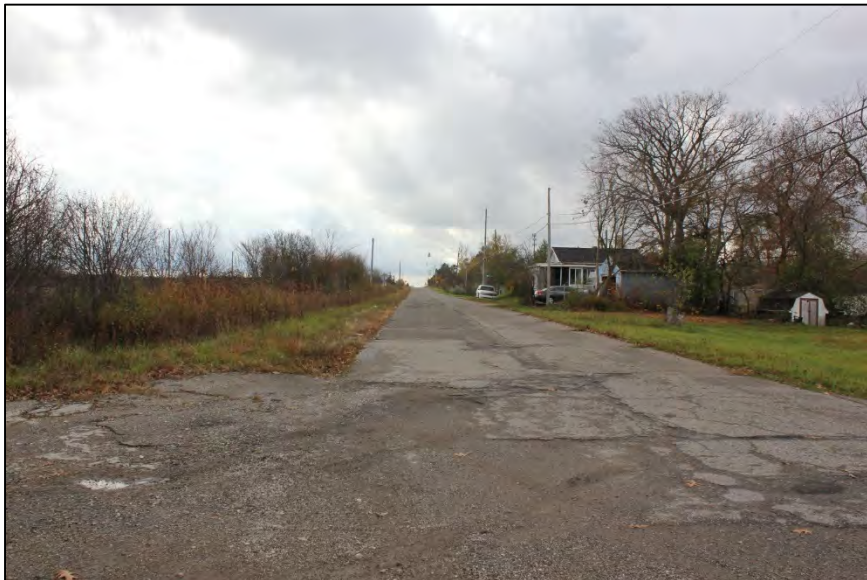
Photo 47: Looking south down Horton Avenue along western edge of project area.
