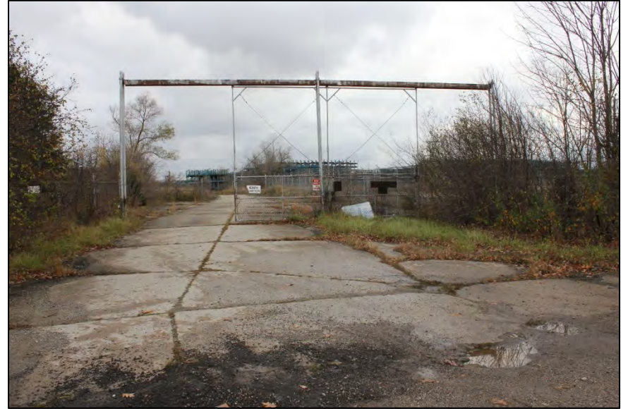
Photo 46: Northwest entrance gate to project area, looking east.
