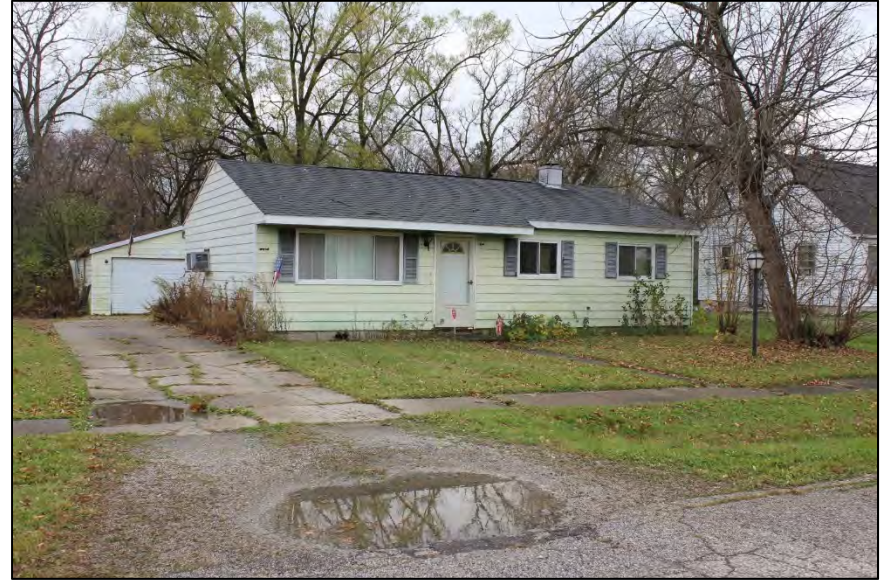
Photo 22: 1312 E Kurtz Avenue, looking southwest. Built 1960.
