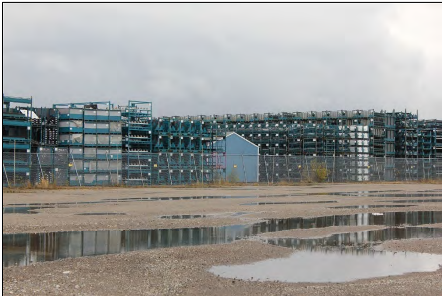
Photo 15: Racking and infrastructure within project area, looking southeast.
