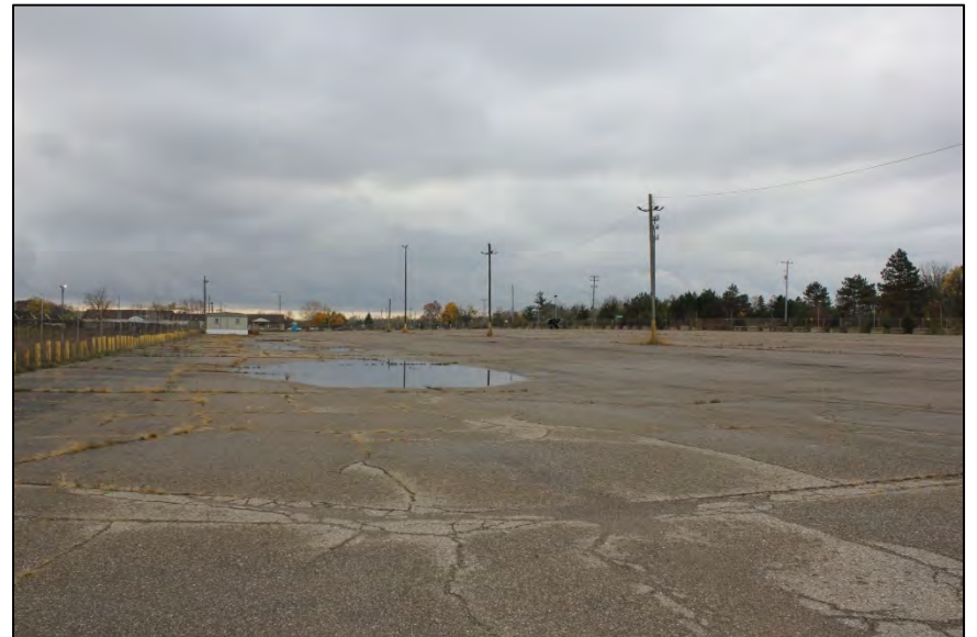
Photo 12: Parking lot on western edge of project area, looking southwest.
