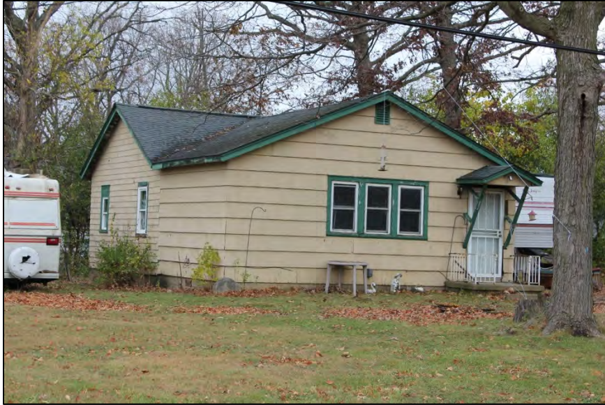
Photo 61: 1167 Morris Hills Pkwy, looking northeast. Built 1940.
