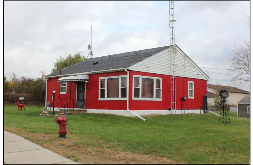
Photo 34: 5500 Horton Avenue looking northeast. Built 1955.
