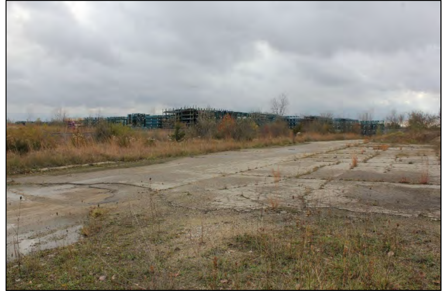
Photo 42: Looking southeast toward project area from northern edge of project area.
