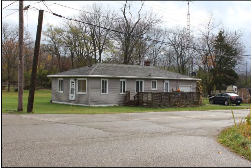
Photo 37: 1334 E Kurtz Avenue looking southeast. Built 1953.
