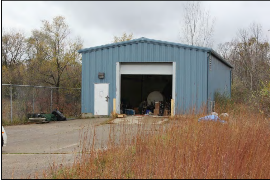
Photo 41: Maintenance shed at northern edge of APE, looking west.
