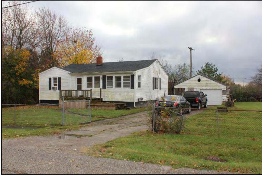
Photo 33: 1240 E Kurtz Avenue looking southeast. Built 1950.
