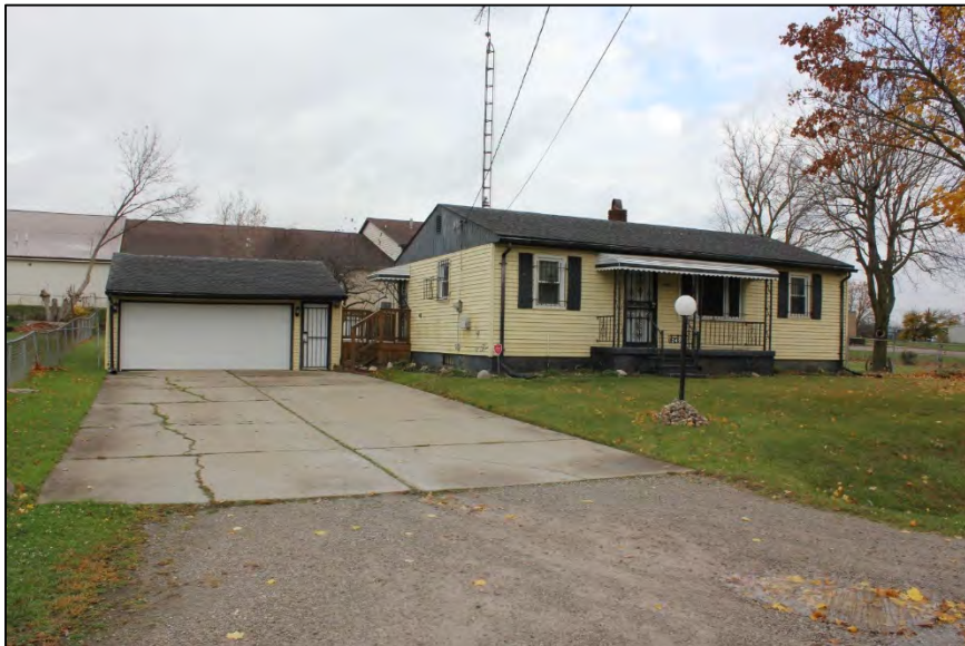
Photo 31: 1249 E Kurtz Avenue looking northeast. Built 1956.
