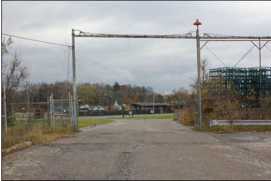
Photo 21: Southeast entrance gate to project area, looking southwest.
