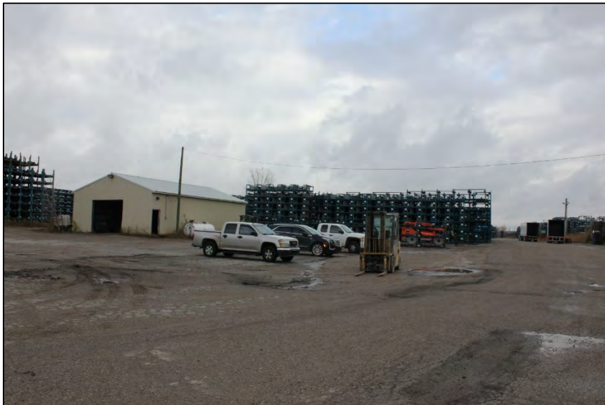
Photo 19: Southeast project area, looking northwest over maintenance/storage building and racking.
