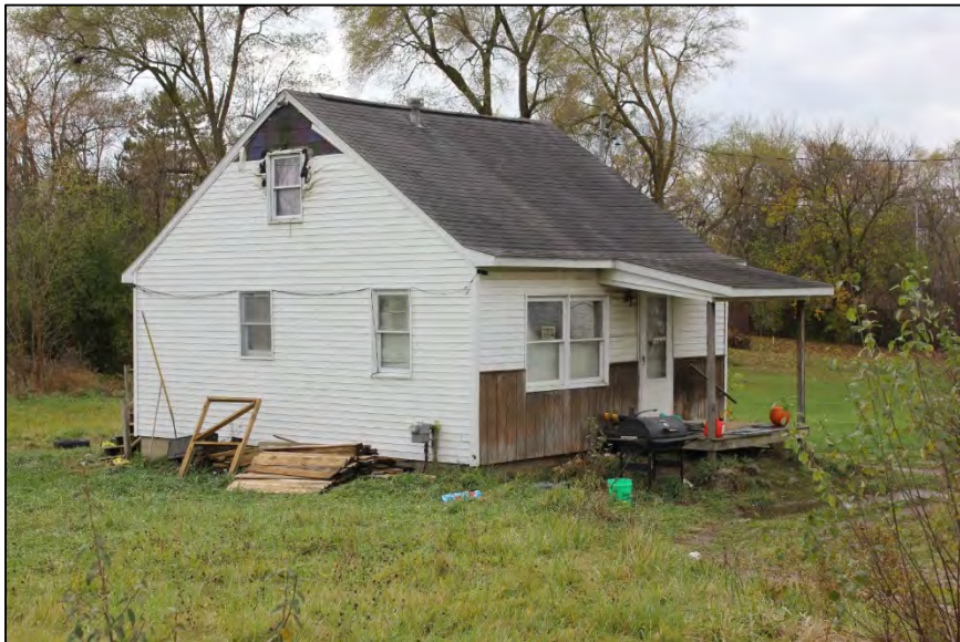
Photo 67: 1198 Dowagiac Avenue looking southwest. Built 1950.
