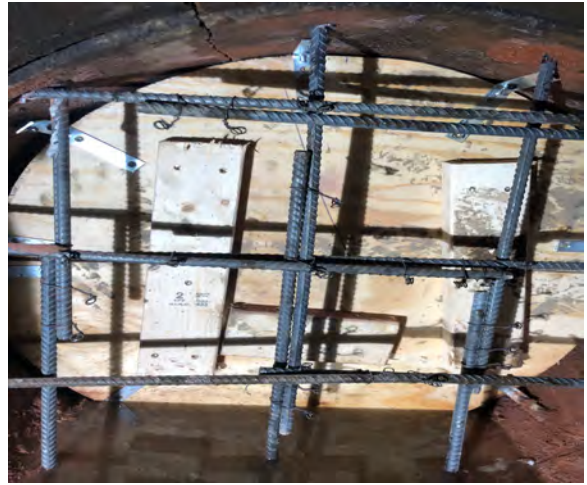
Back form with rebar
