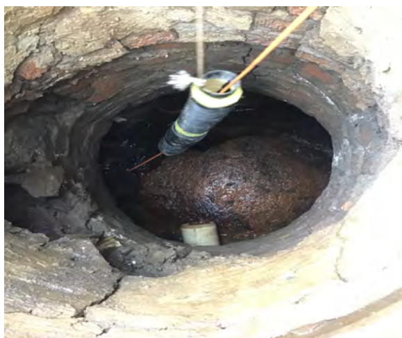
Concrete inside MichAve-MH-7
