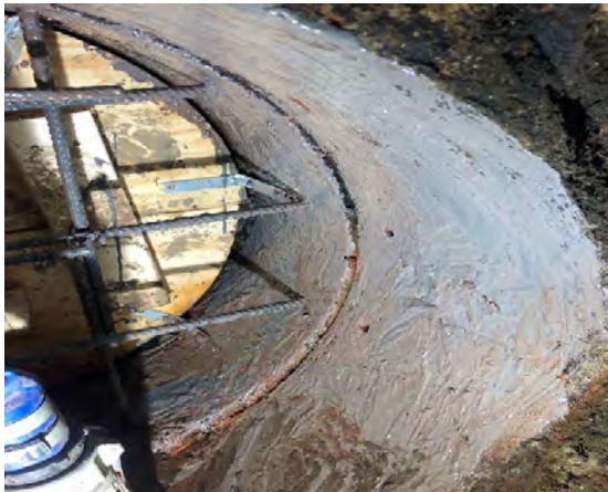
Photograph 9: Continued building of bulkhead form, using bonding agent
