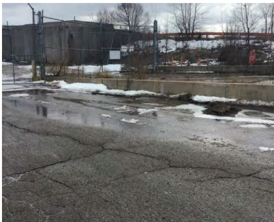
Photograph 29: Plant 6 Osborn entrance runoff inspection
