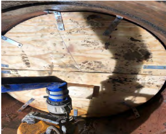
Photograph 7: Beginning of building bulkhead form in Plant 3 Sanitary Vault
