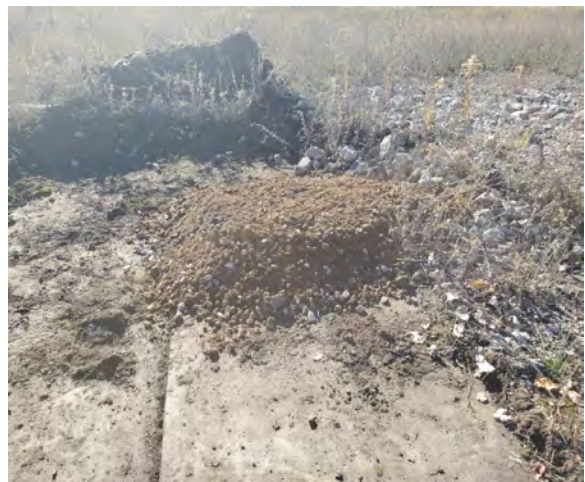
second completed catch basin capping
