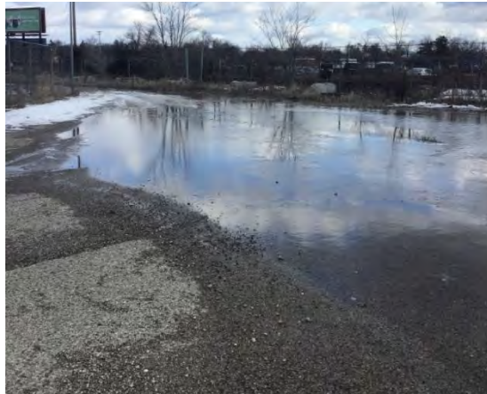
Photograph 20: Plant 2 bridge to Plant 3 runoff inspection
