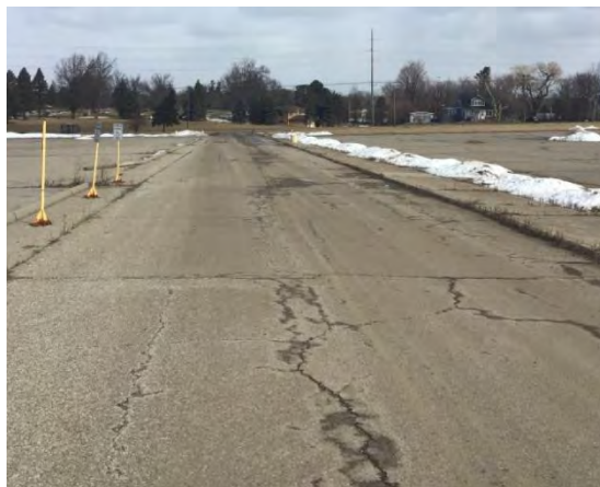
Photograph 24: Plant 3 Willow Street parking lot runoff inspection
