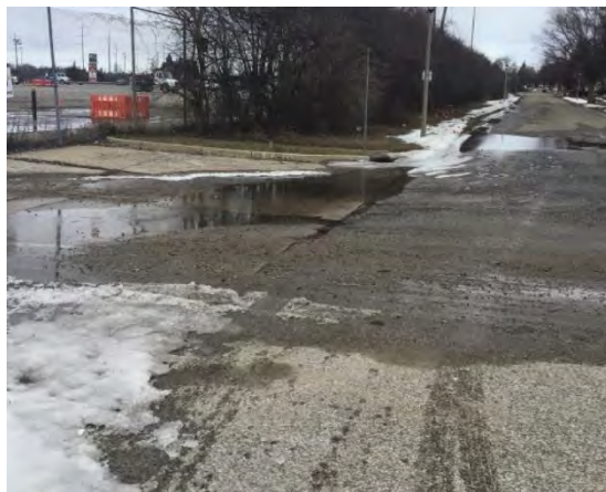
Photograph 30: Plant 6 intersection with Osborn and Stanley runoff inspection
