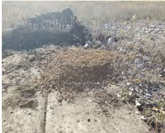
Photograph 2: Typical capped catch basin
