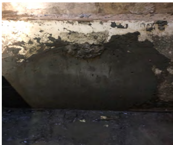
Plant 3 vault bulkhead with form removed
