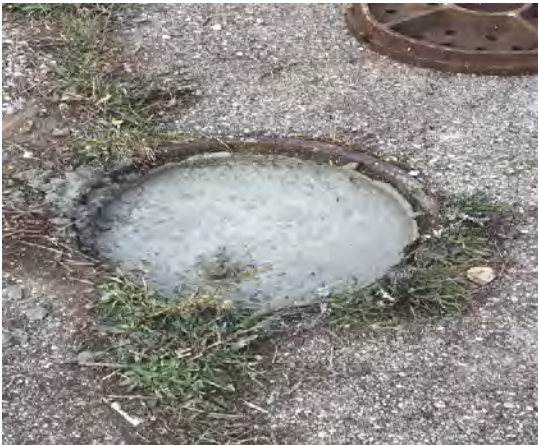
Photograph 3: Typical manhole filled with concrete to ground surface
