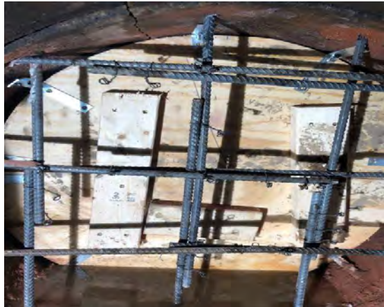
Photograph 8: Continued building of bulkhead form
