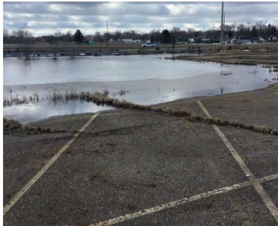
Photograph 28: Plant 3 southern parking lot runoff inspection
