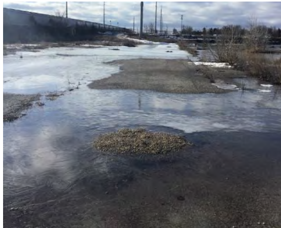
Photograph 22: Plant 2 eastern boundary runoff inspection
