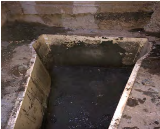
Photograph 13: Completed bulkhead after concrete pour
