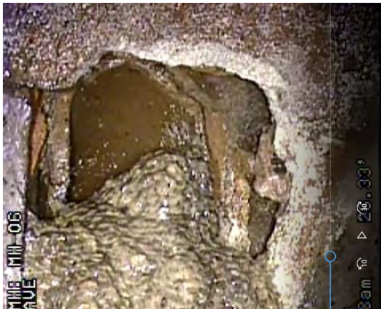
Photograph 15: Active pipe coming from Plant 6 along Verlinden
