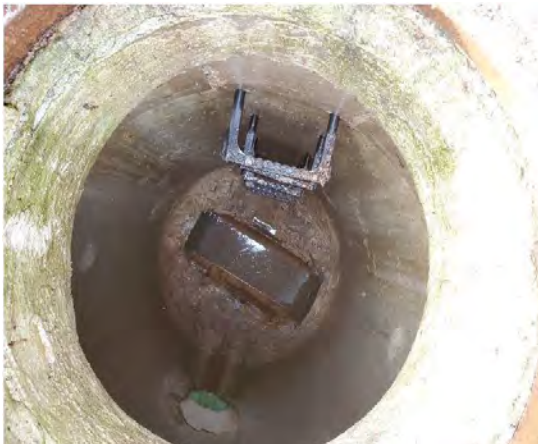
Photograph 1: Typical cleaned manhole to be filled with concrete
