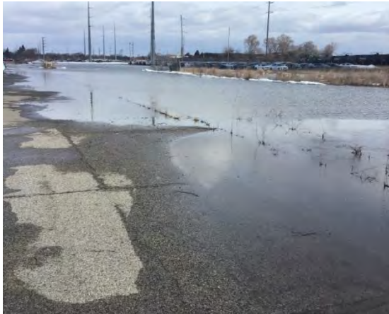
Photograph 25: Plant 3 eastern boundary runoff inspection
