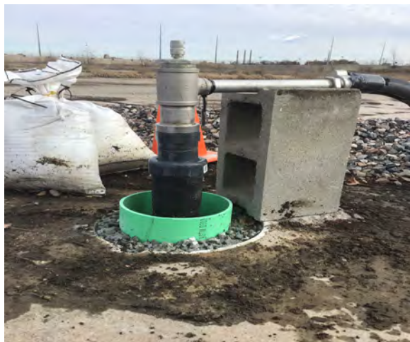
Well vault seal
