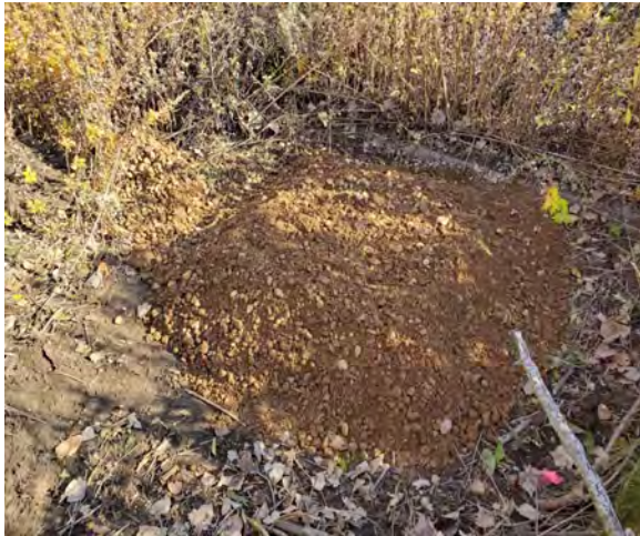
first completed catch basin capping
