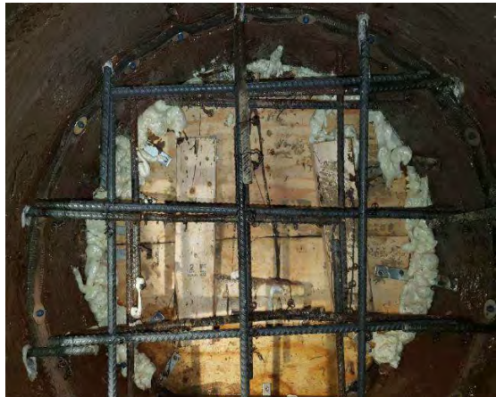
Photograph 10: Continued building of bulkhead form, using more rebar
