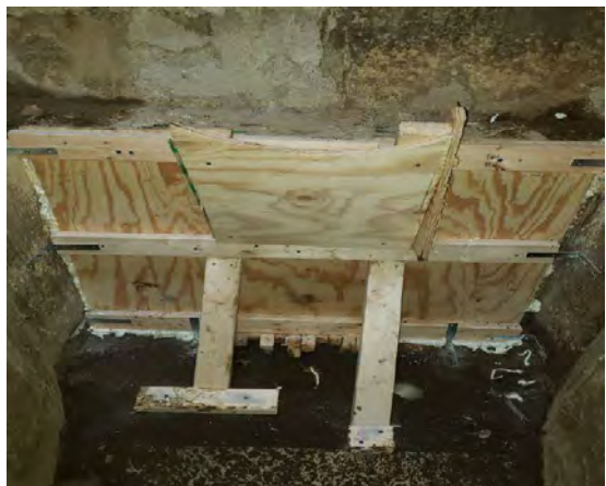
Photograph 12: Bulkhead form, view from inside vault
