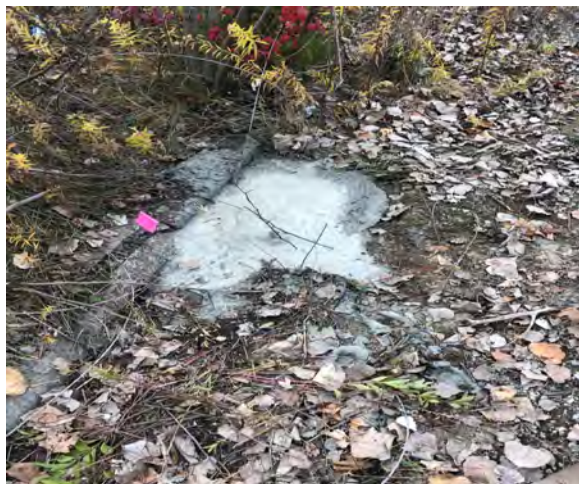
Filled catch basin
