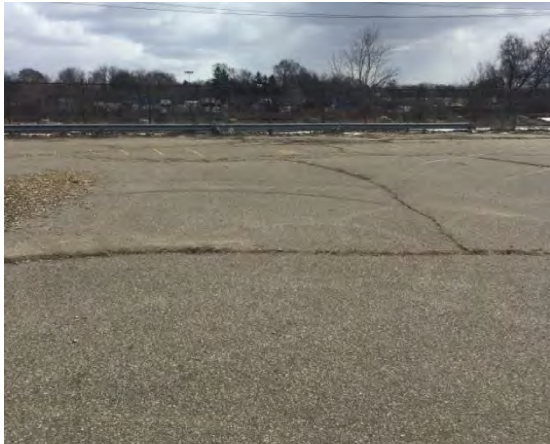
Photograph 19: Plant 2 northeast corner runoff inspection
