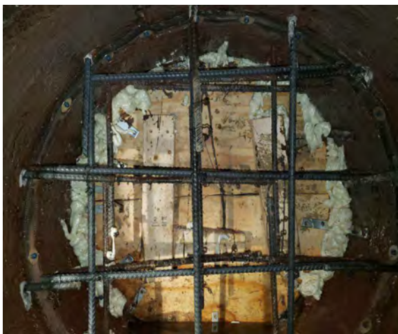
Second layer of rebar
