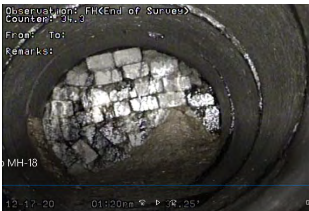
Photograph 17: Zoomed in view of "cut and cap" upstream of property boundary
