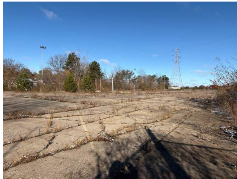
PP01, Facing Northwest
