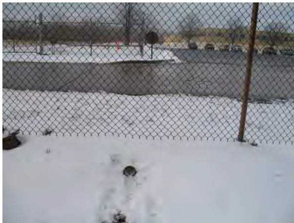
Photograph 3. View of a polyvinyl chloride discharge pipe located along the western boundary of the Site, adjacent to the General Motors SPO facility.
