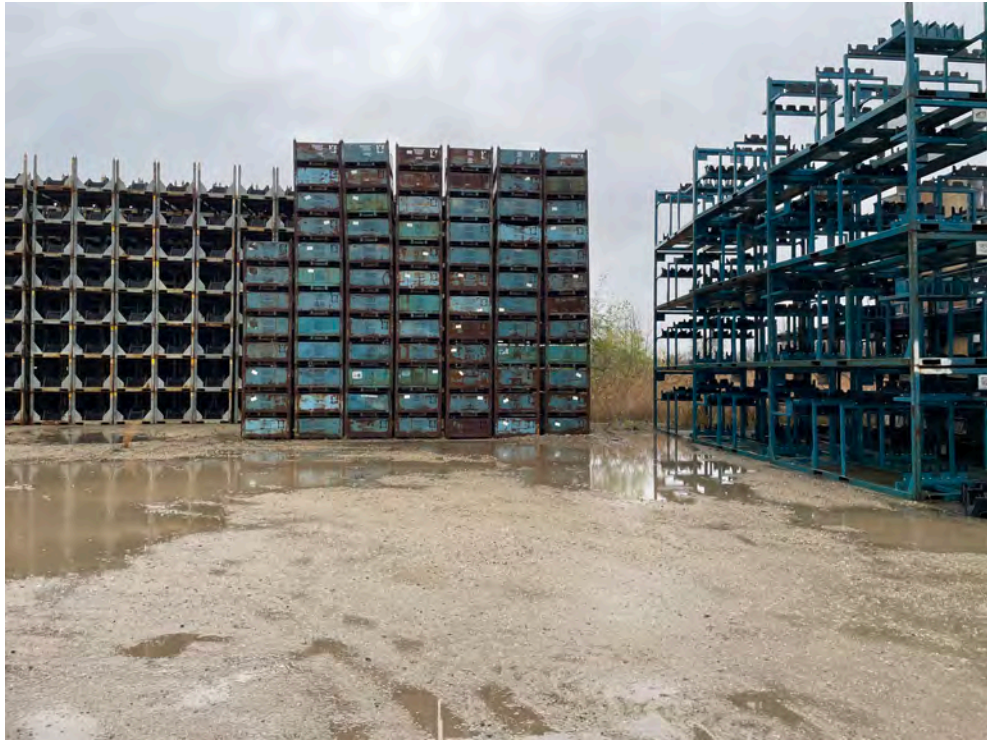
Steel racks being stored at the facility
