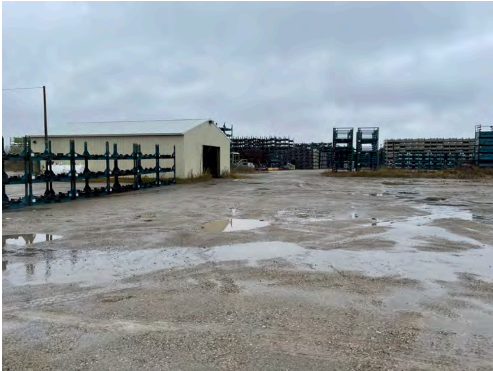
Steel racks being stored at the facility
