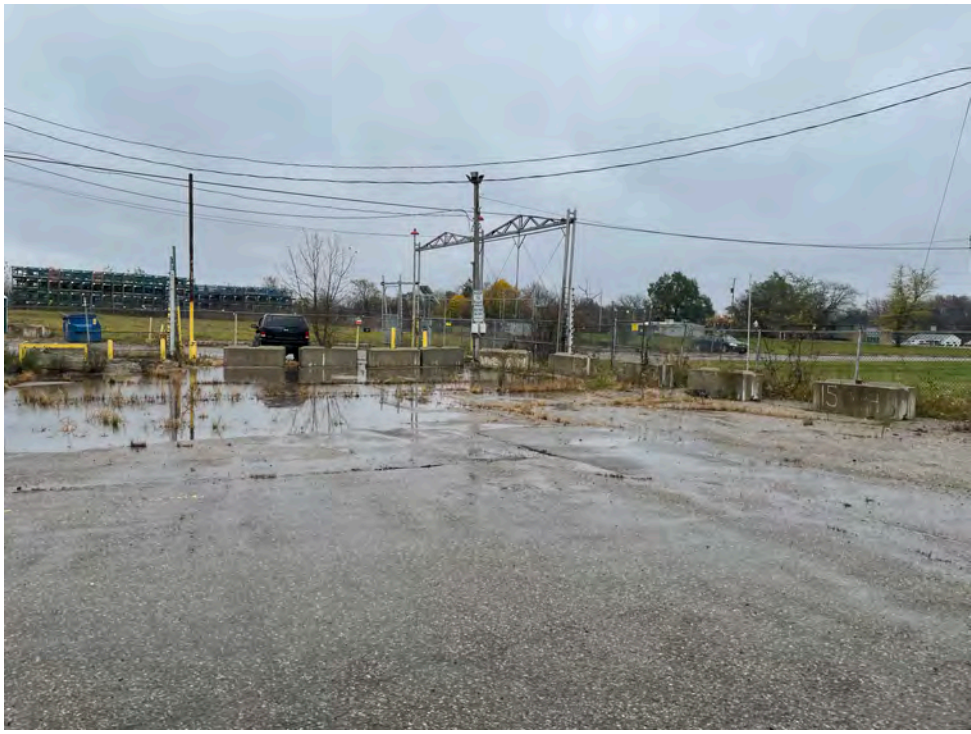
Southern entrance of facility, facing southeast
