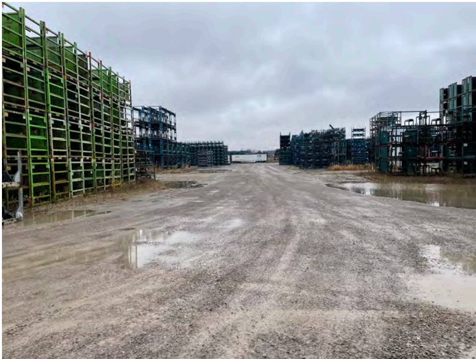
Steel racks and semi trailers being stored at the facility
