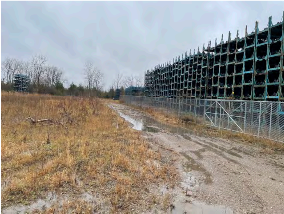
Steel racks being stored at the facility
