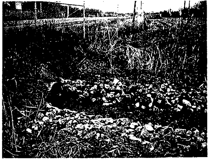
Photograph 6-View of area near CB-3
