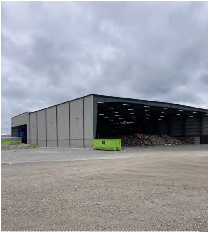
Building addition to existing assembly plant that was constructed last year in use located in northern portion of property
