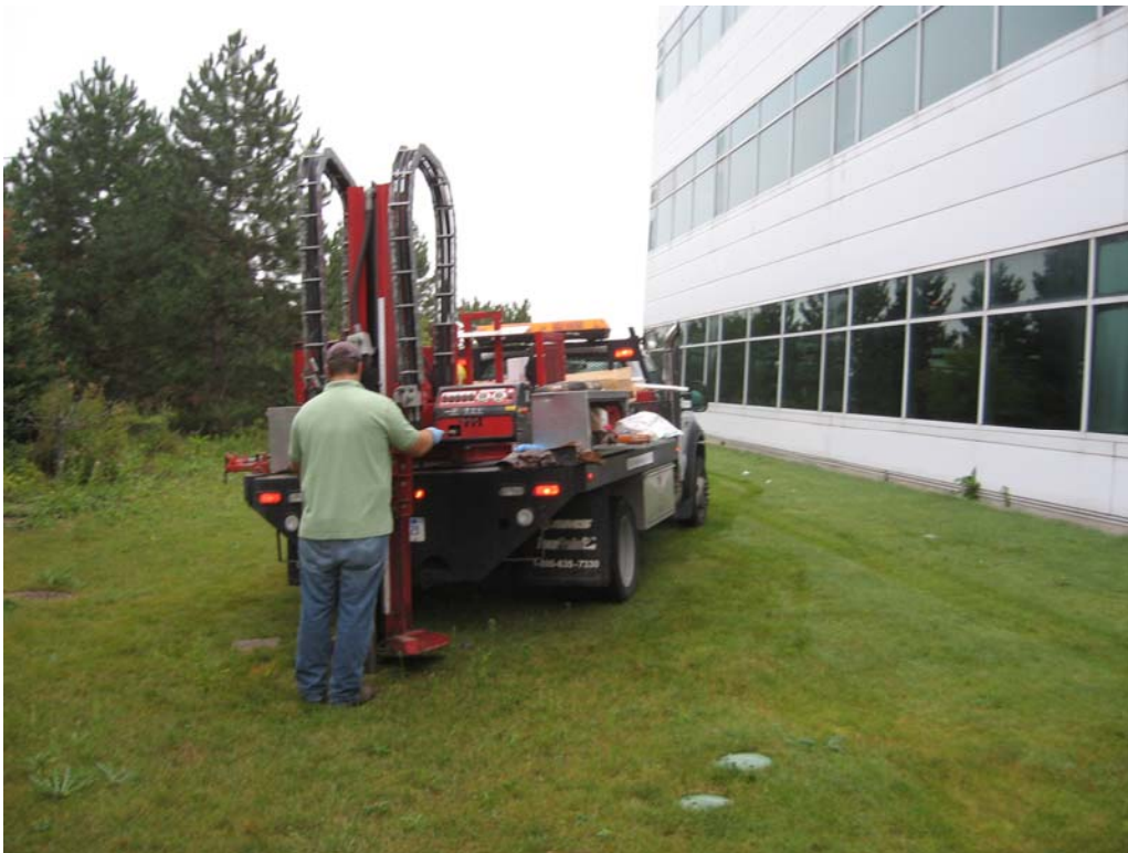
Photo 6. View of the completion of soil boring SS-11
