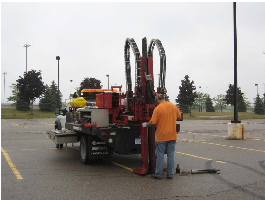
Photo 4. View of the completion of soil boring SS-3
