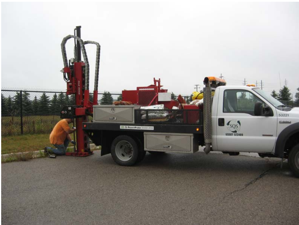
Photo 3. View of the completion of soil boring SS-5
