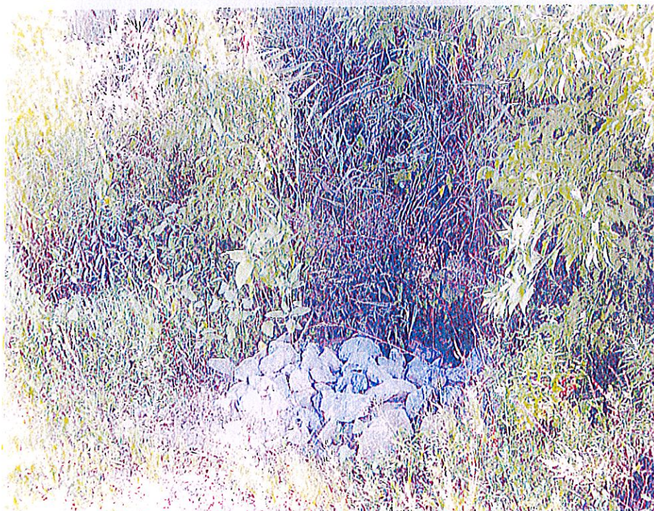
Photograph 12: Rip-rap repair at bank erosion location near the outfall from CB-3.
