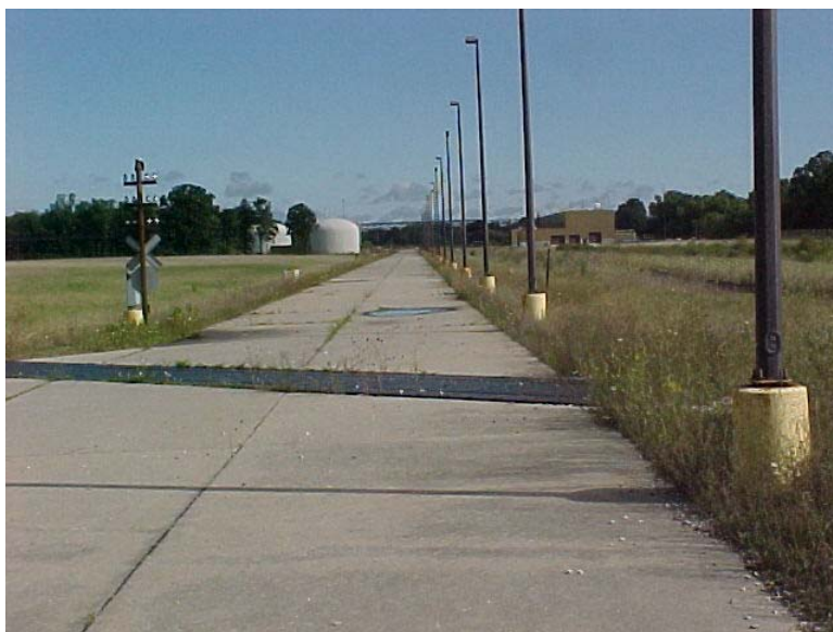
Photograph 11: Rail siding, water tanks and Waste Water Treatment Building, facing north.
