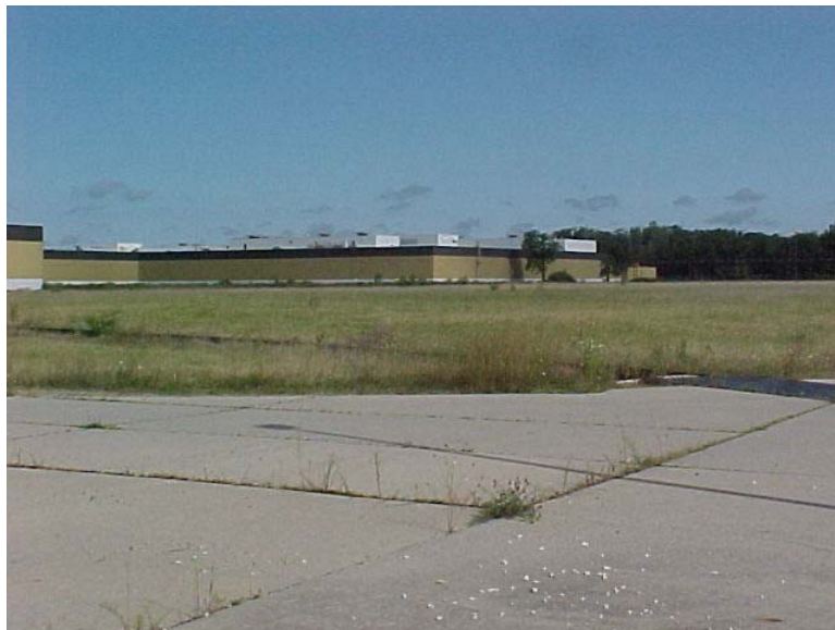
Photograph 10: East side of building 502 facing northwest.
