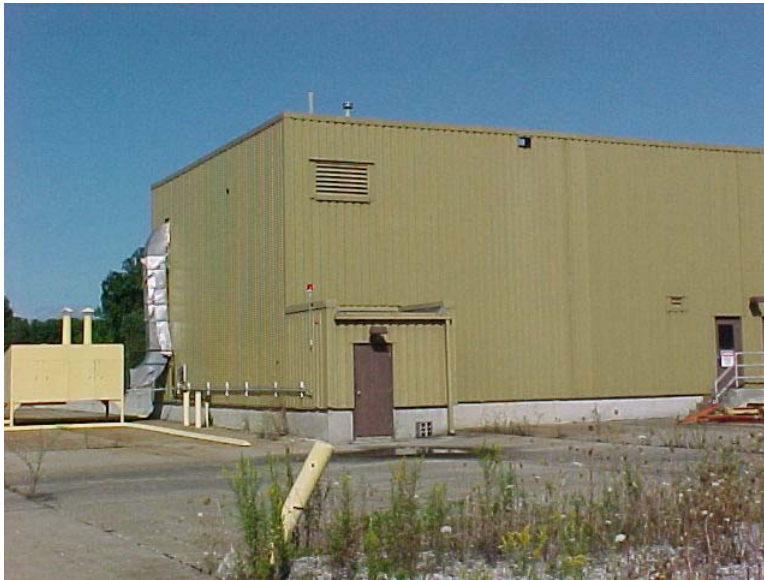
Photograph 17: Combustible/Flammable material and Hazardous Waste Storage Building (#566).
