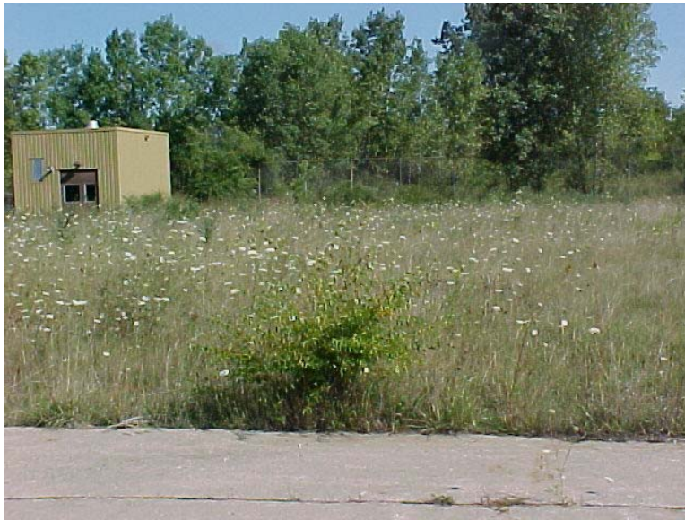
Photograph 19: North retention pond pump house (#568) and wooded northern portion of the Site (background).
