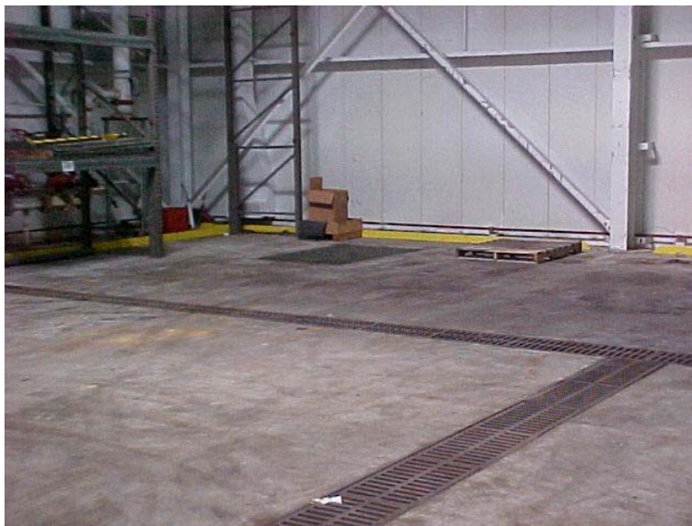
Photograph 18: Interior of Building 566.
