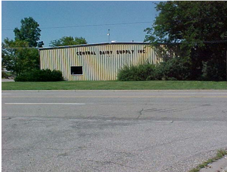
Photograph 25: Adjoining commercial property on the west side of Canal Road.
