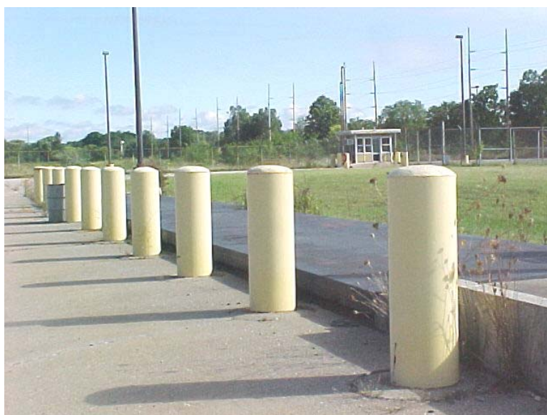
Photograph 12: Scale (foreground) and Gate House (#580).
