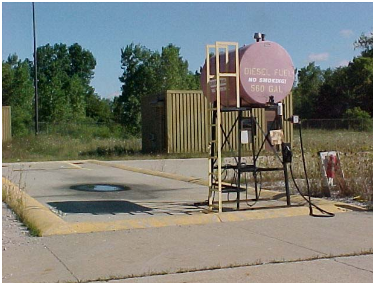
Photograph 24: Diesel tank and containment pad adjoining the east side of the north tank farm and the tank farm control house (#567, background).
