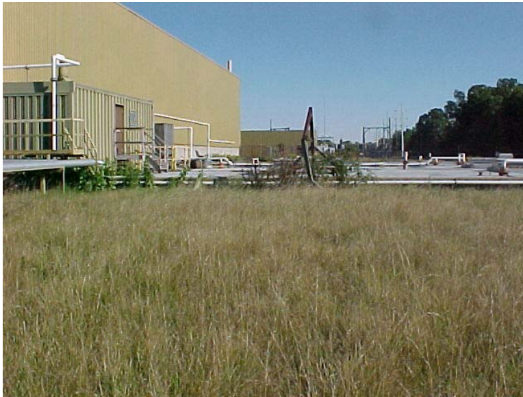
Photograph 7: Below grade portion of Waste Water Treatment Building (east side of building).
