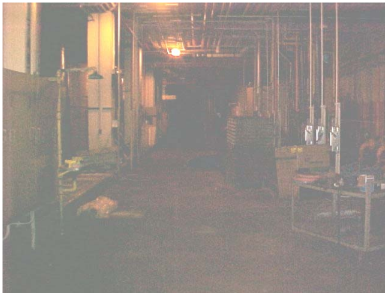
Photograph 6: Basement of Waste Water Treatment Building (#561).
