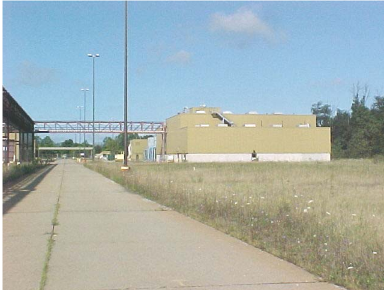
Photograph 15: Compressor Building (#565) facing west.
