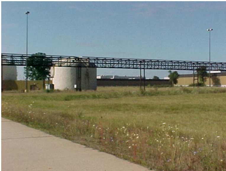
Photograph 14: Catwalk facing southwest.
