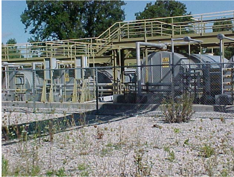
Photograph 23: North tank farm.
