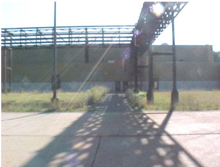
Photograph 4: Catwalk and Waste Water Treatment Building (#561).
