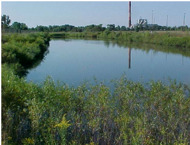
Photograph 8: South retention pond facing south.
