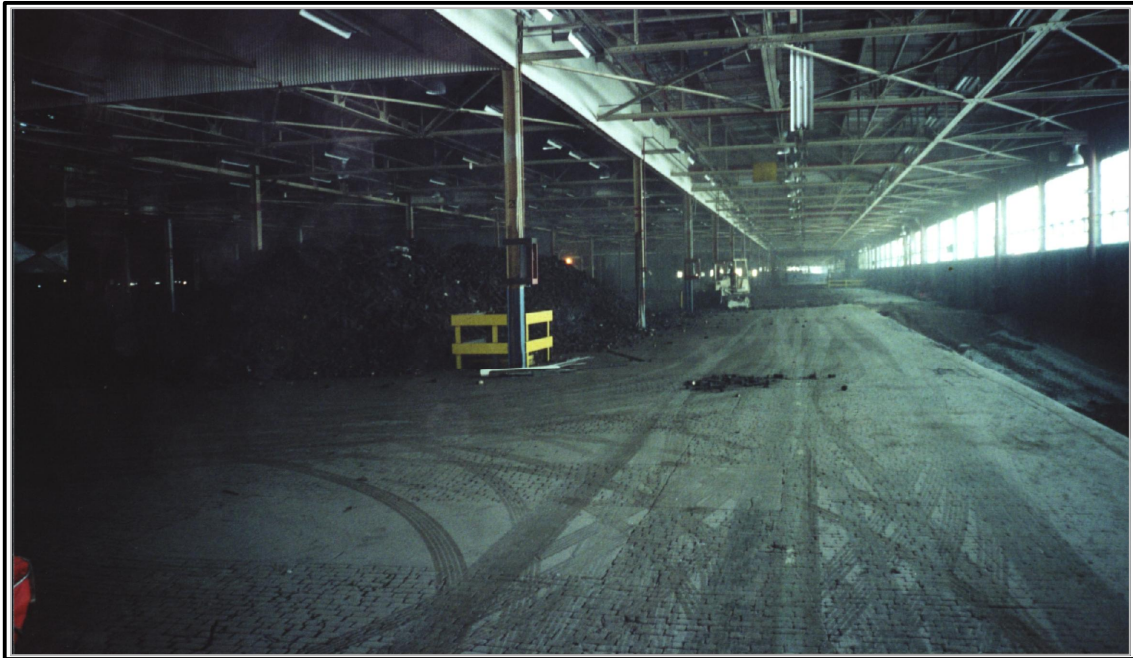
PHOTO #7 STAGED WOOD BLOCK FLOORING.
