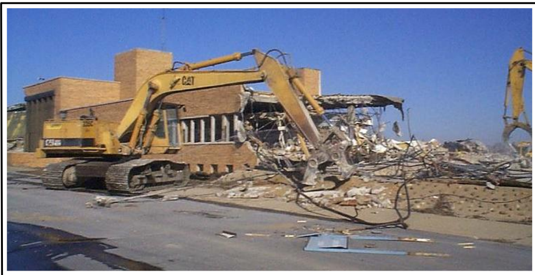
PHOTO 6: ADMINISTRATION BUILDING DEMOLITION
