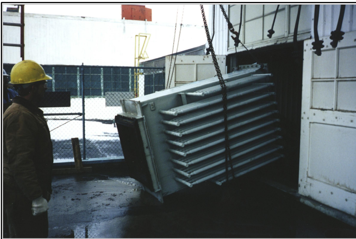
PHOTO #2 REMOVING TRANSFORMER FROM OUTSIDE ROOF TOP PAD INTO BUILDING 44.
