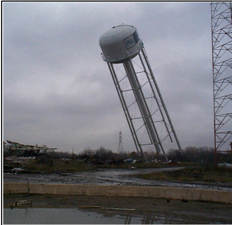
PHOTO 3: WATER TOWER DEMOLITION
