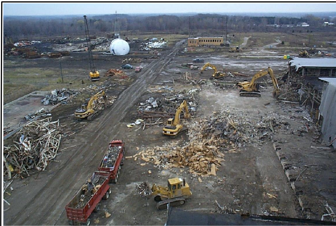
PHOTO 4: SORTING DEMOLITION DEBRIS
