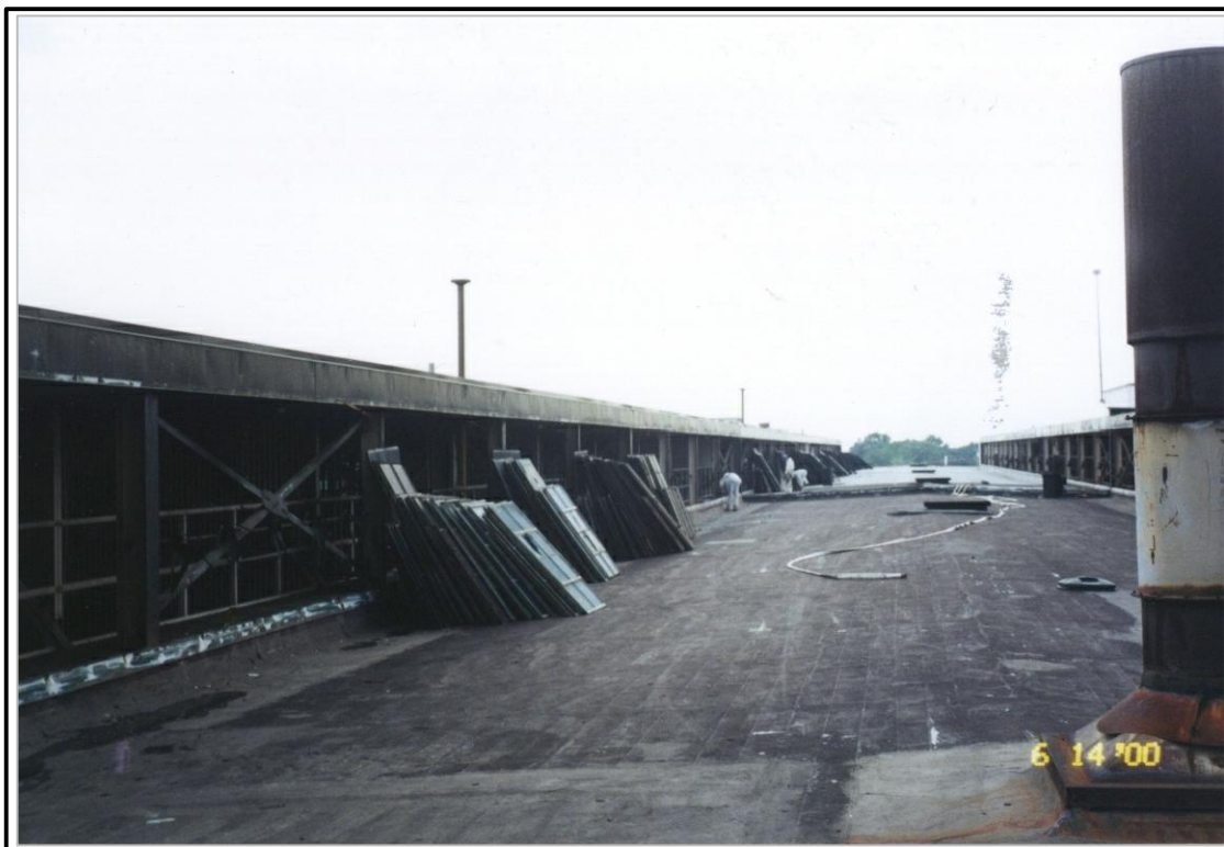
PHOTO #12 WINDOW PANE REMOVAL FROM BUILDING 44.
