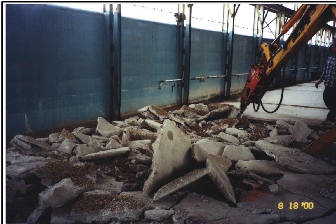
PHOTO #10 OPENING CONCRETE BINS IN BUILDING 63.
