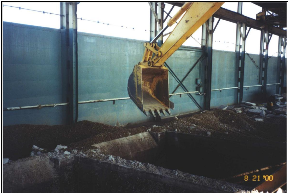
PHOTO #11 REMOVING MATERIAL FROM BINS IN BUILDING 63.
