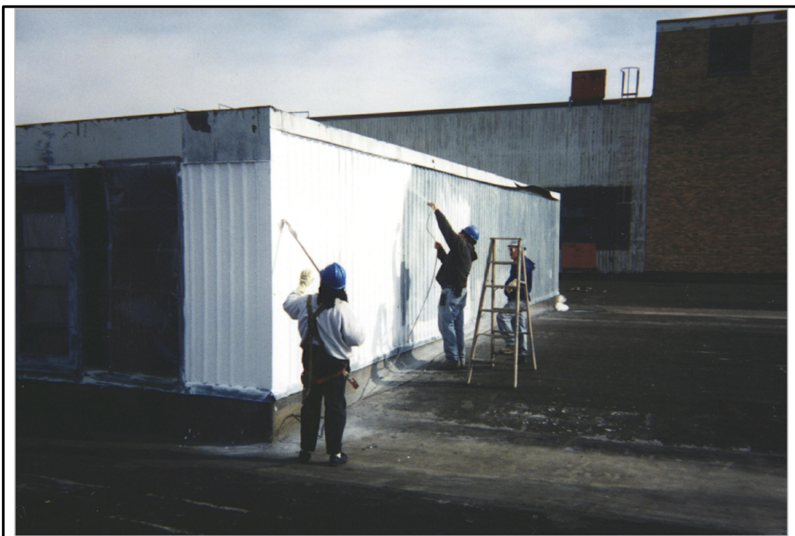
PHOTO #1 GALBESTOS ENCAPSULATION
