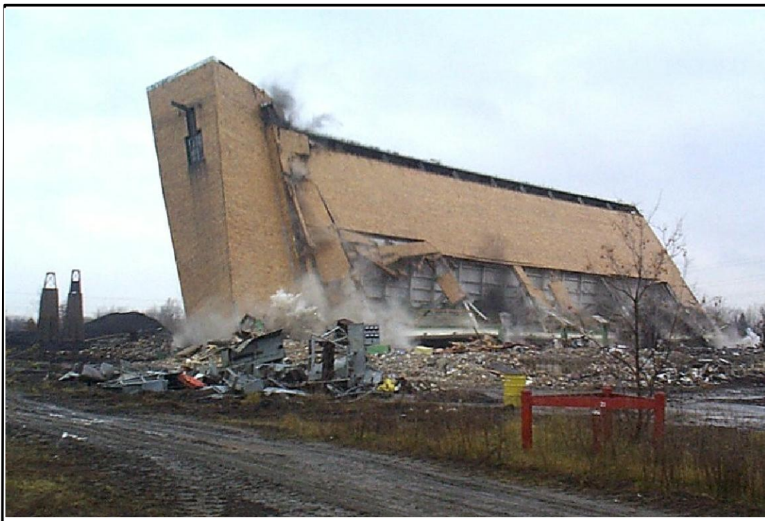
PHOTO 2: SOUTH WALL POWERHOUSE DEMOLITION
