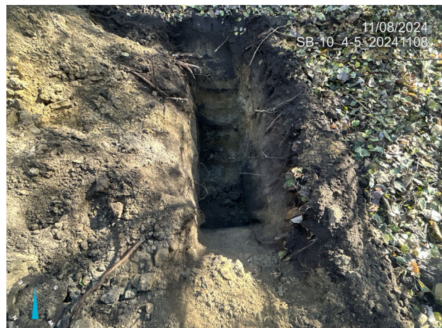
Test pit that was dug for gathering sample SB-10_4-5_11082024
