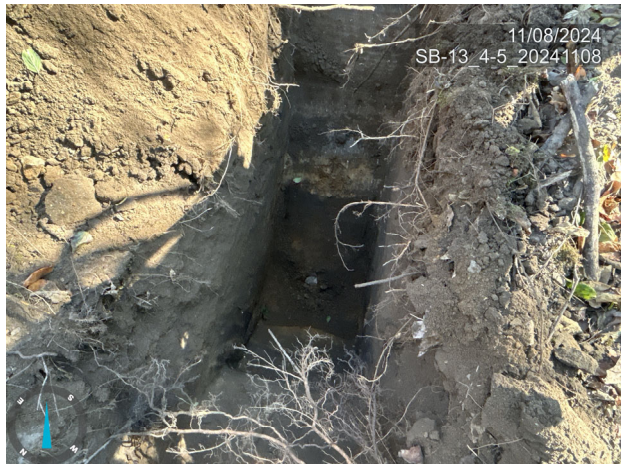
Test pit that was dug for gathering sample SB-13_4-5_11082024
