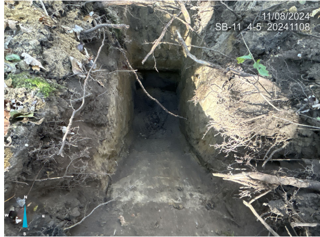
Test pit that was dug for gathering sample SB-11_4-5_11082024
