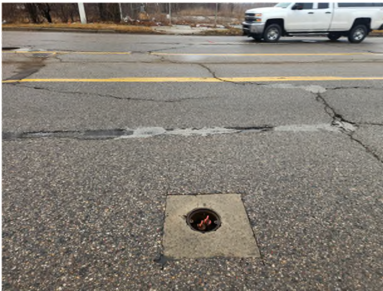
Monitoring well and MW-09-92
