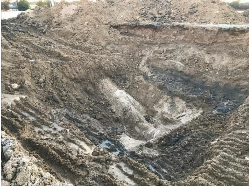
17: The crew excavated and daylighted the eastern storm interceptor.
