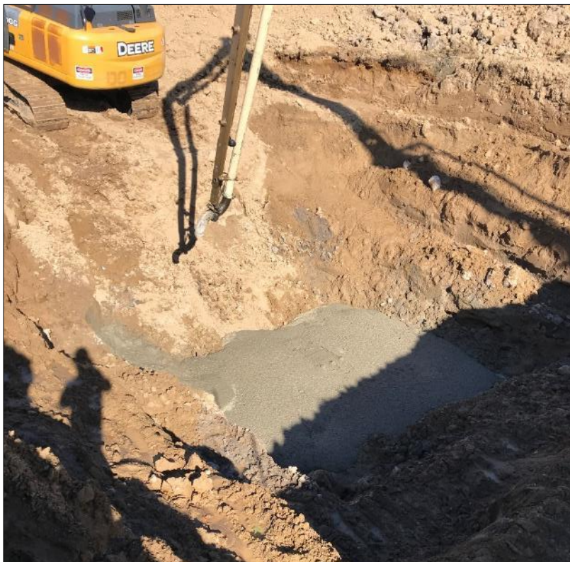
21: Eastern CLSM monolith being poured
