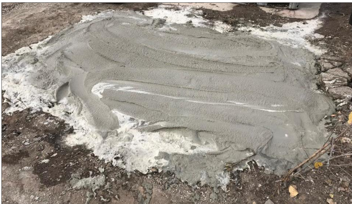
30: The former OWS after being filled with CLSM
