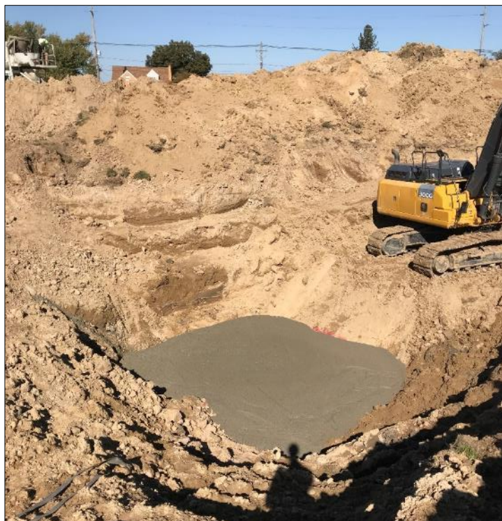
20: Western CLSM monolith after pouring was complete
