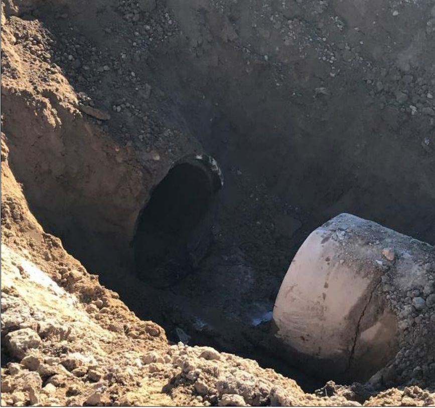
14: Sacrificial forms were installed in both of the exposed pipe ends. Note that the sacrificial form in the pipe on the right was placed beyond the separated pipe seam.
