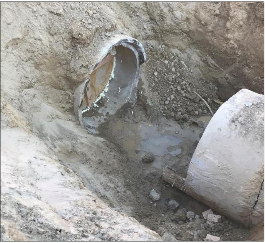
14: Sacrificial forms were installed in both of the exposed pipe ends. Note that the sacrificial form in the pipe on the right was placed beyond the separated pipe seam.
