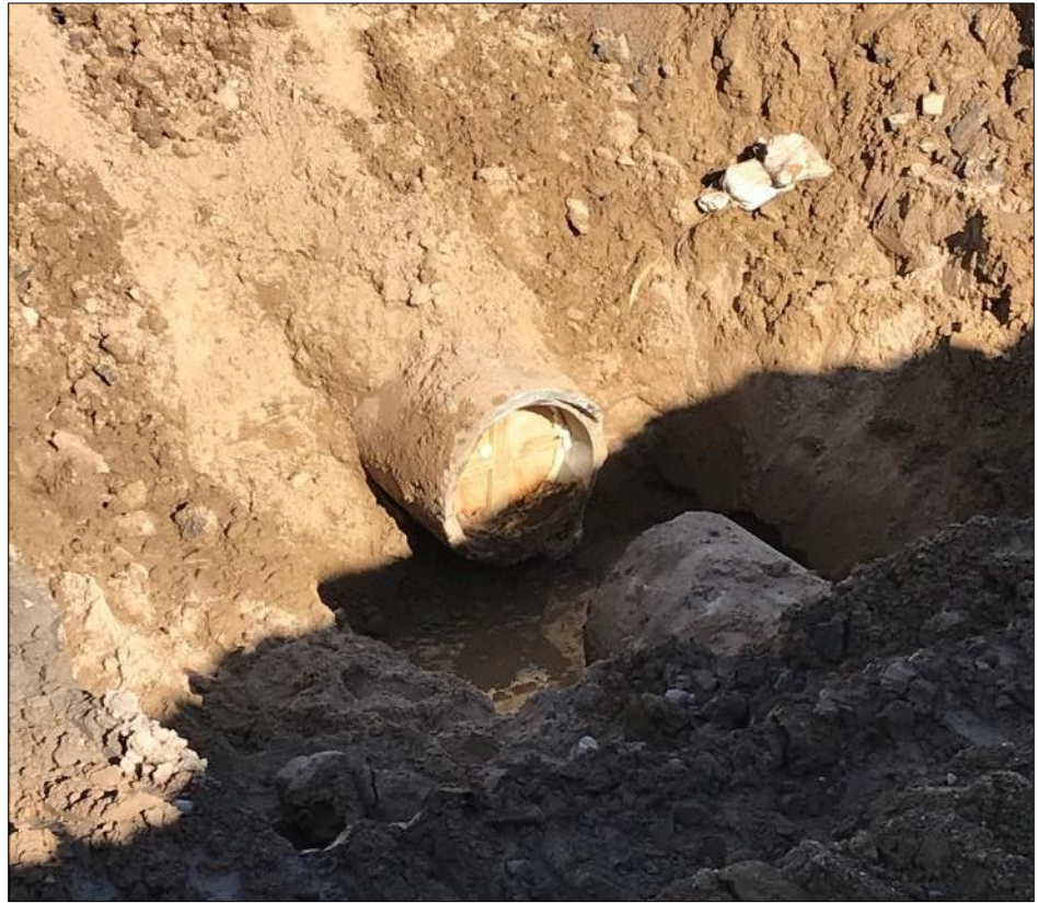
18: Sacrificial forms were installed into the ends of the exposed pipes.
