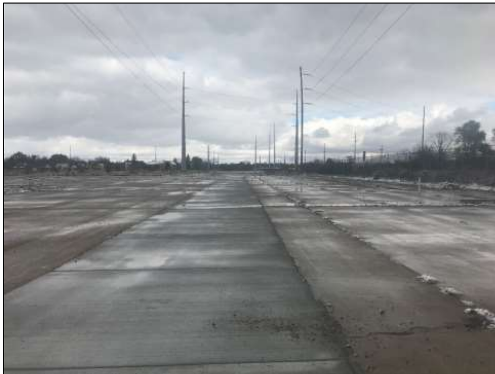
6 and 7: Water noted to run east near the western property boundary.
