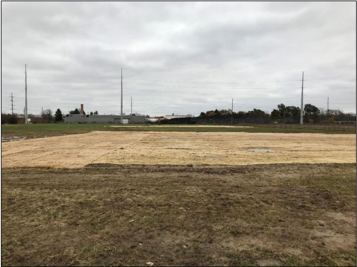
32: Excavation areas were seeded and covered with hay during restoration.
