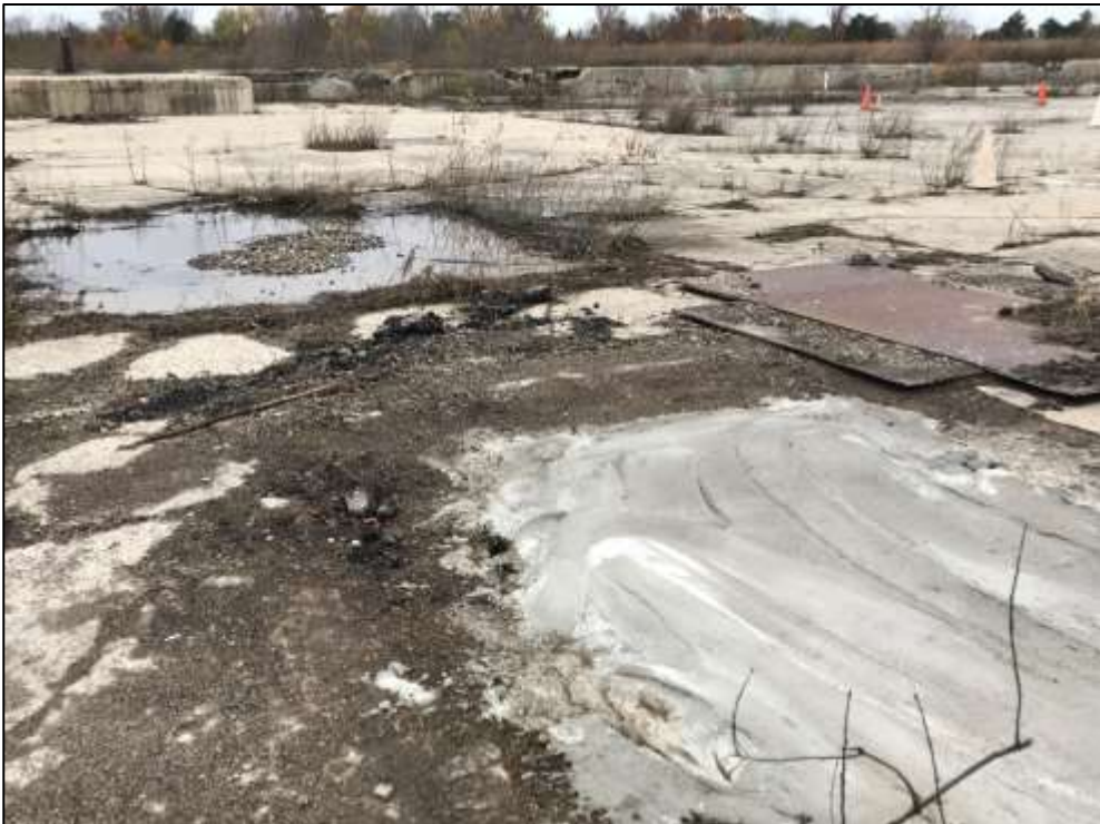
3: Oil-Water Separator (OWS) filled with CLSM. Pictured November 7, 2018
