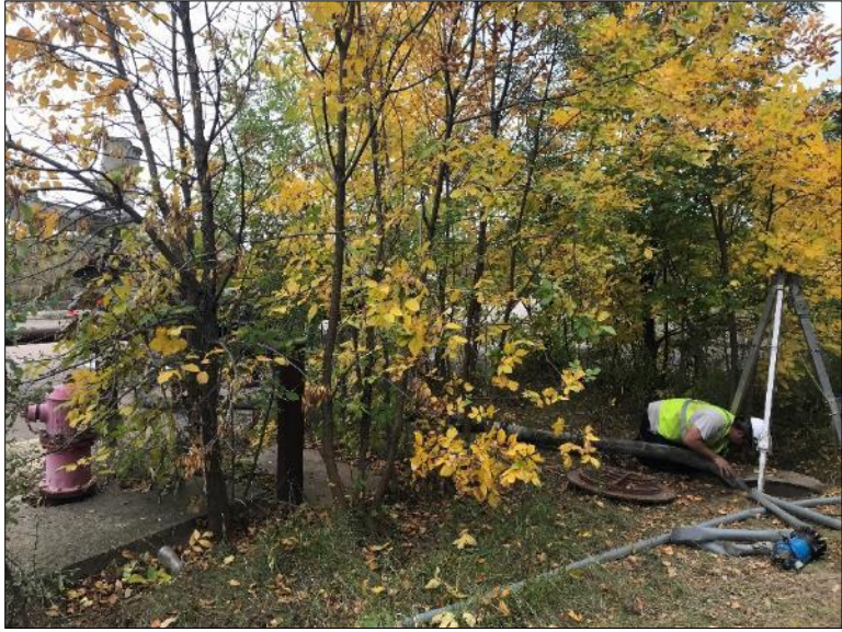
6: The crew directs concrete into the bulkhead form in manhole P3-MH-1-7
