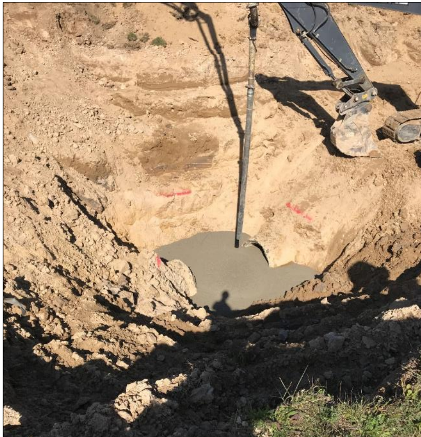
20: Western CLSM monolith after pouring was complete
