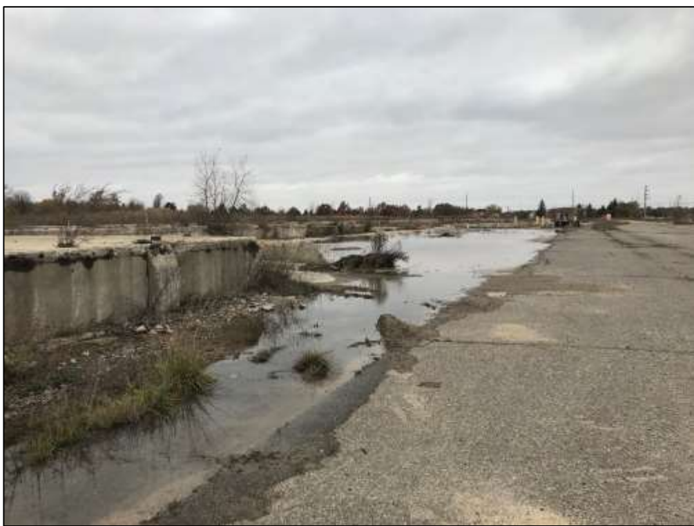
3: Oil-Water Separator (OWS) filled with CLSM. Pictured November 7, 2018
