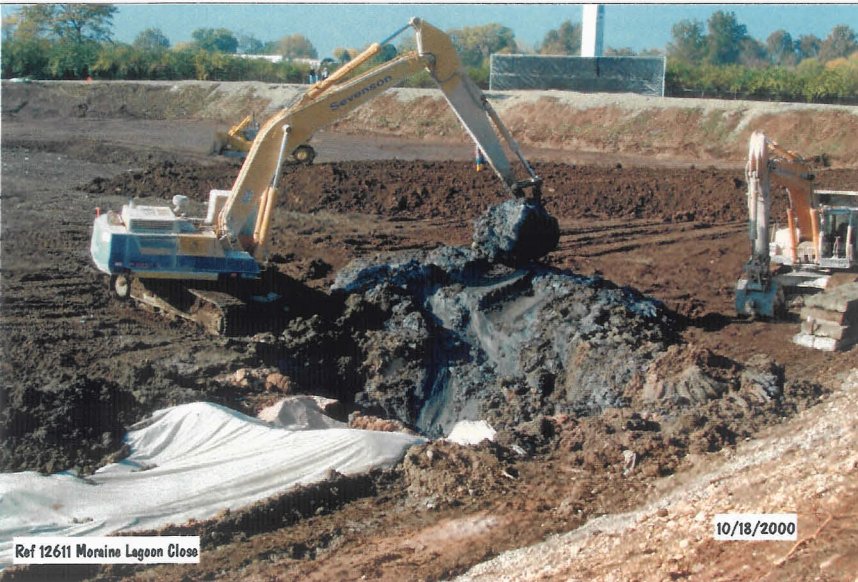
Photograph No. 21 Solidifying Sludge - South Lagoon - Secondary Basin
