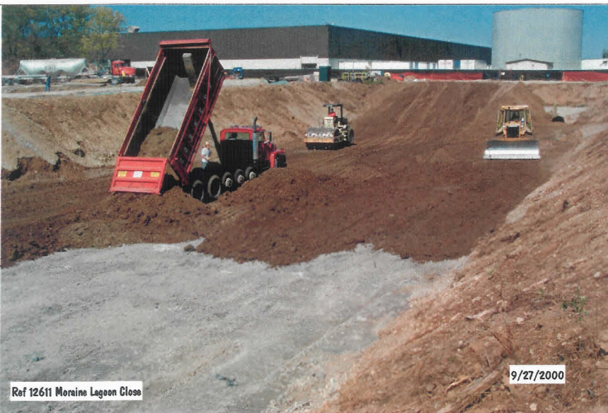
Photograph No. 18 Solidifying Sludge - South Lagoon - Primary Basin
