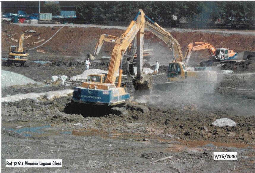
Photograph No. 16 Solidifying Sludge - South Lagoon - Secondary Basin
