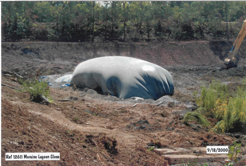
Photograph No. 13 Solidifying Sludge - South Lagoon - Secondary Basin Unloading CKD into visqueen pocket. Looking at southeast corner from east bank.
