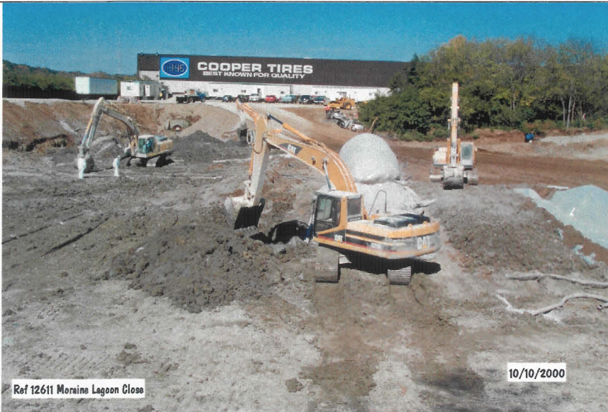
Photograph No. 20 Solidifying Sludge - South Lagoon - Secondary Basin
