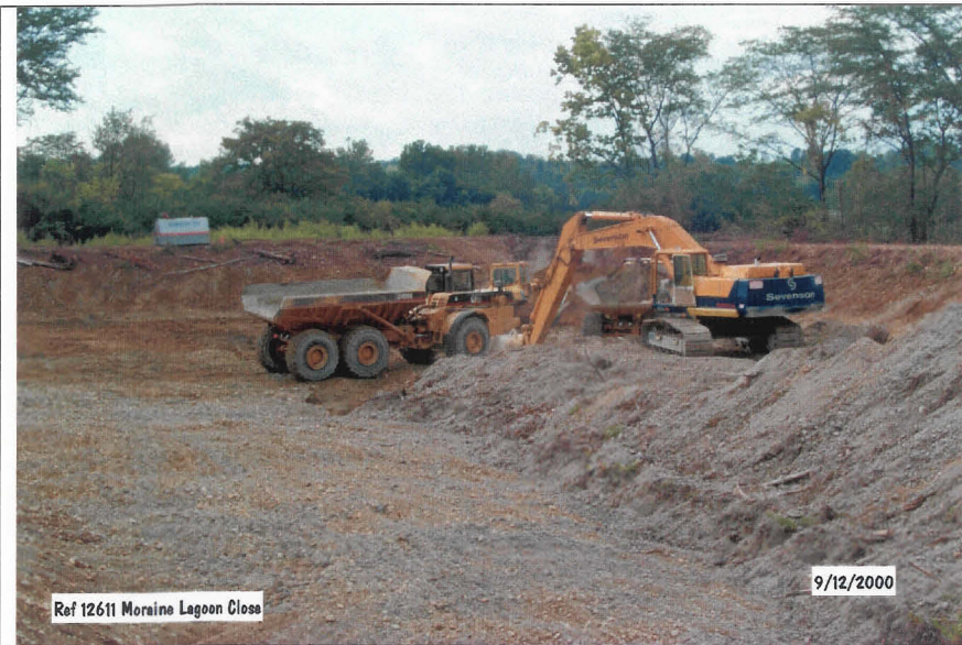
Photograph No. 7 Sludge Transfer - South Lagoon - Sludge Drying Basin
