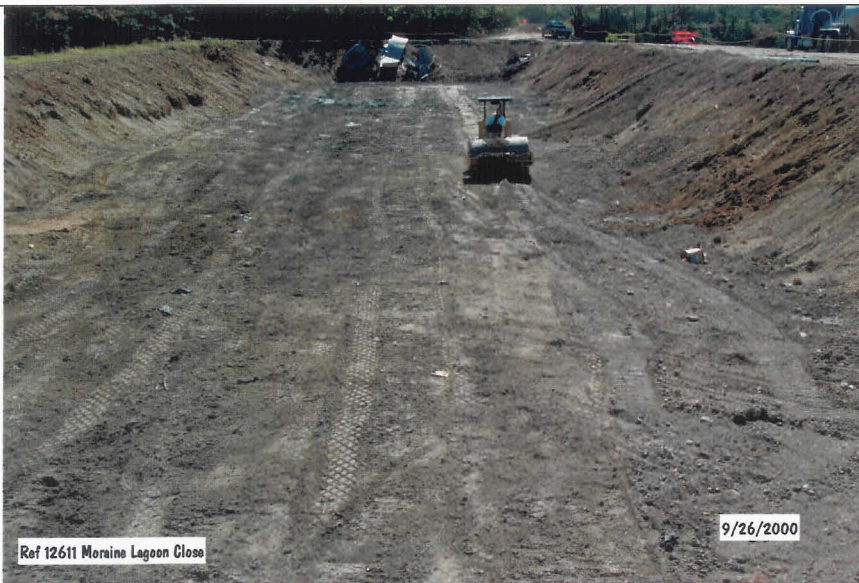
Photograph No. 17 Solidifying Sludge - South Lagoon - Primary Basin
