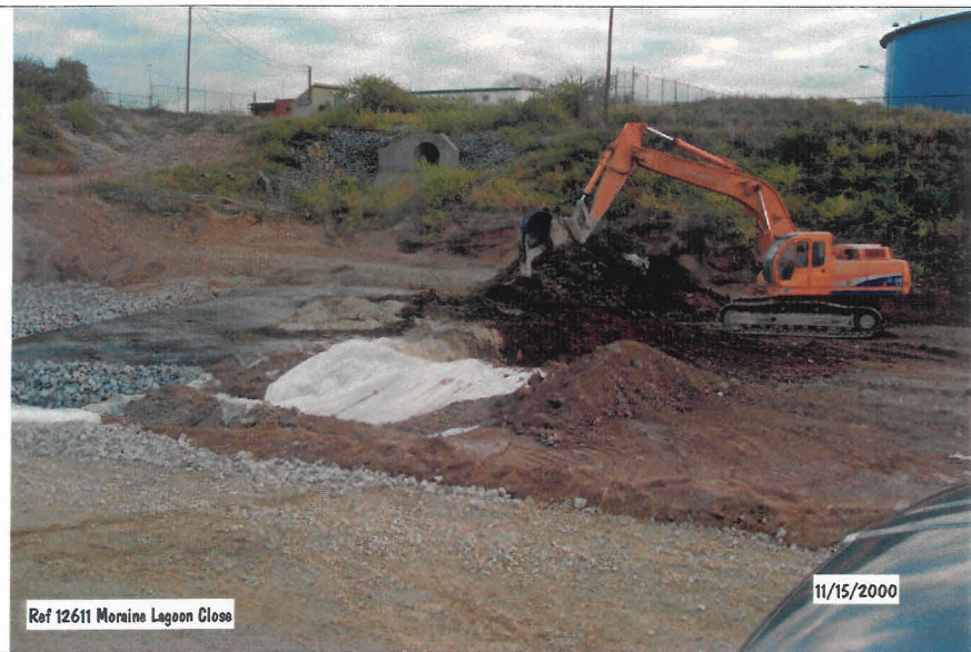
Photograph No. 33 Solidifying Sludge - North Lagoon – Secondary Basin
