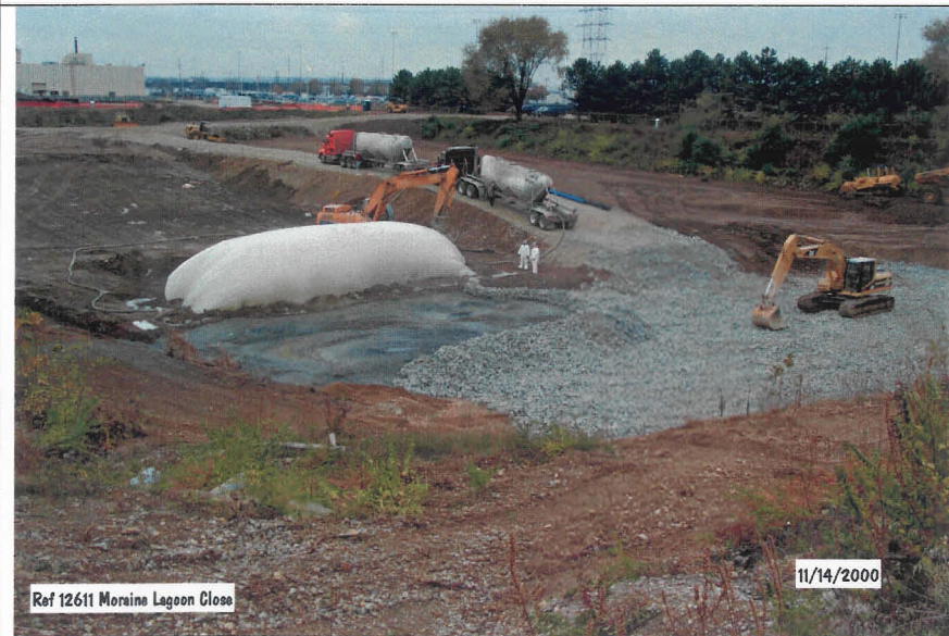
Photograph No. 32 Solidifying Sludge - North Lagoon – Secondary Basin
