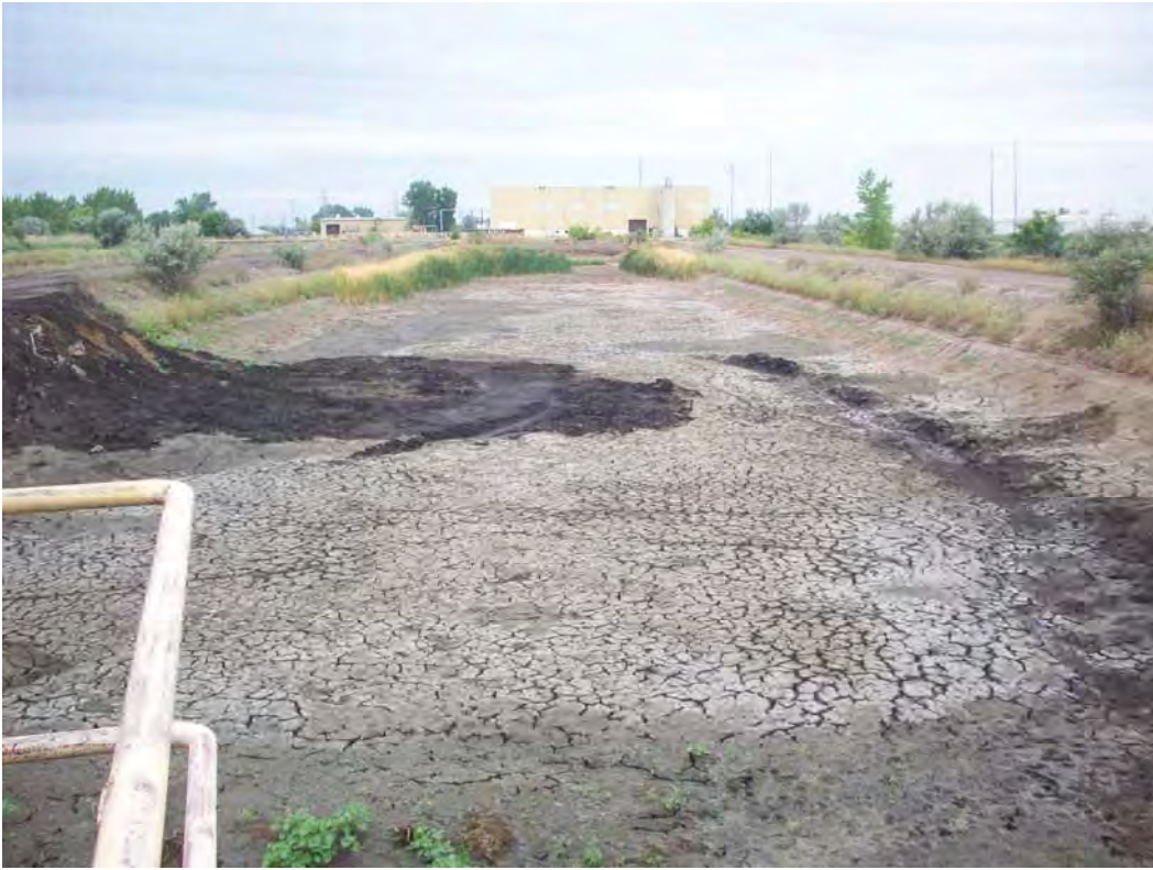
PHOTO 1: PRIMARY SETTLING BASIN 3 - LOOKING SOUTHWEST (7/18/2012)
