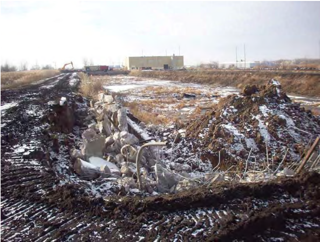
PHOTO 6: PRIMARY SETTLING BASIN 4 - LOOKING SOUTHWEST (12/12/2012)
