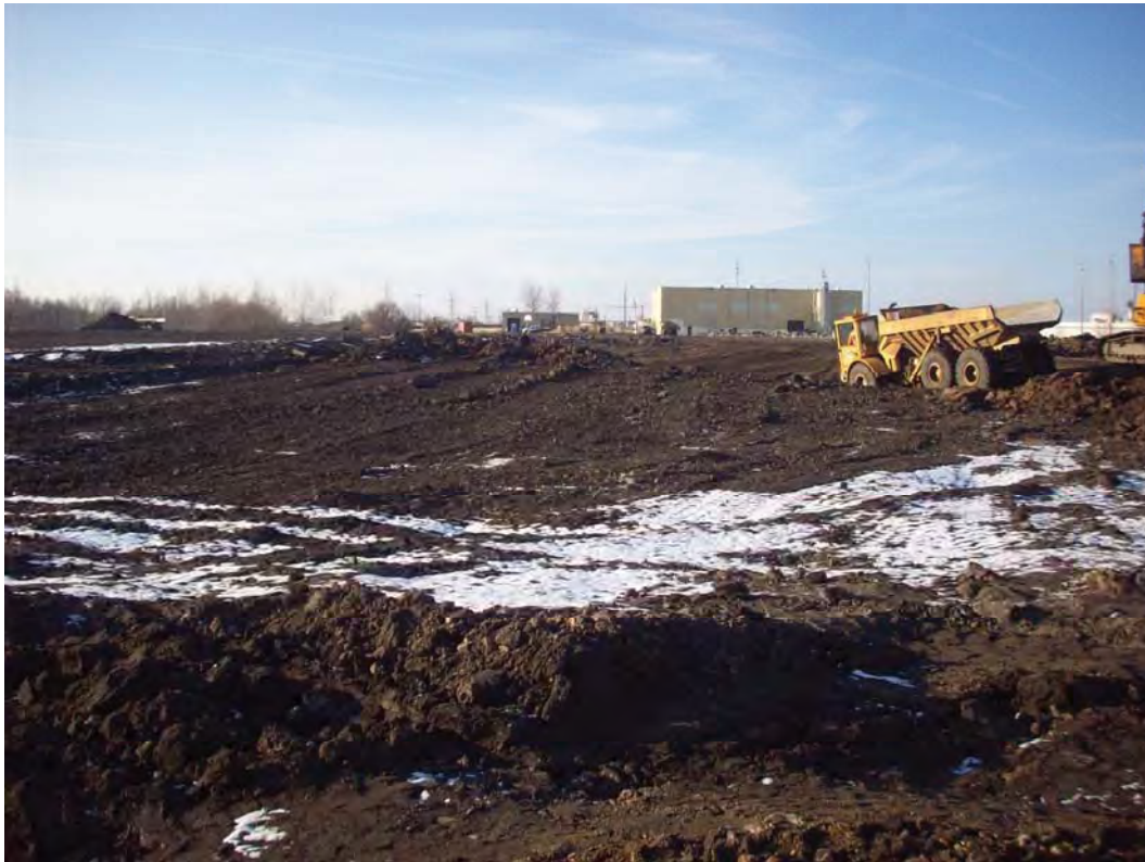
PHOTO 8: PRIMARY SETTLING BASIN 4 - LOOKING SOUTHWEST (01/07/2013)
