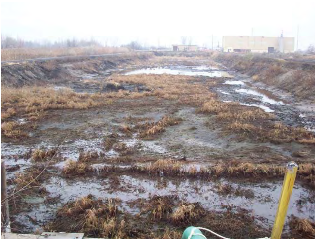
PHOTO 4: PRIMARY SETTLING BASIN 4 - LOOKING SOUTHWEST (12/4/2012)
