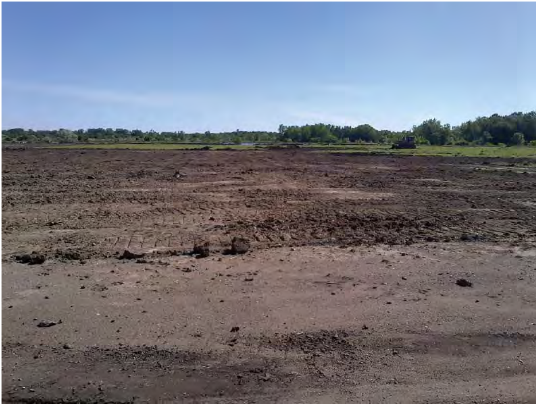
PHOTO 10: PRIMARY SETTLING BASINS – TOPSOIL (06/03/2013)
