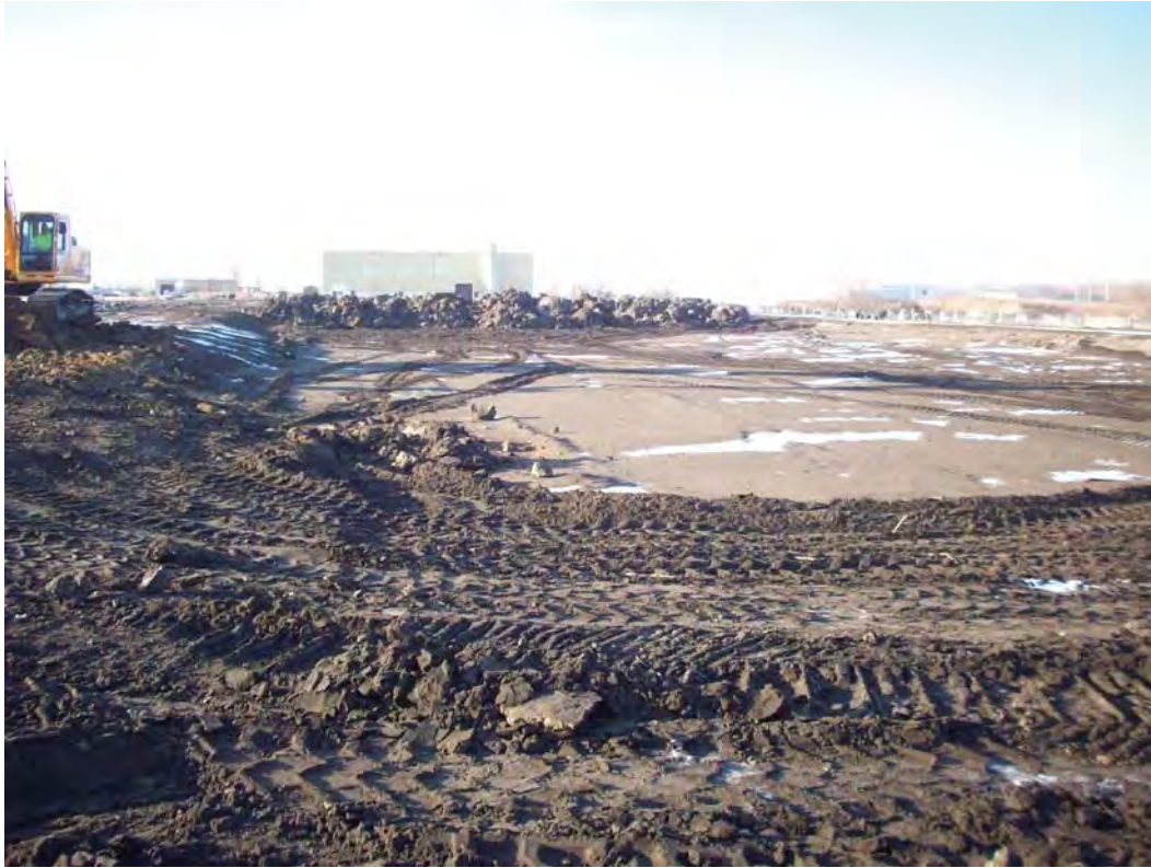
PHOTO 7: PRIMARY SETTLING BASIN 3 - LOOKING SOUTHWEST (01/07/2013)
