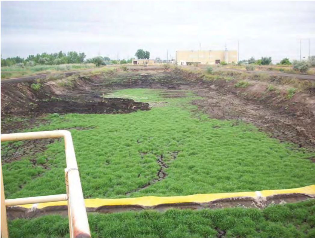
PHOTO 2: PRIMARY SETTLING BASIN 4 - LOOKING SOUTHWEST (07/18/2012)
