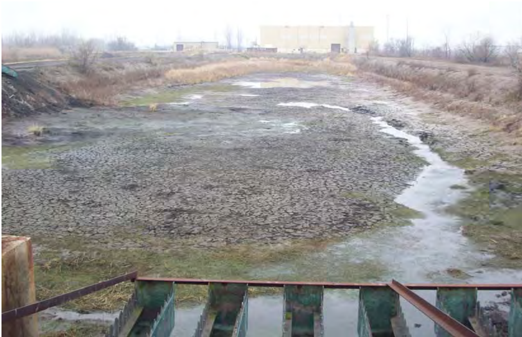
PHOTO 3: PRIMARY SETTLING BASIN 3 - LOOKING SOUTHWEST (12/4/2012)
