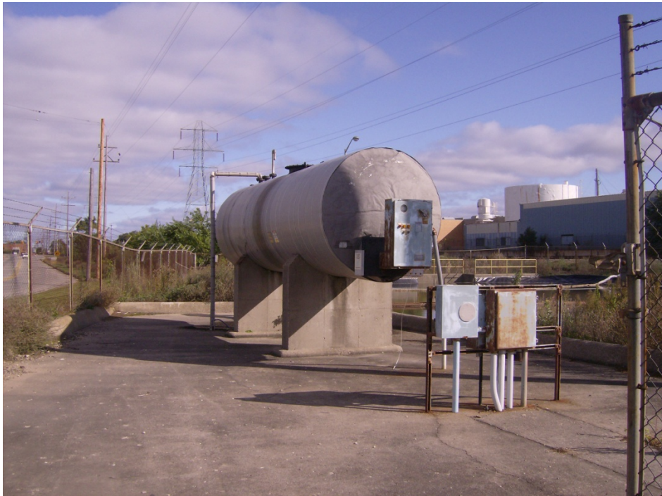
Photo 1 – View of former skimmed oil AST on concrete pad
