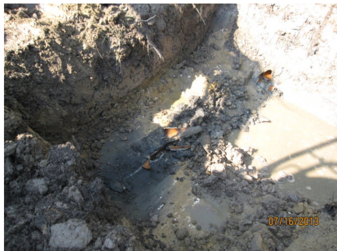
View of drain tile section uncovered.
