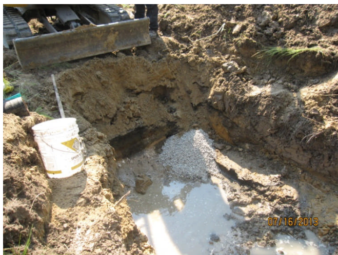
View of bentonite placed on east end pipe.
