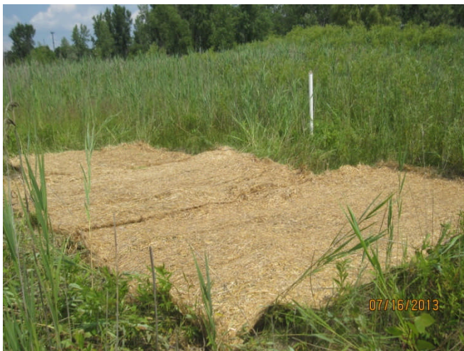
Straw matting placed at test excavation area.
