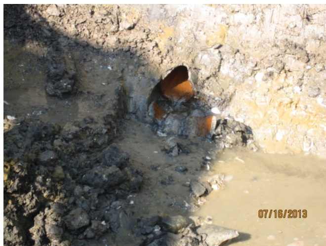
View of west end of pipe opening adjacent to fence.
