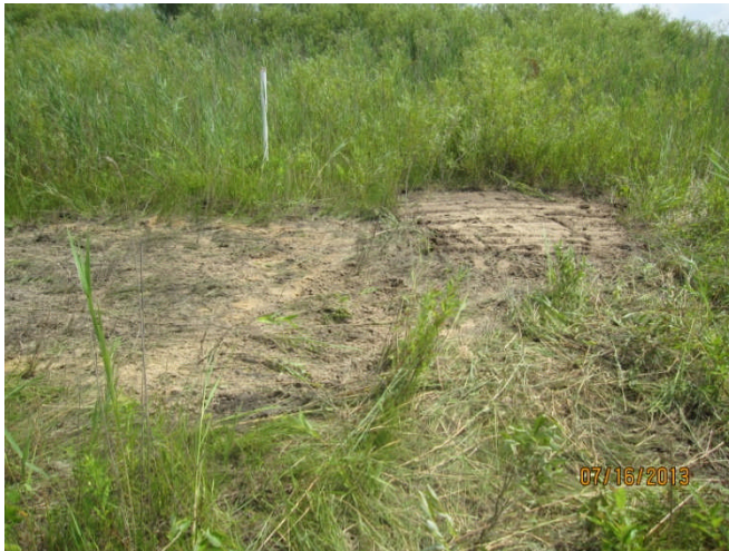
Topsoil and seed placed at test excavation area.
