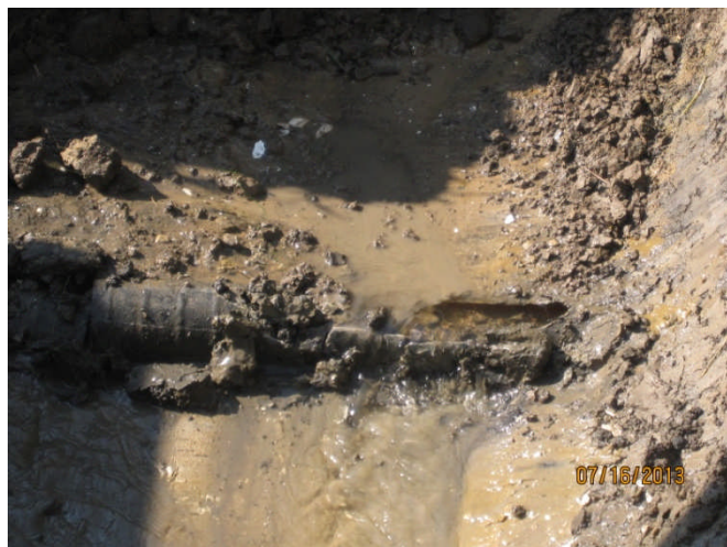
View of drain tile at west end adjacent to fence line.
