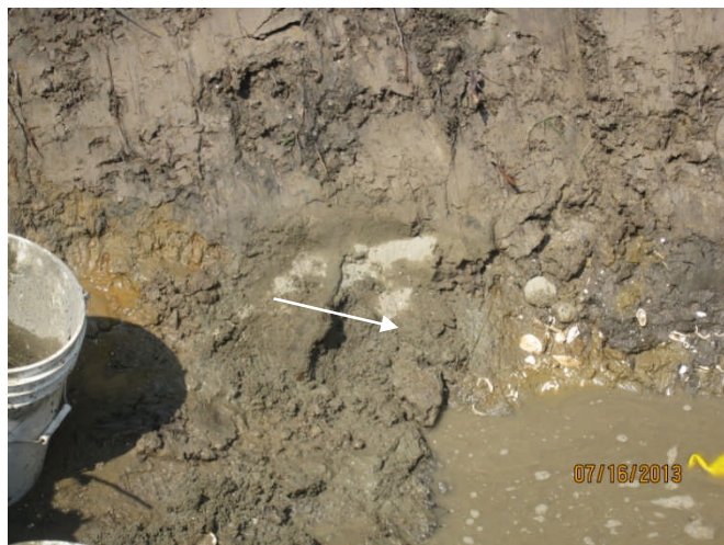
Hydraulic cement placed over opening at west end (see arrow).
