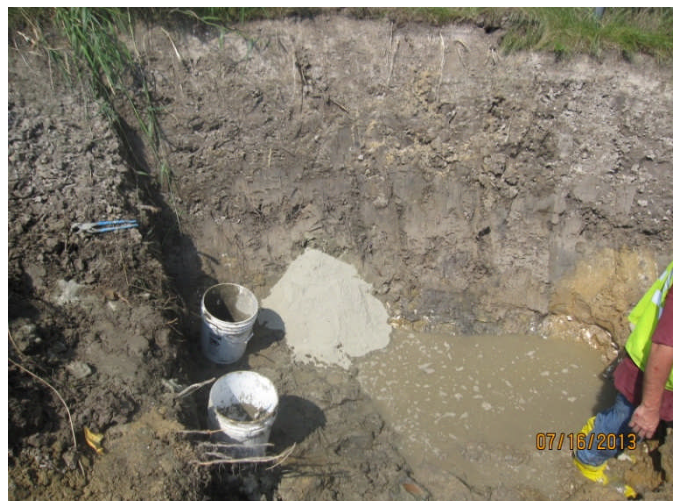
Quick-crete placed over opening at west end.
