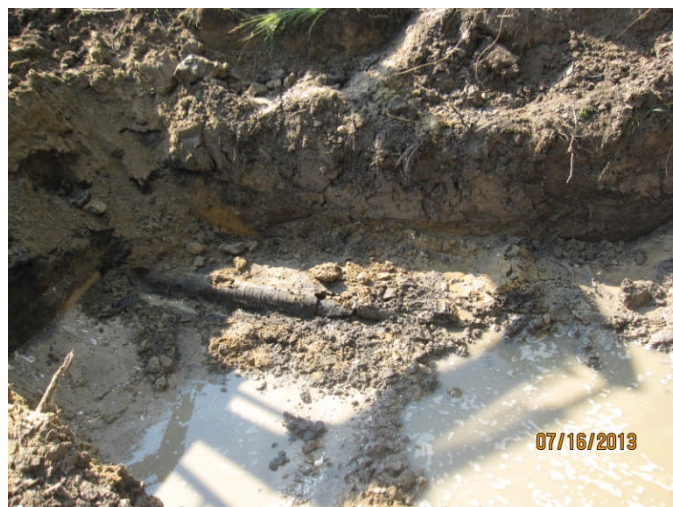
View of tile sections uncovered at east end.
