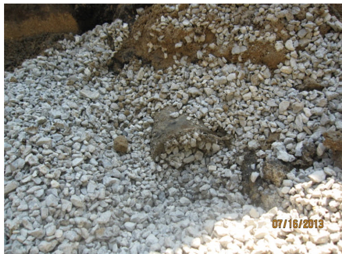
Hydraulic cement and bentonite placed at east end of pipe.
