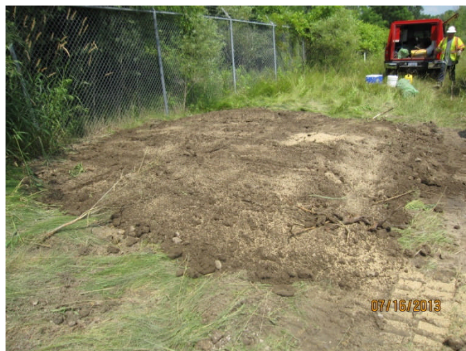
Topsoil and seed placed at excavation by fence line.
