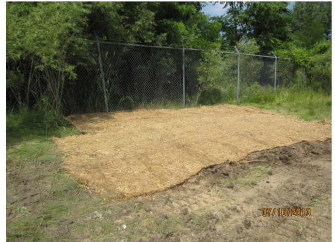
Straw matting placed at excavation by fence line.
