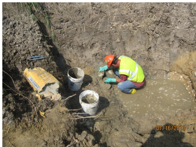
YECI placing clay pieces inside of west end pipe opening to stop water flow.
