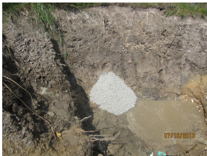
View of bentonite placed over opening at west end.
