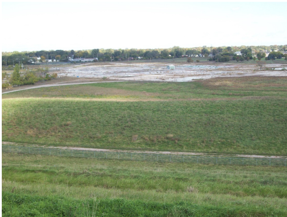
Photo 1 – Concrete Floor Slab From Green Point Landfill (9/20/12)
