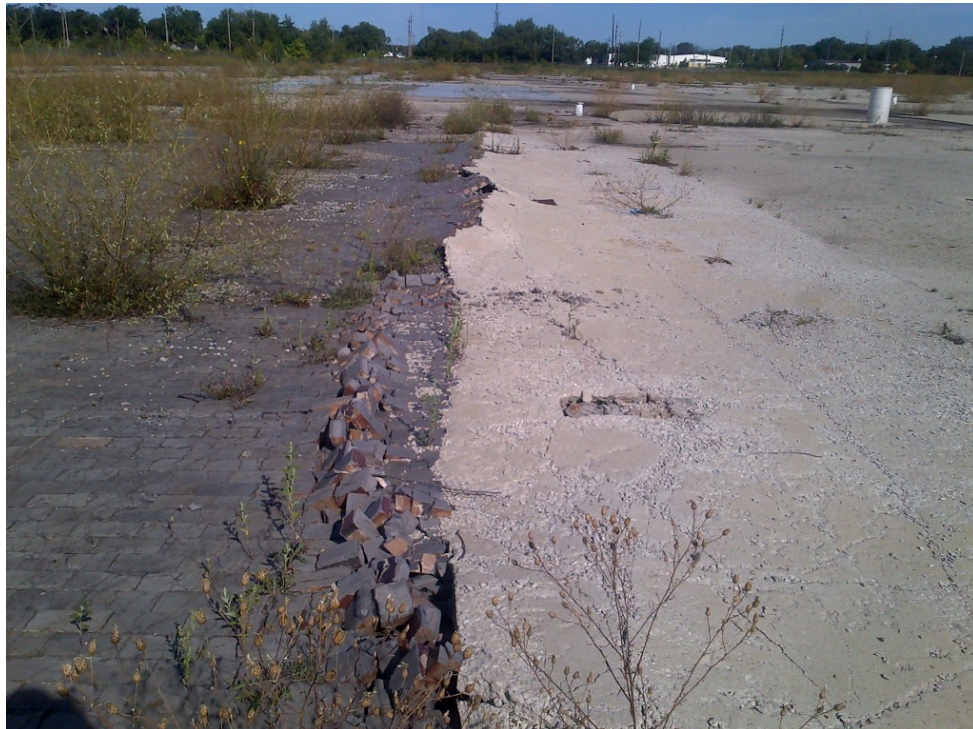
Photo 4 – Concrete Floor Slab and Brick flooring (8/15/2014)
