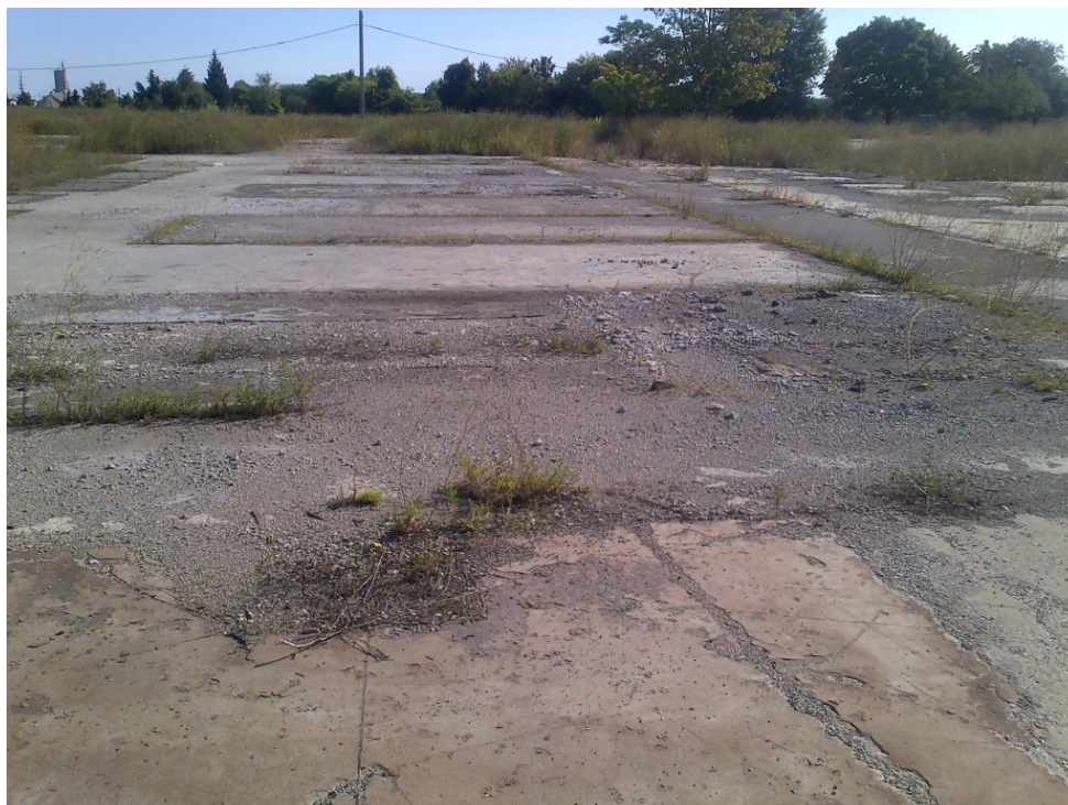
Photo 2 – Concrete Floor Slab (8/15/2014)
