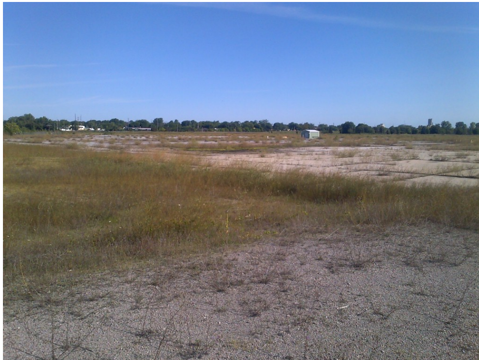
Photo 3 – Concrete Floor Slab (8/15/2014)
