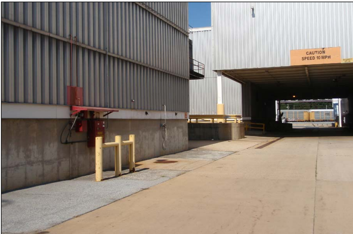
PHOTO 6: Tank truck loading area for waste solvent tanks
