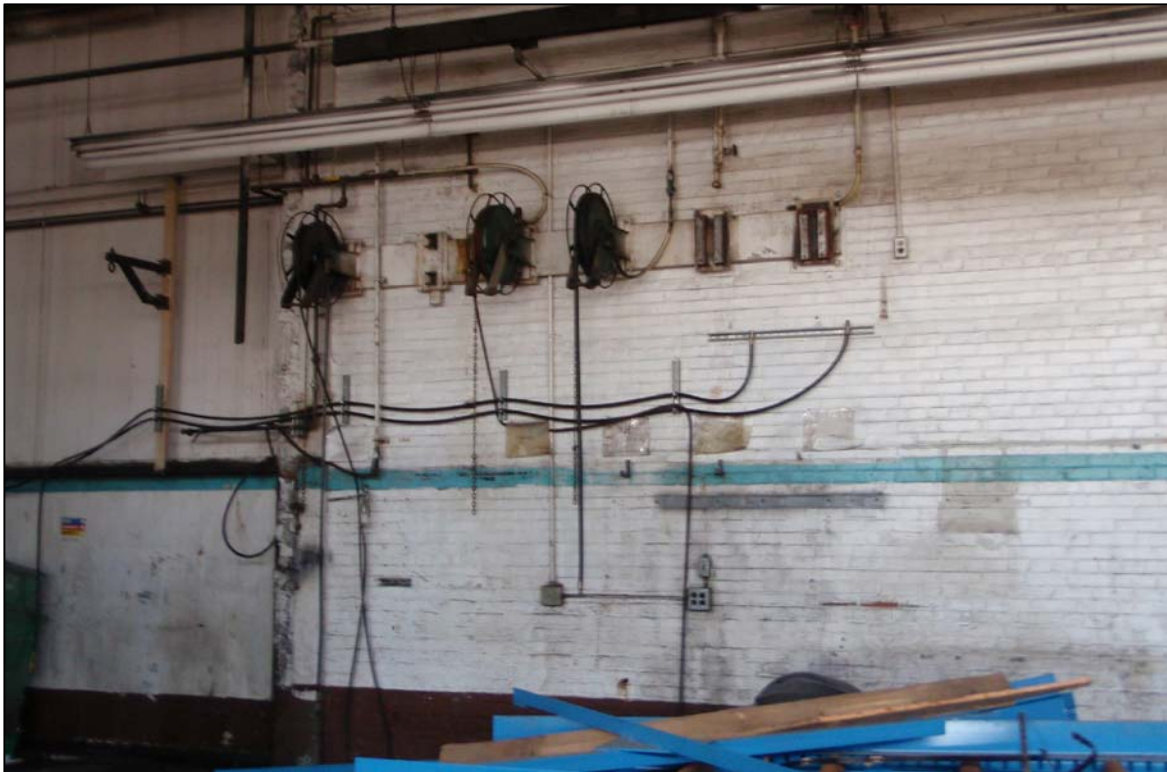
PHOTO 23: Petroleum Dispensing Area - Anchor Building
