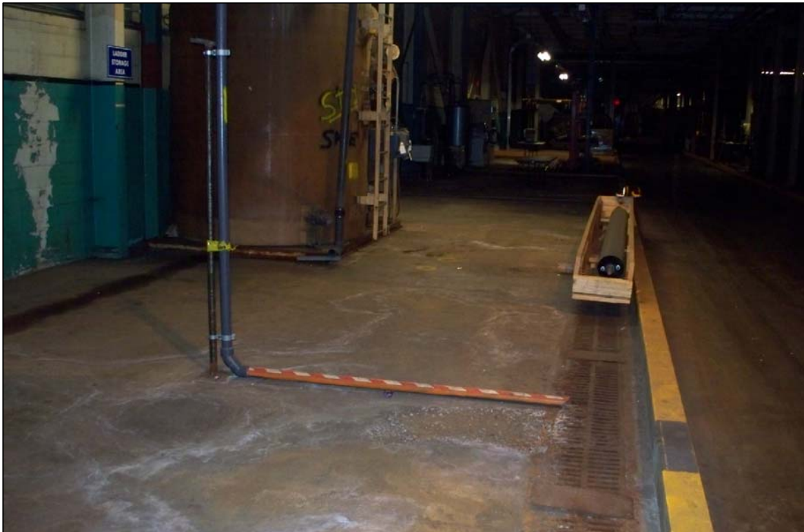
PHOTO 13: DI water system area
