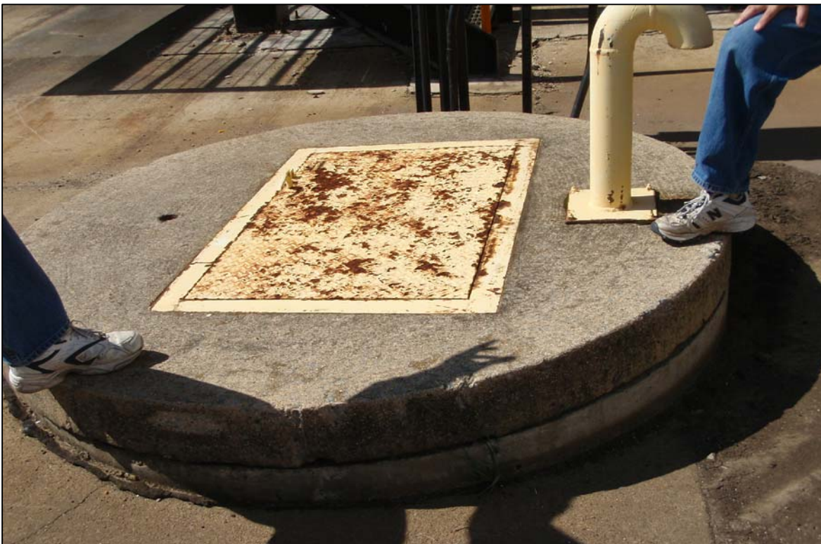
PHOTO 24: Groundwater sump east of Modular Paint Building
