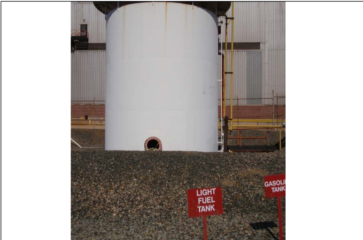
PHOTO 2: AST "B" - Facing north
