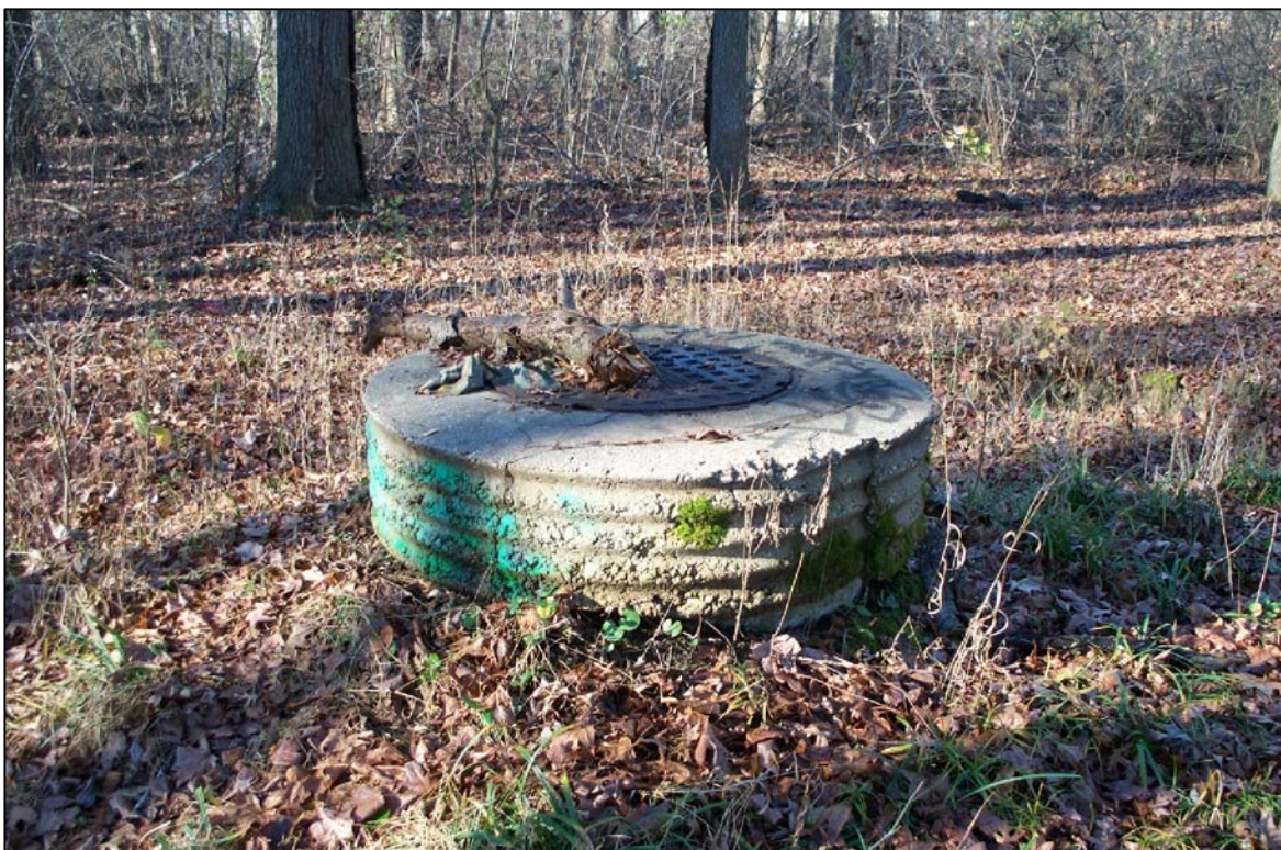
PHOTO 27: Sanitary sewer manhole in wooded area
