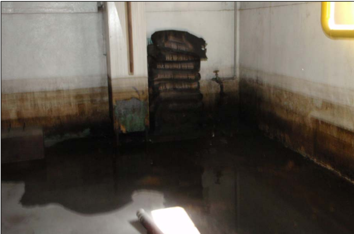
PHOTO 16: Power House basement
