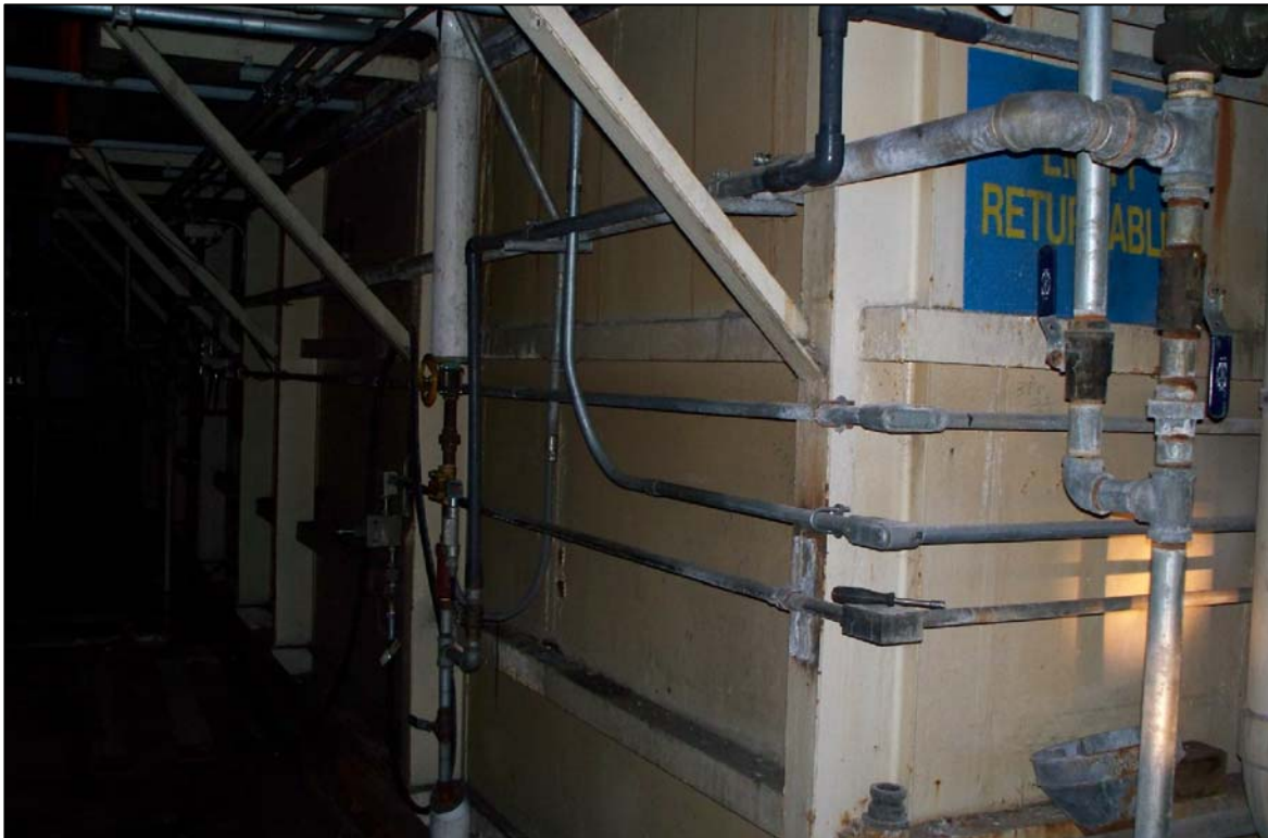
PHOTO 21: Sludge tank near Grit Separator Building
