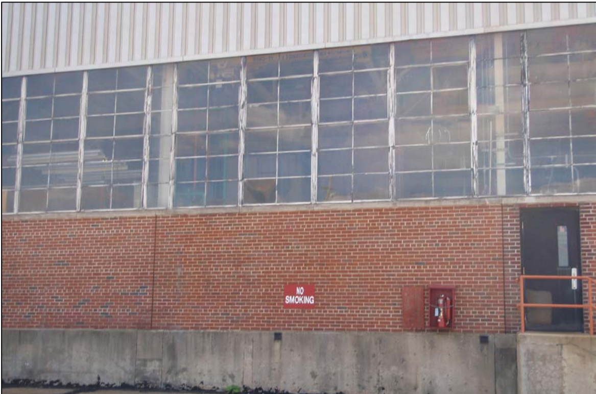
PHOTO 20: Former hazardous waste storage area
