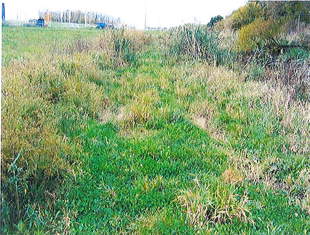
Photograph 3: Vegetation in access road between CB-5 and CB-4 near turnaround area.
