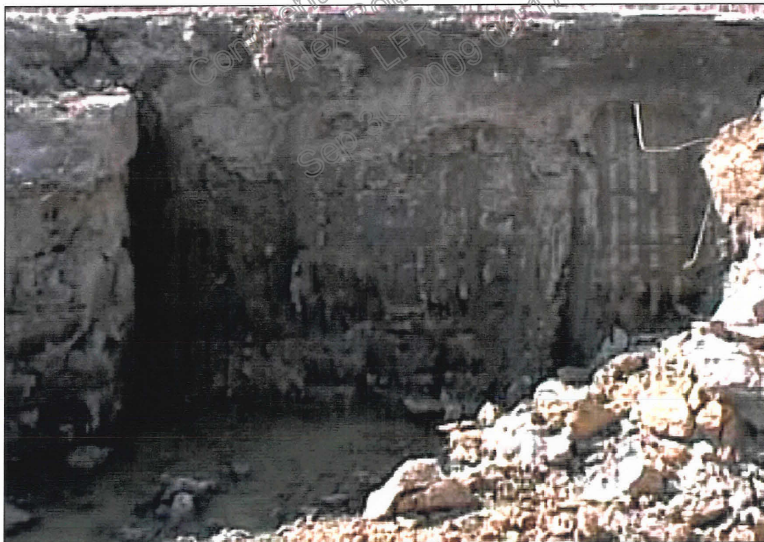
SOUTH WALL - DSA EXCAVATION
