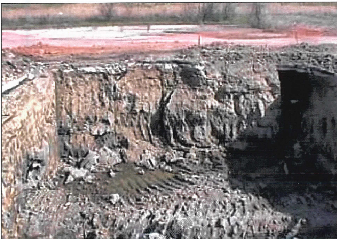
NORTH WALL - DSA EXCAVATION
