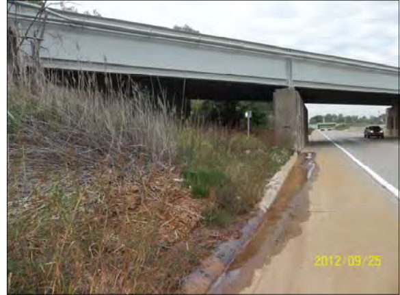
Ueepagg"qdugt xgf "along Michii cp"Cxg0 Photo direction southwest.
