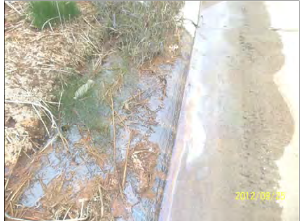
Uggr ci g"qdugt xgf "cnp i "O lej ki cp"Cxg0 Photo direction southwest.
