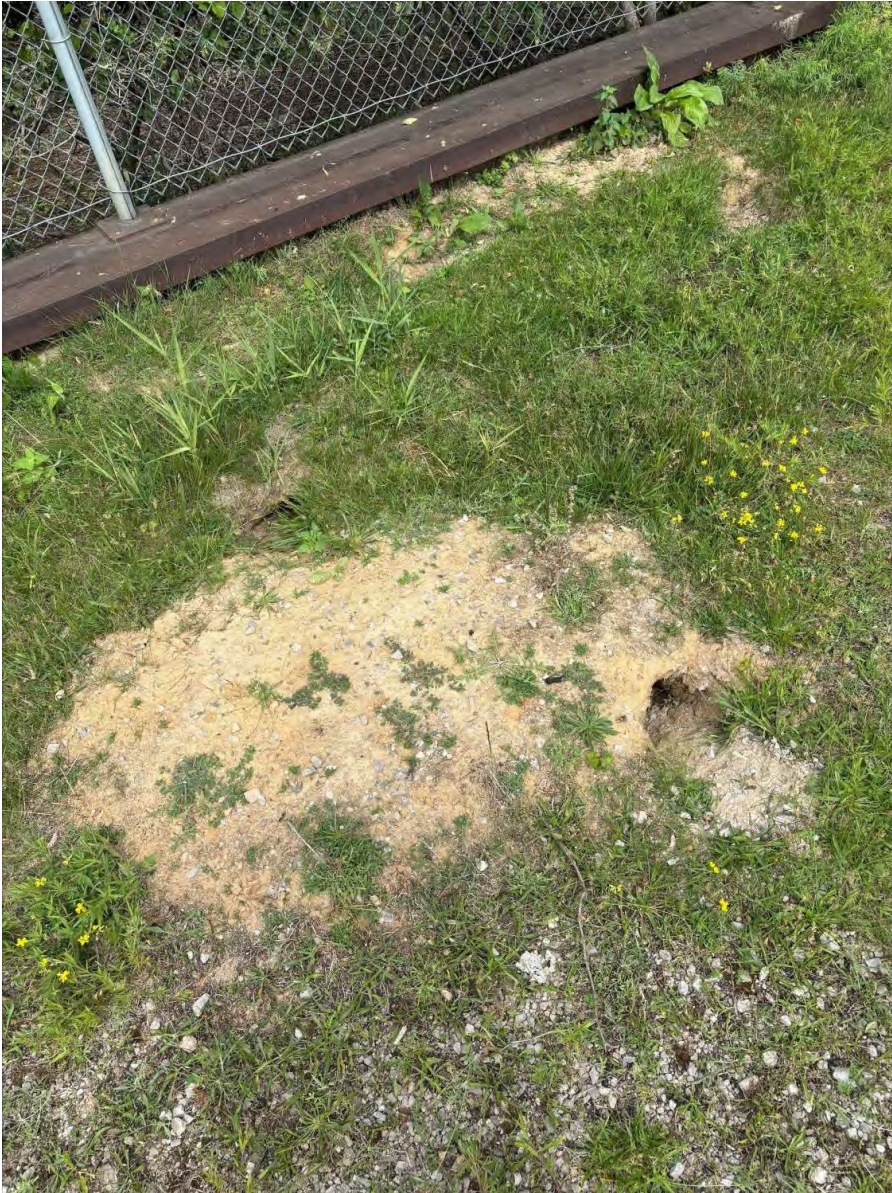
4. Left: Groundhog burrow near outfall on cap (EGLE, July 11). Right: Same burrow marked and staked (GHD, Oct 4), to be filled following animal removal.
