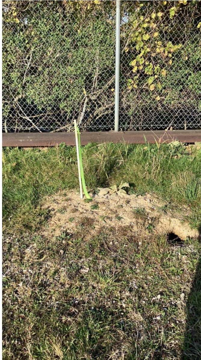
4. Left: Groundhog burrow near outfall on cap (EGLE, July 11). Right: Same burrow marked and staked (GHD, Oct 4), to be filled following animal removal.
