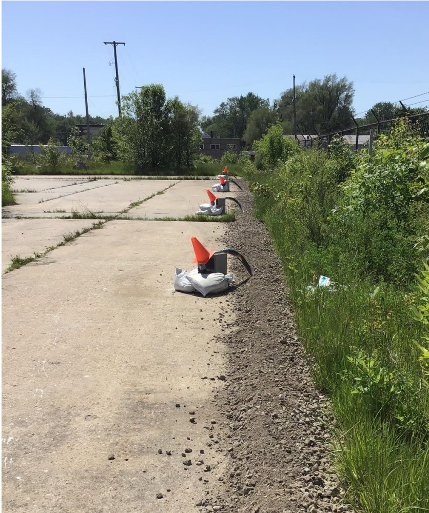
Biosparge transect with hoses covered in gravel
