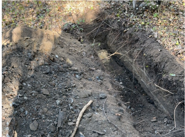
TP-137_0-4_11072024 Debris present
