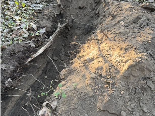
TP-124_0-3_11072024 No debris present
