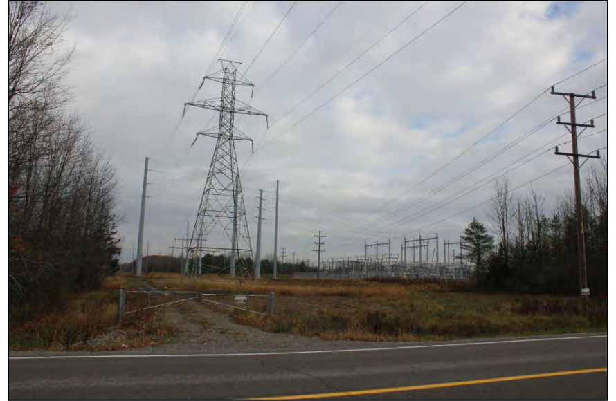
Photo 38: Power substation looking northeast from E Stanley Road. Built c.1955.
