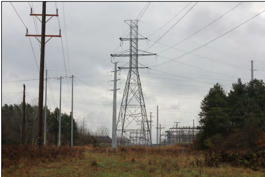
Photo 27: Looking east toward power substation from clearing between project areas.
