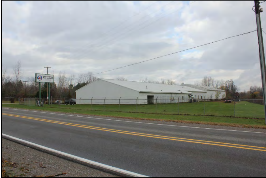
Photo 41: 1217 E Stanley Road looking northwest. Built c.1990.
