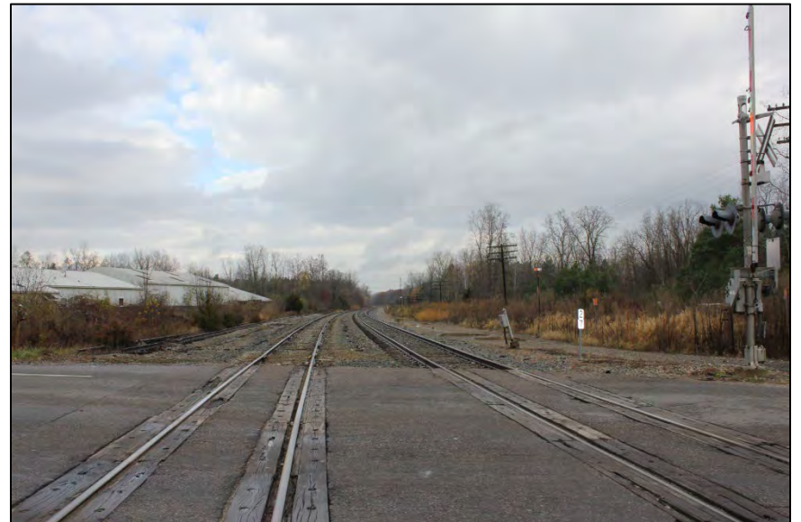
Photo 40: Looking north up railroad tracks along western edge of project area.
