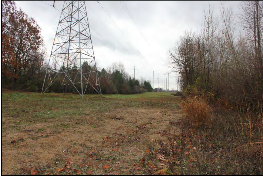
Photo 21: Looking south down power line clearing from east edge of Project Area 1.
