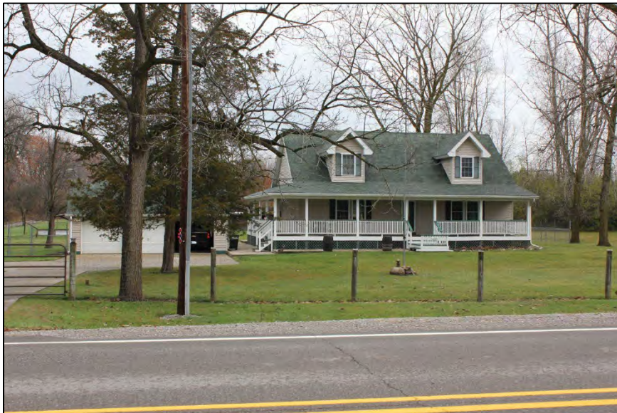
Photo 39: 1297 E Stanley Road looking northeast. Built c.1930.
