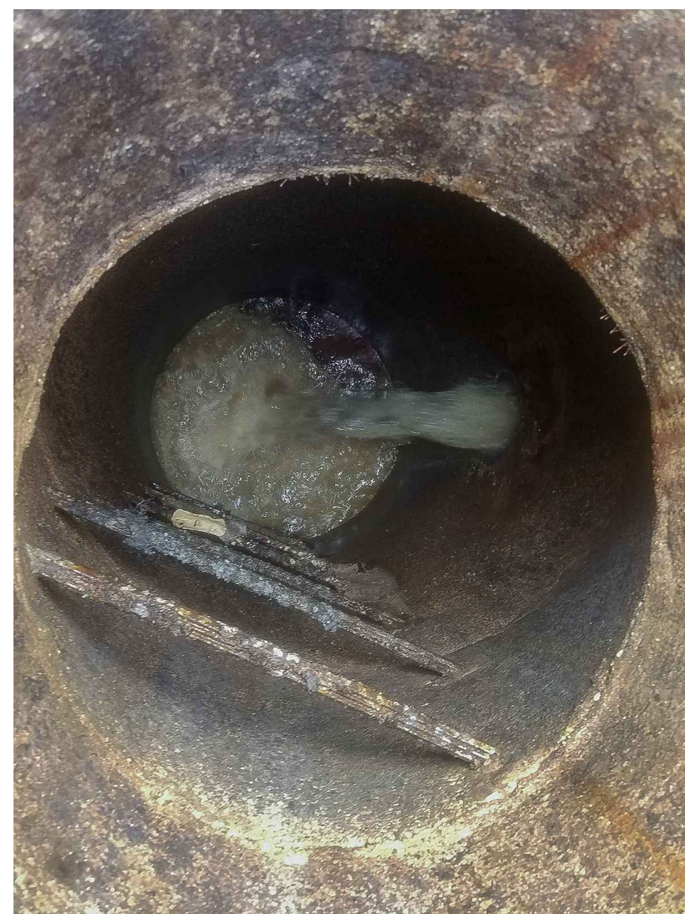
IMAGE OF INSIDE MANHOLE 5G0047
