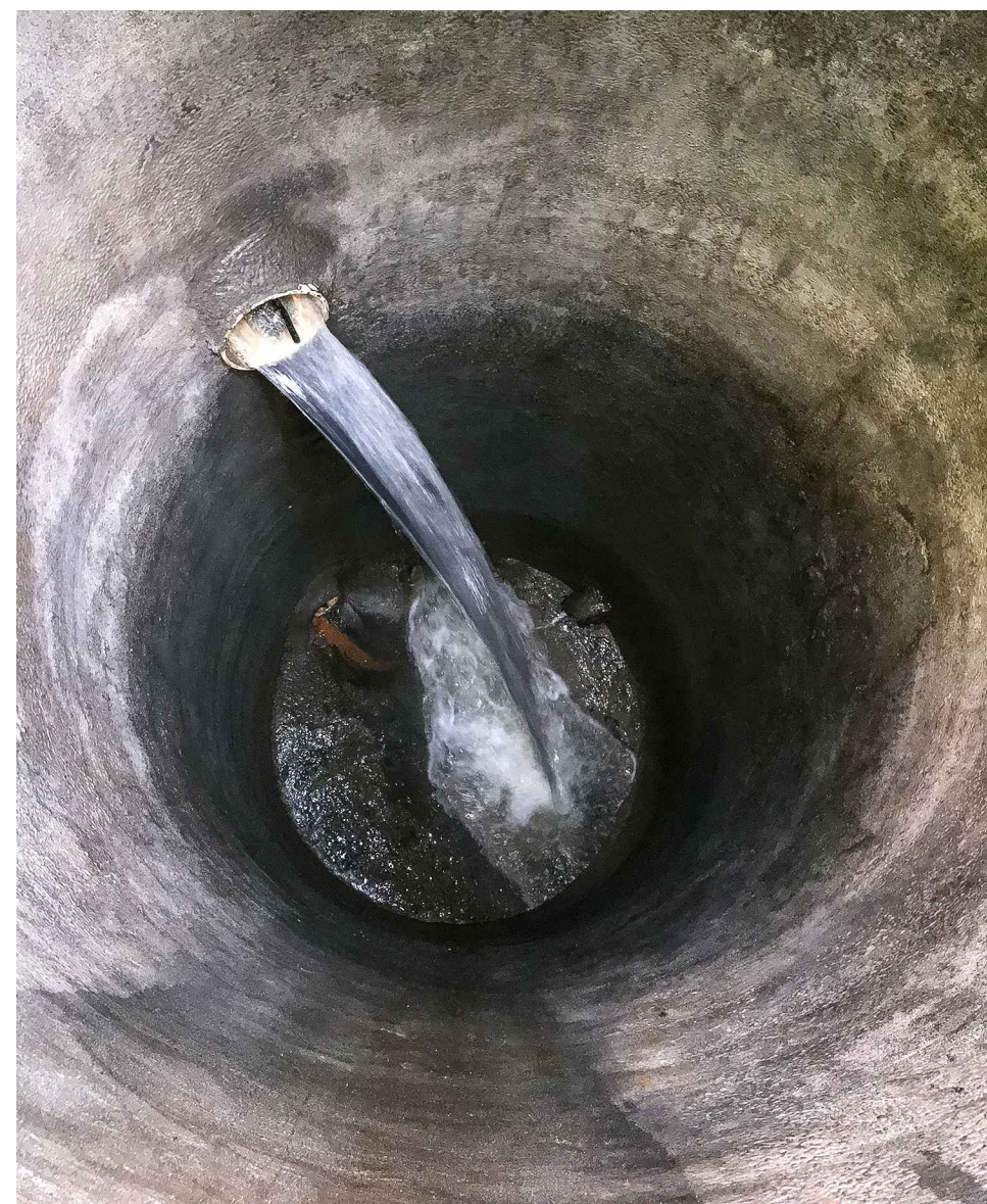
IMAGE OF INSIDE MANHOLE 5F0226
