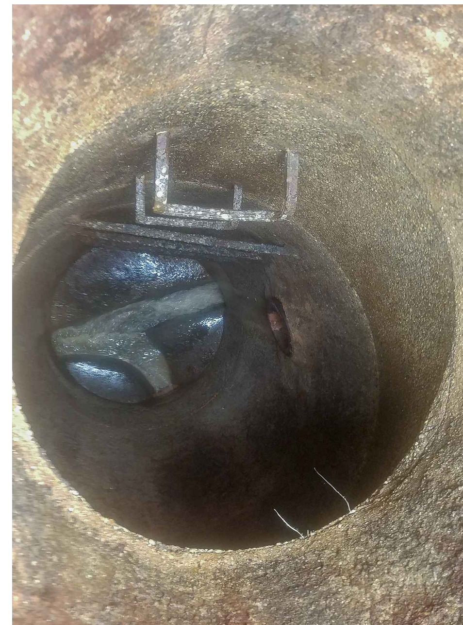
IMAGE OF INSIDE MANHOLE 5G0049
