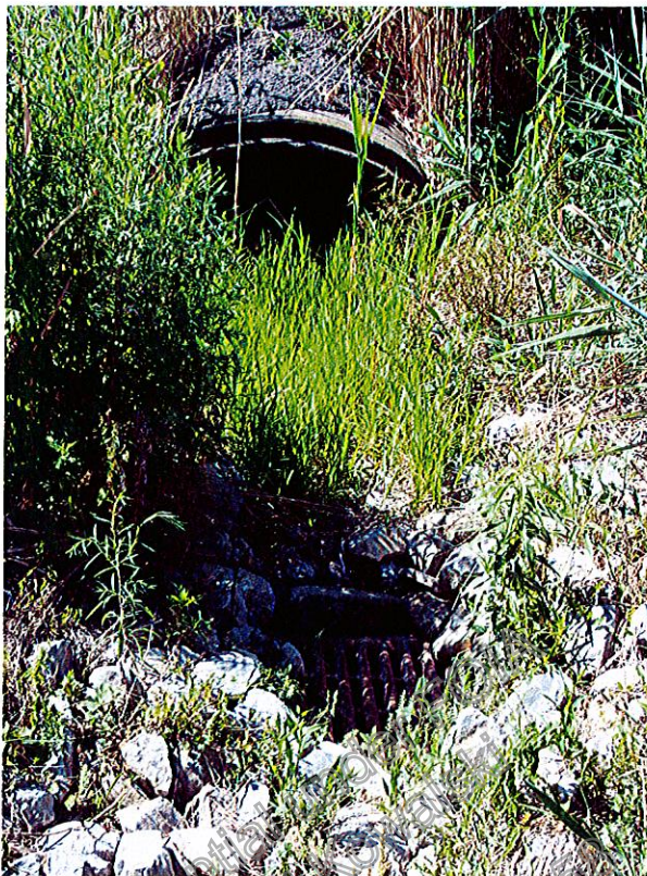
Photograph 1: View of CB-5/Outfall 004 spillway.
