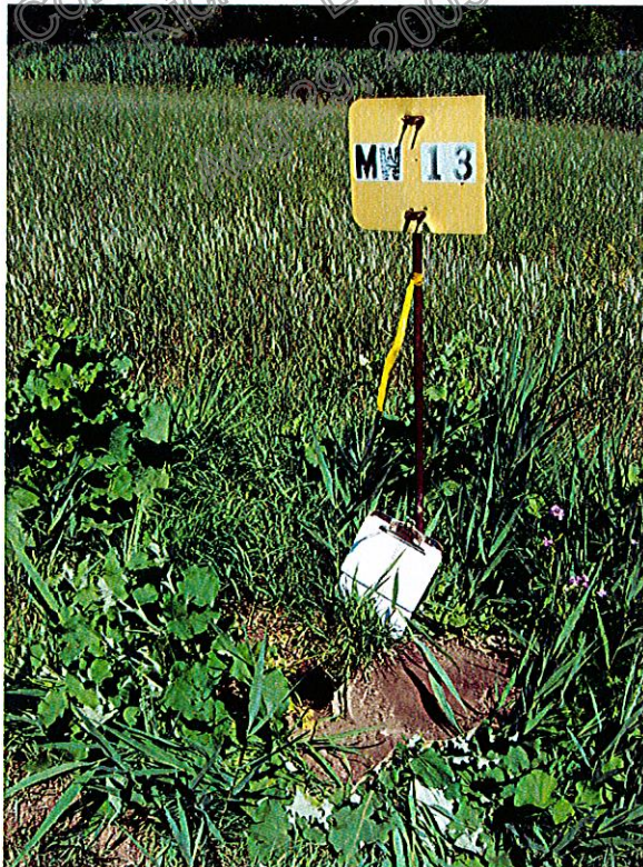
Photograph 14: View looking at burrowing animal hole at MW-13.
