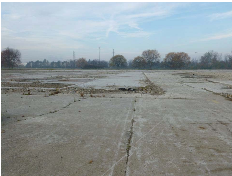
Photograph 26. Concrete footprint of former facility. Photo taken facing west from area approximately central to "D" and "E" Test Cell Wings.
