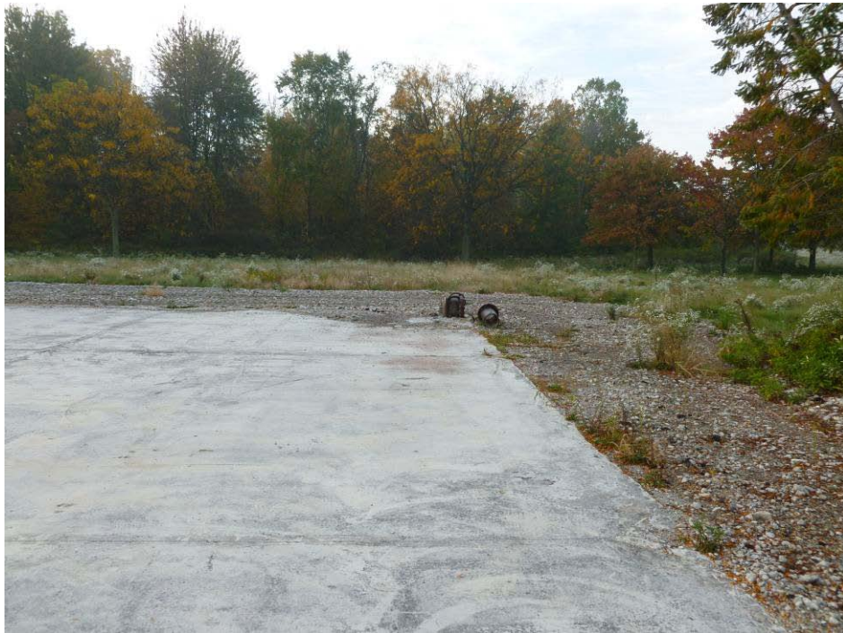
Photograph 34. Southwestern-most corner of former facility. Photo taken facing south. Objects in background believed to be components of former fire suppression system.
