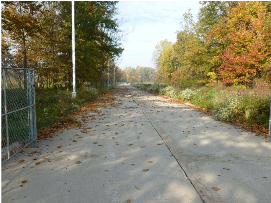
Photograph 4. Entrance to access road to Site. Photo taken facing west.
