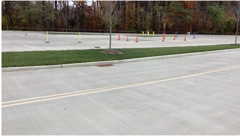
Photo 27 - View Looking East -
