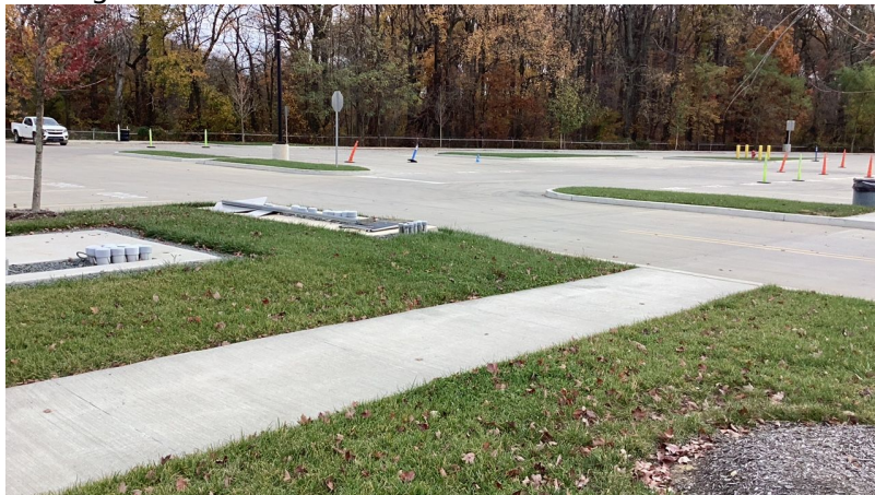
Photo 32 - View Looking East -
