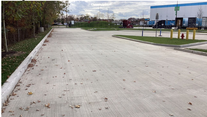
Photo 20 - View Looking East -
