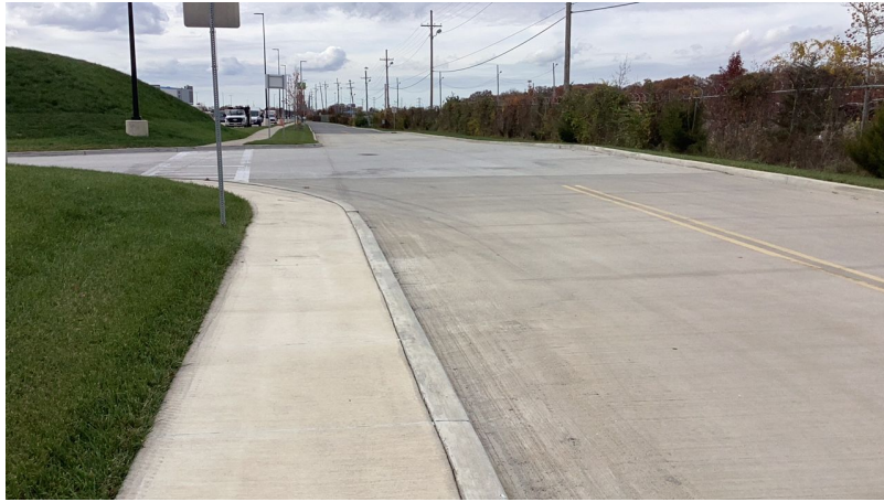
Photo 30 - View Looking East -
