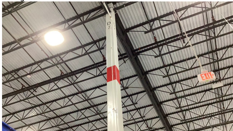
Photo 1 - View Looking East -
