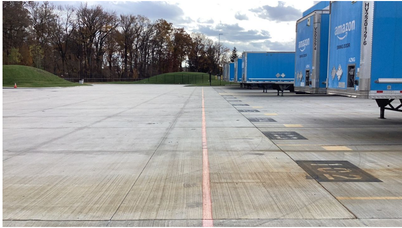
Photo 15 - View Looking East -
