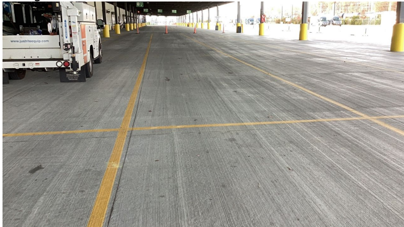
Photo 8 - View Looking East -
