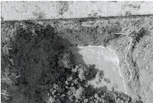
Picture 1: Water flowing out through horizontal 3/8" pilot hole for Extraction Point B.
